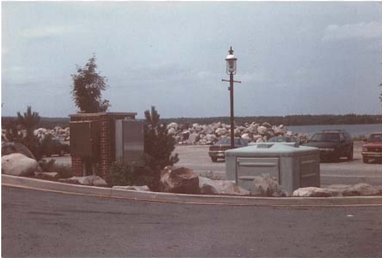
Town Of Liverpool Pumping Station
