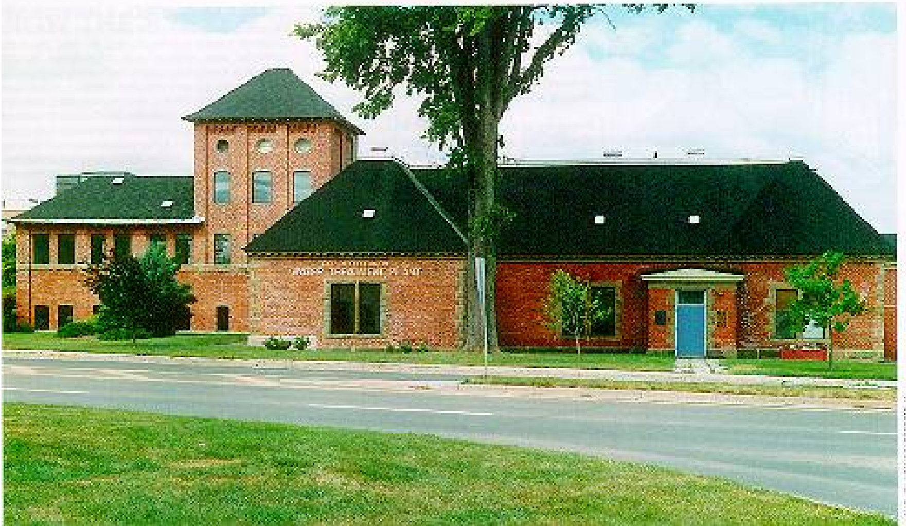
William L Barrett Water Treatment Plant
