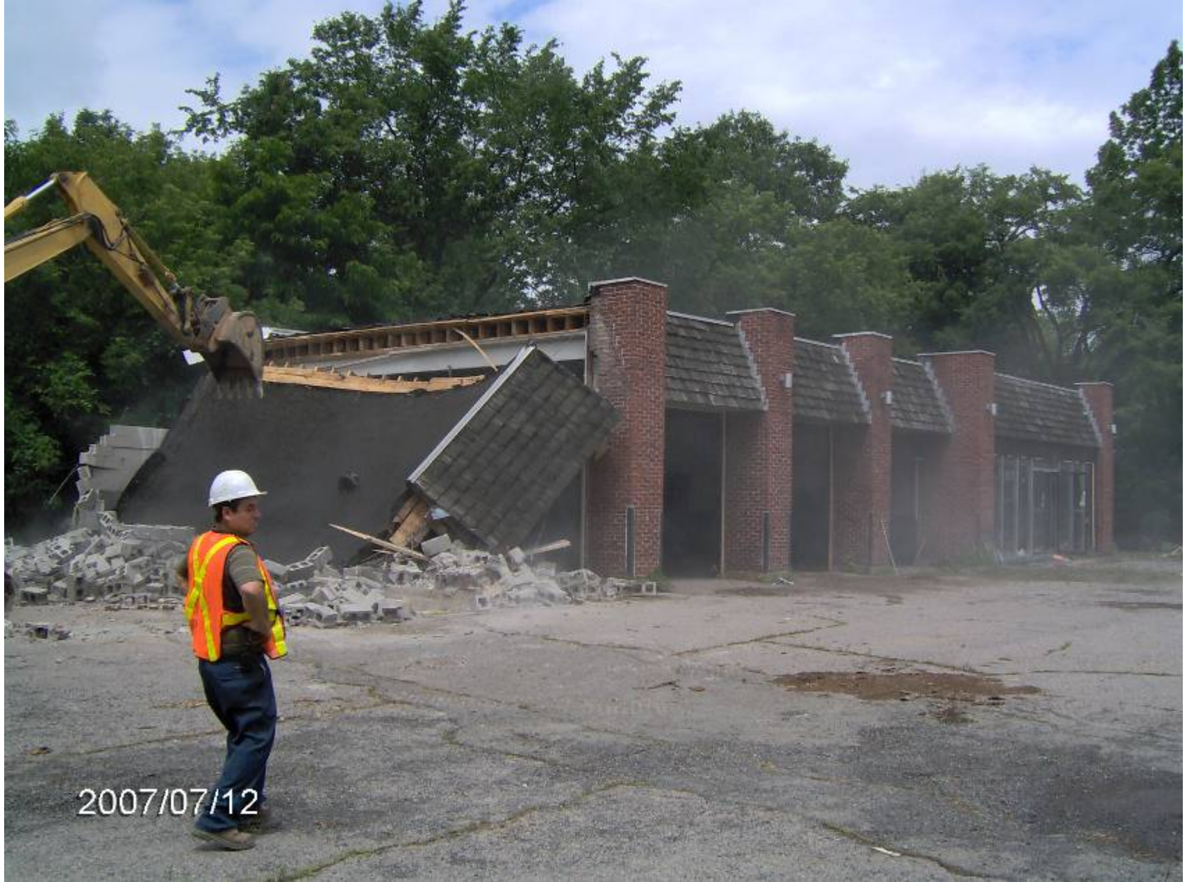
Waterloo Row ESSO Demolition, 2007-July-10
