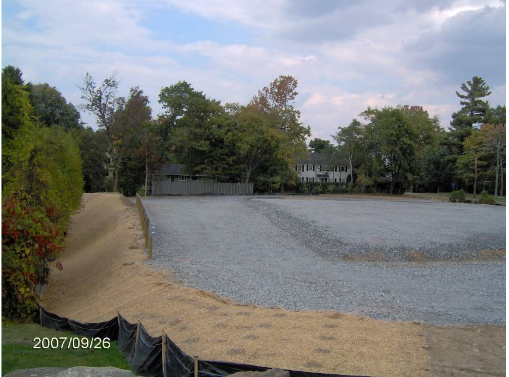
Erosion Control Mats, West Property line
