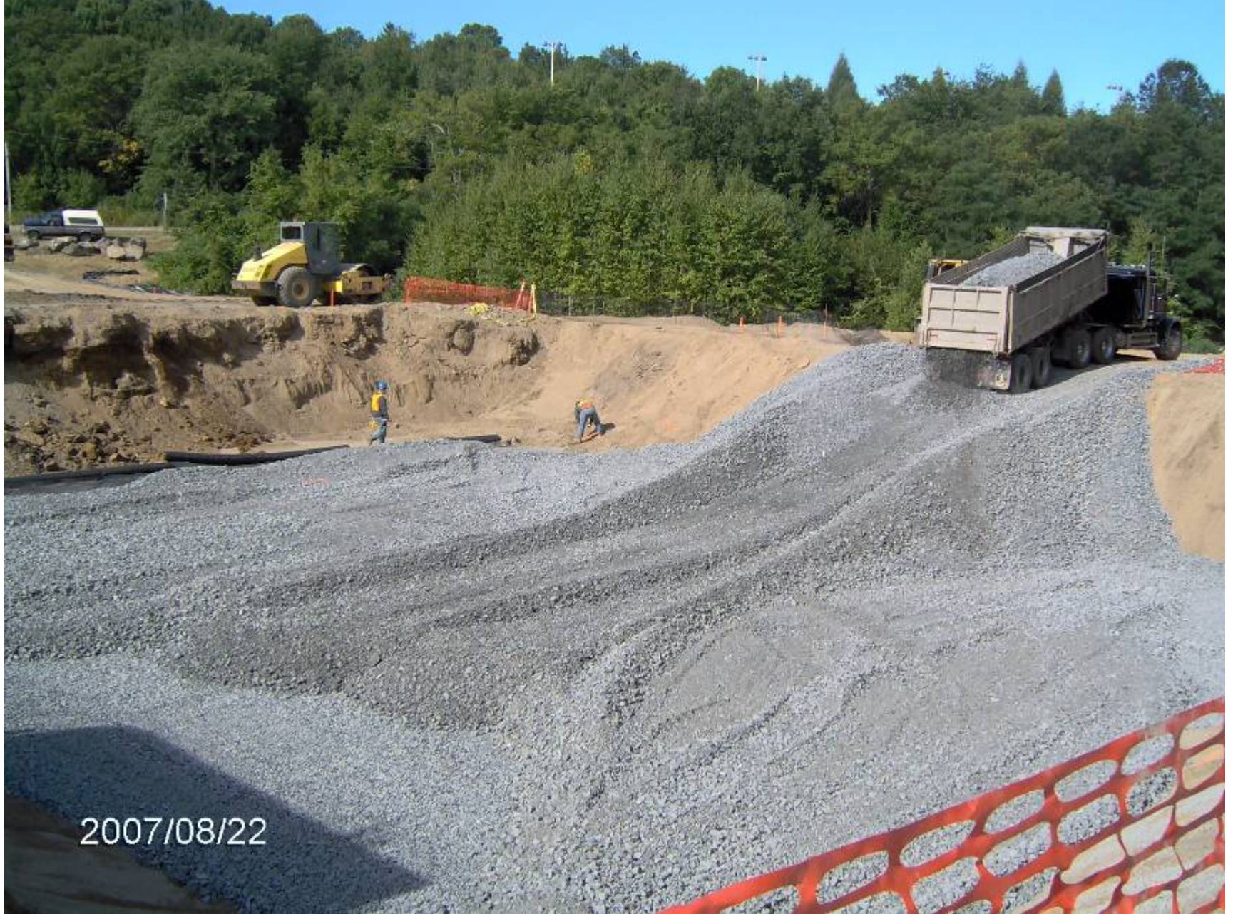
Engineered Pad, Water Treatment Building
