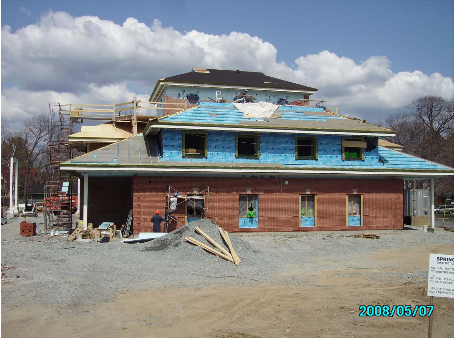
“South End of Building Exterior
