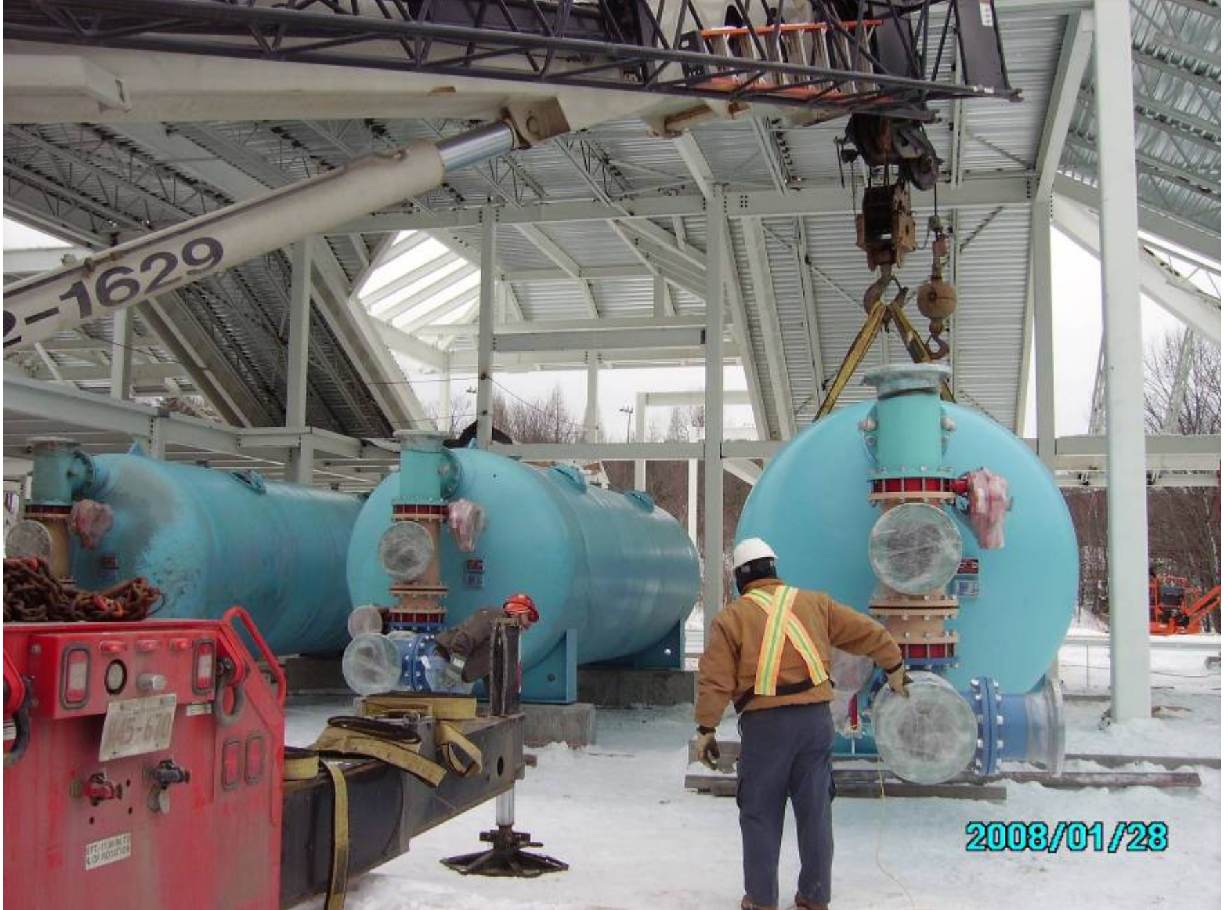
Arrival of Third Filter and Placement of Filters within Building
