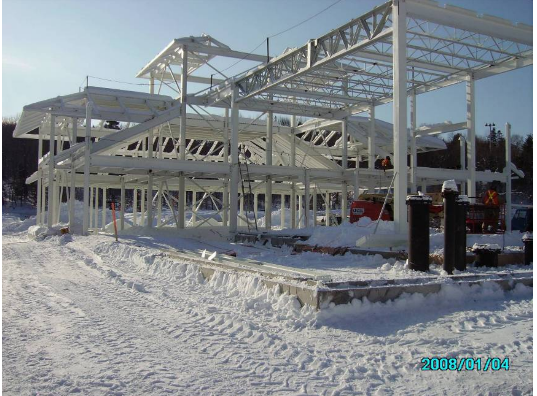
Filtration Room Roof
