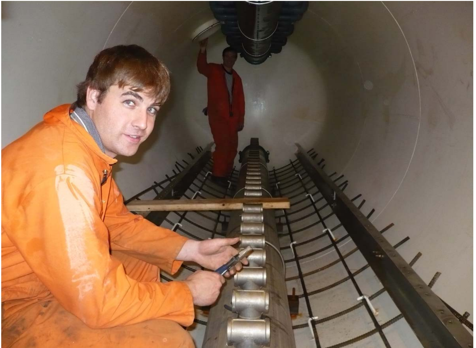
Inside Filter Vessel – Tie off of R-Bar
