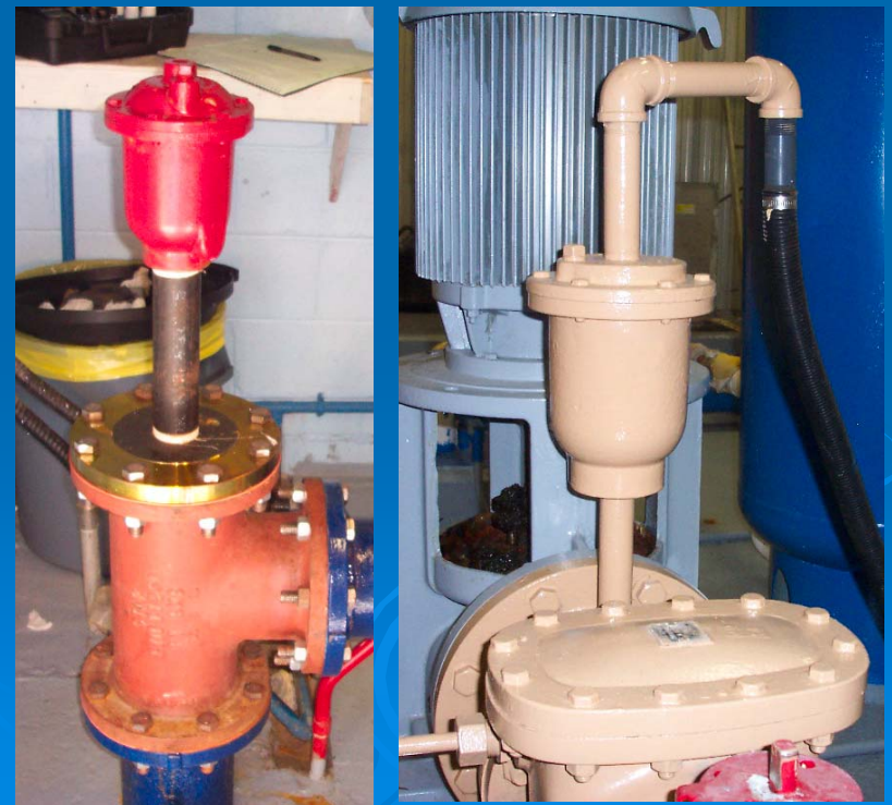
Air Release Valves
