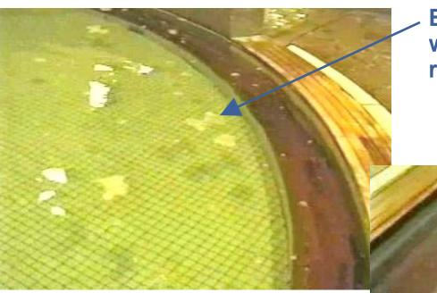
Biofilm sloughed into pool water, and was physically removed by operators
