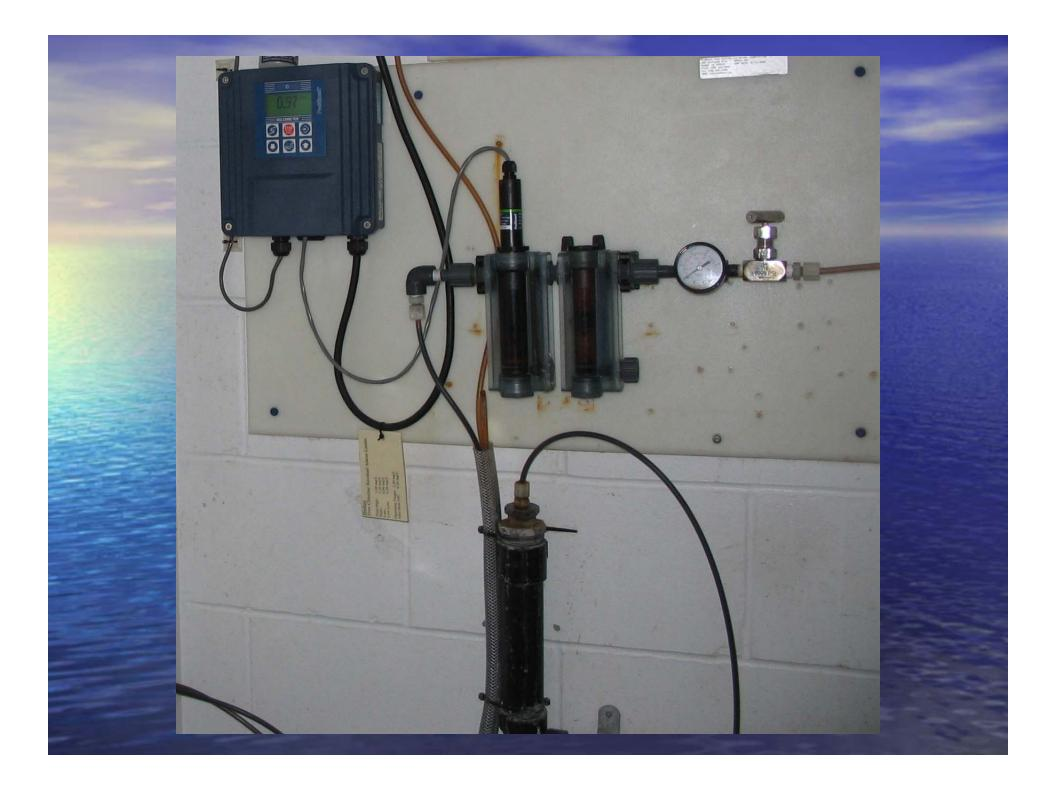
BASIC # 2 – CHLORINE ANALYZER AND CHART RECORDER CONNECTED TO PHONE LINE.
