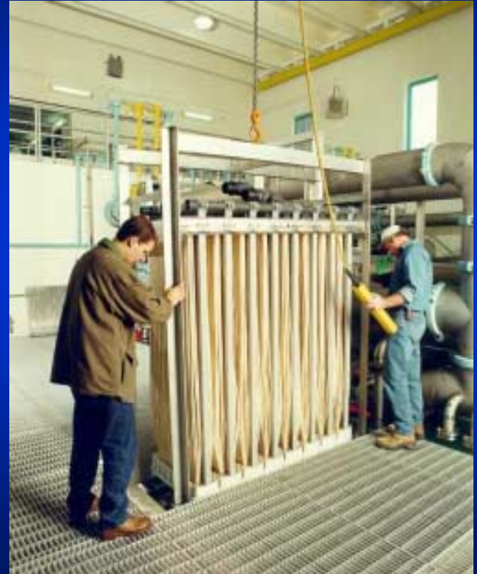
Single cassette of 8 ZeeWeed ZW500 immersed modules
