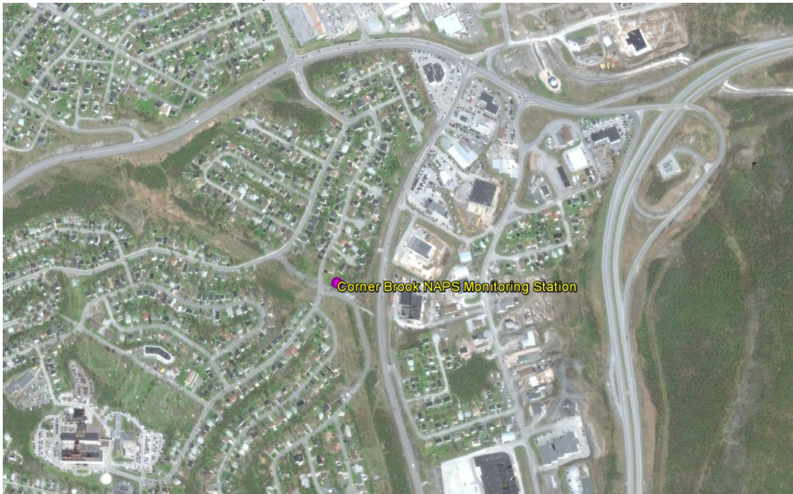
FIGURE 3.0.4 - NAPS AIR QUALITY MONITORING STATION IN CORNER BROOK
