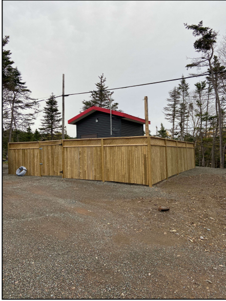
Figure 2: Hut Structure for groundwater well
