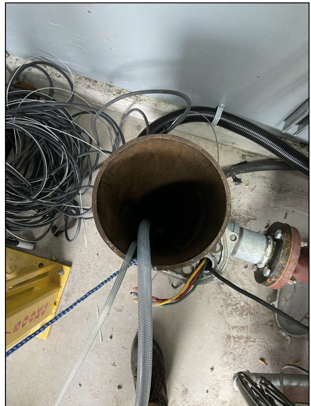
Figure 5: View looking into well
