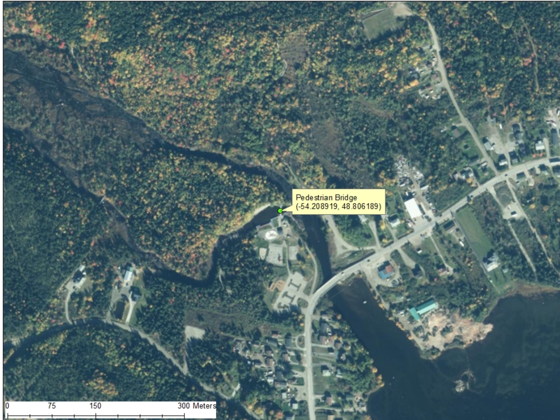
Repairs to an Existing Pedestrian Bridge, Town of Gambo
