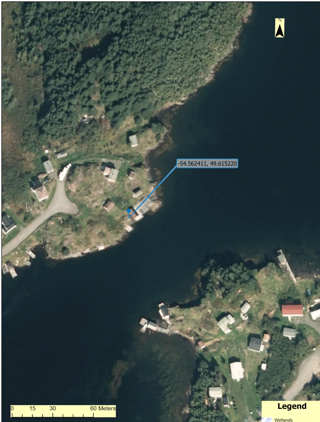
Community of Cobb's Arm (Roger's Cove) - Septic Outfall Pipe
