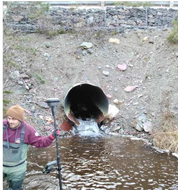
Photo 2: Downstream End of Structure
