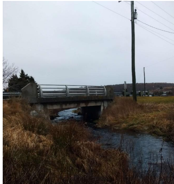
Photo 2: Downstream End of Structure
