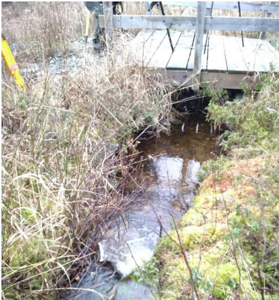
Photo 1: Upstream End of Structure
