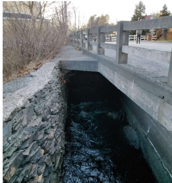
Photo 2: Downstream End of Structure
