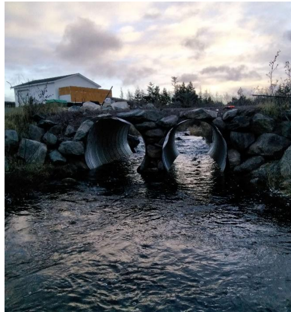
Photo 2: Downstream End of Structure
