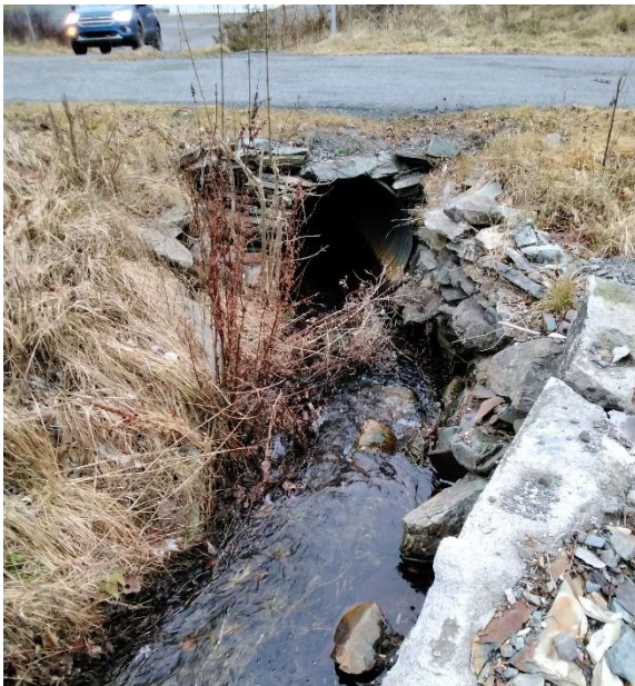
Photo 1: Upstream End of Structure
