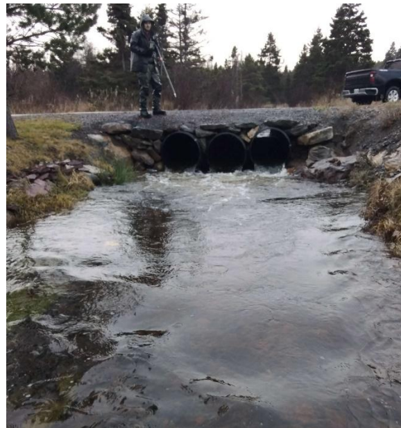
Photo 2: Downstream End of Structure
