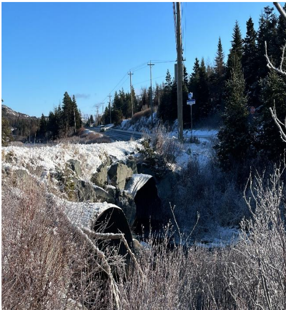
Photo 1: Upstream End of Structure
