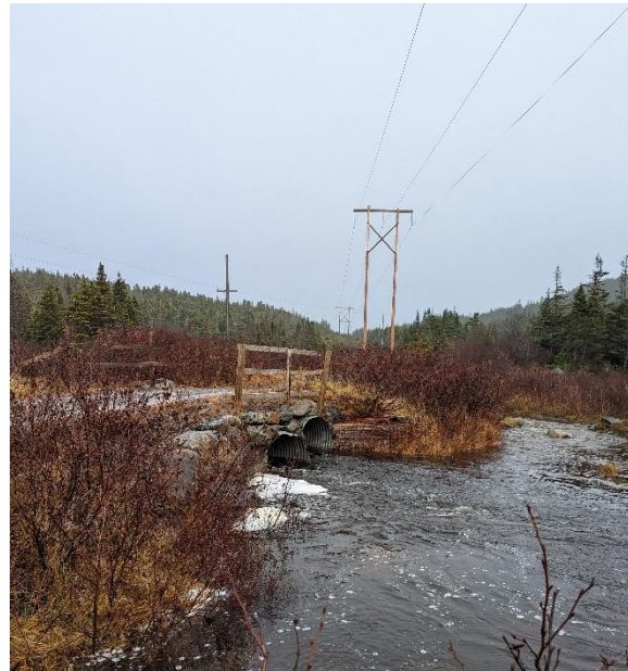
Photo 2: Downstream End of Structure
