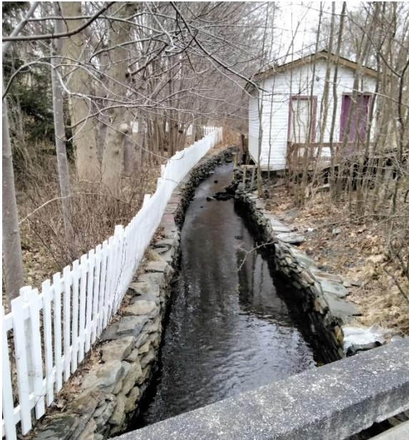
Photo 3: Looking Upstream from Structure
