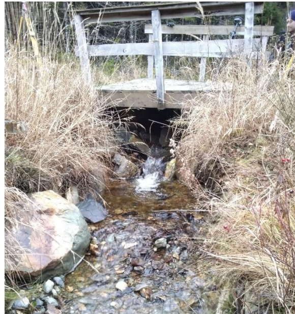
Photo 2: Downstream End of Structure
