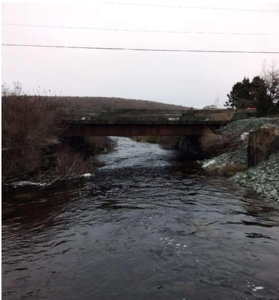
Photo 1: Upstream End of Structure
