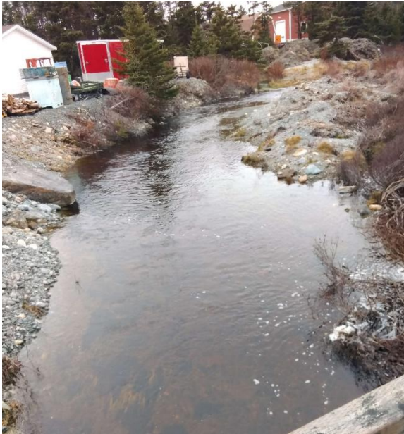
Photo 3: Looking Upstream from Structure
