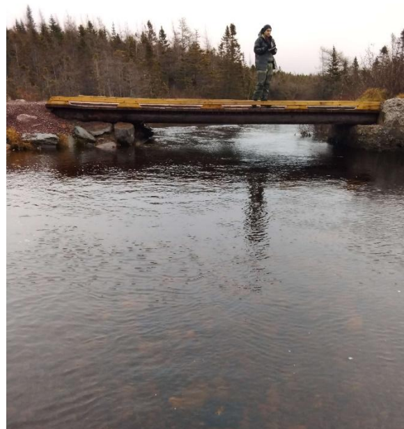
Photo 2: Downstream End of Structure
