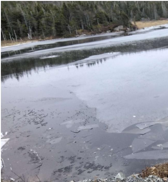
Photo 3: Looking Upstream from Structure
