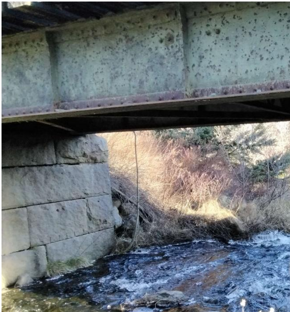
Photo 1: Upstream End of Structure
