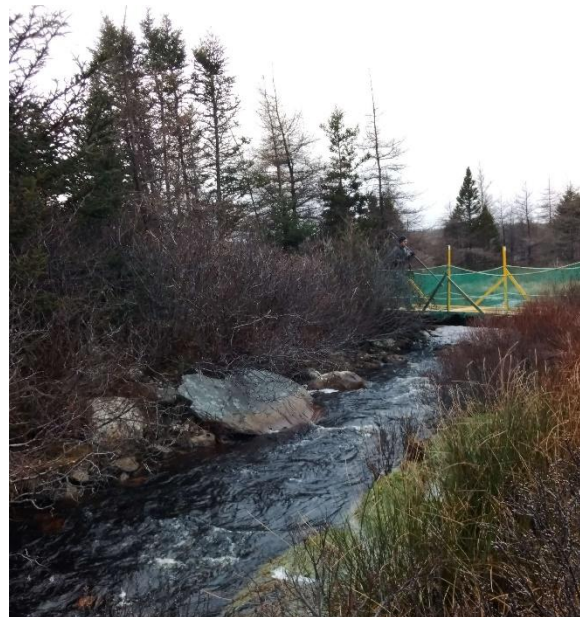
Photo 2: Downstream End of Structure
