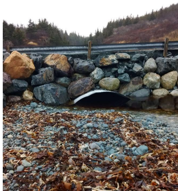
Photo 2: Downstream End of Structure
