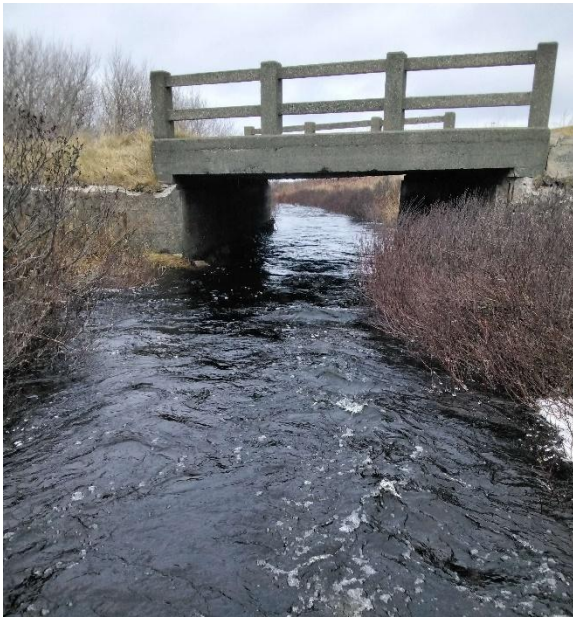
Photo 1: Upstream End of Structure
