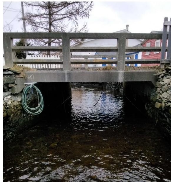
Photo 2: Downstream End of Structure
