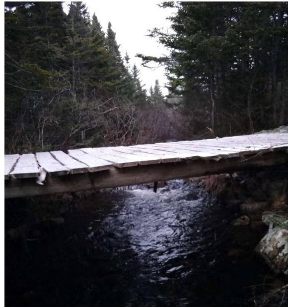
Photo 2: Downstream End of Structure
