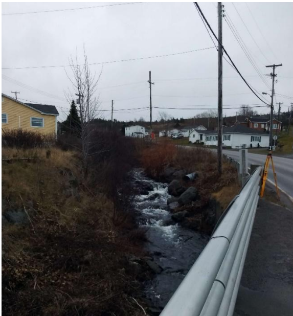
Photo 3: Looking Upstream from Structure
