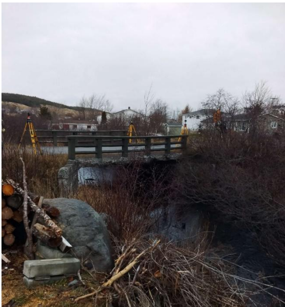
Photo 1: Upstream End of Structure
