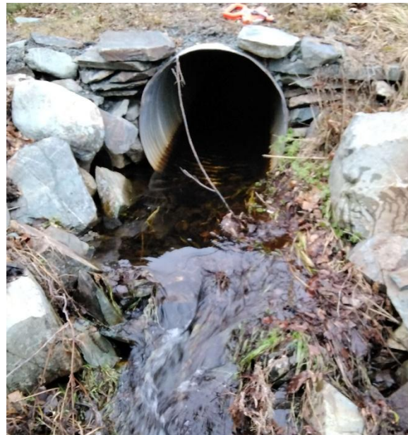
Photo 2: Downstream End of Structure
