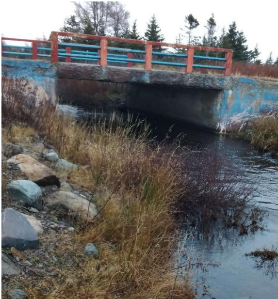
Photo 1: Upstream End of Structure
