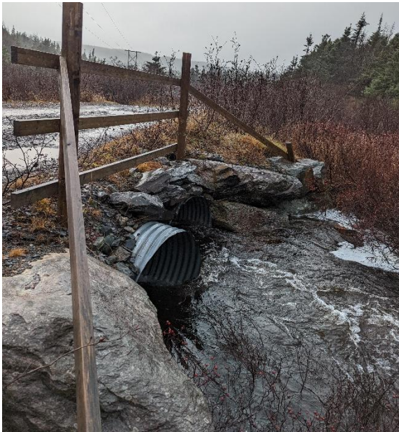
Photo 1: Upstream End of Structure
