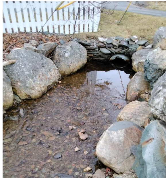
Photo 2: Downstream End of Structure
