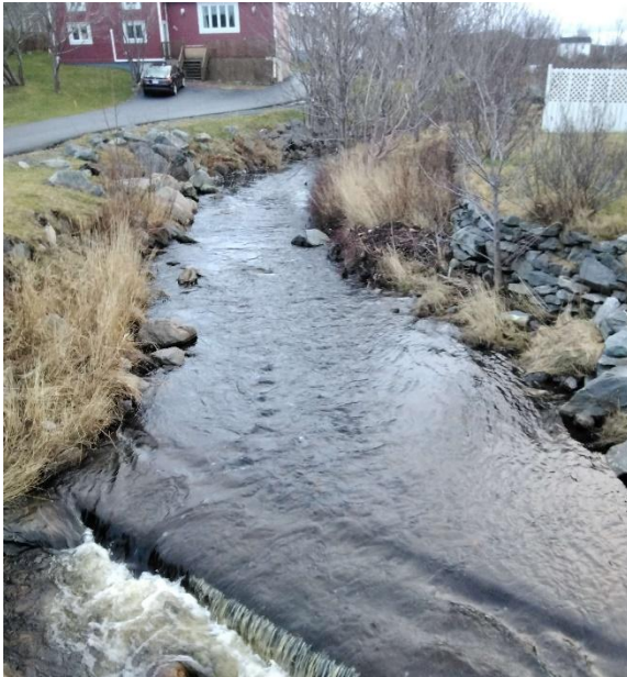
Photo 3: Looking Upstream from Structure
