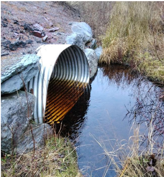
Photo 1: Upstream End of Structure
