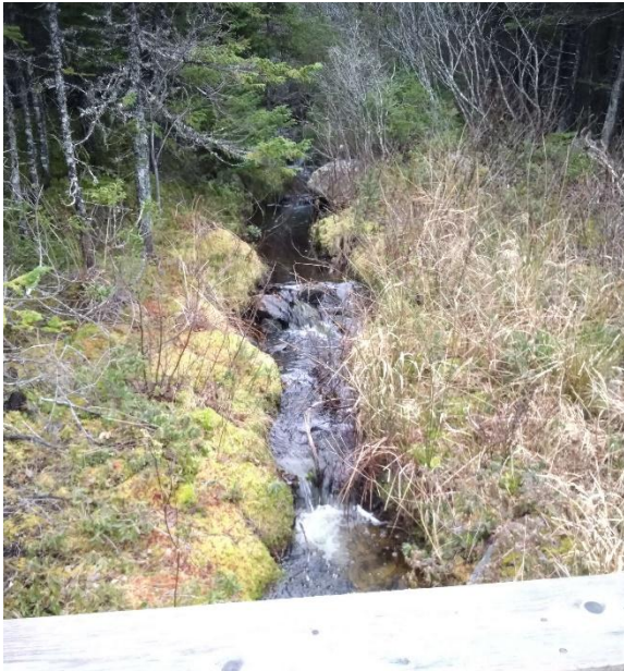
Photo 3: Looking Upstream from Structure
