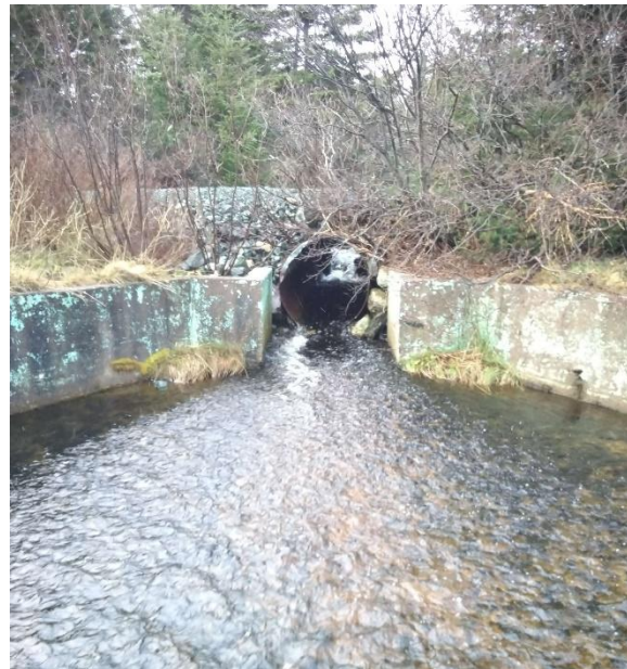
Photo 2: Downstream End of Structure
