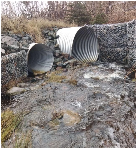
Photo 1: Upstream End of Structure
