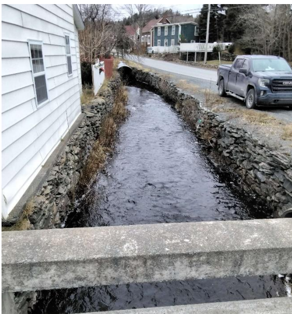
Photo 3: Looking Upstream from Structure
