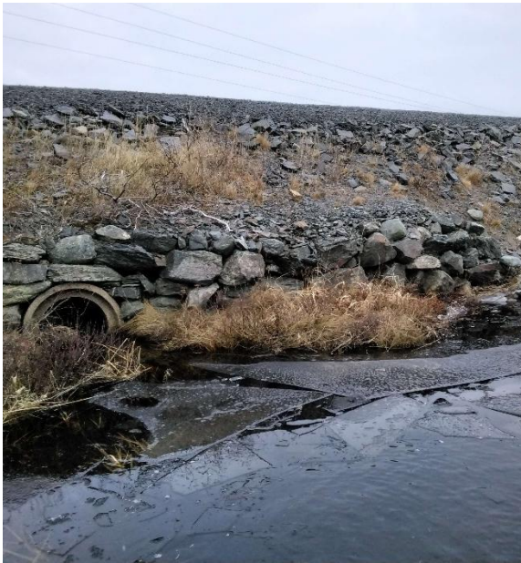
Photo 1: Upstream End of Structure
