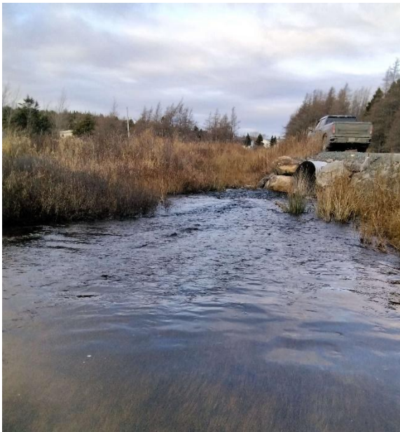
Photo 1: Upstream End of Structure
