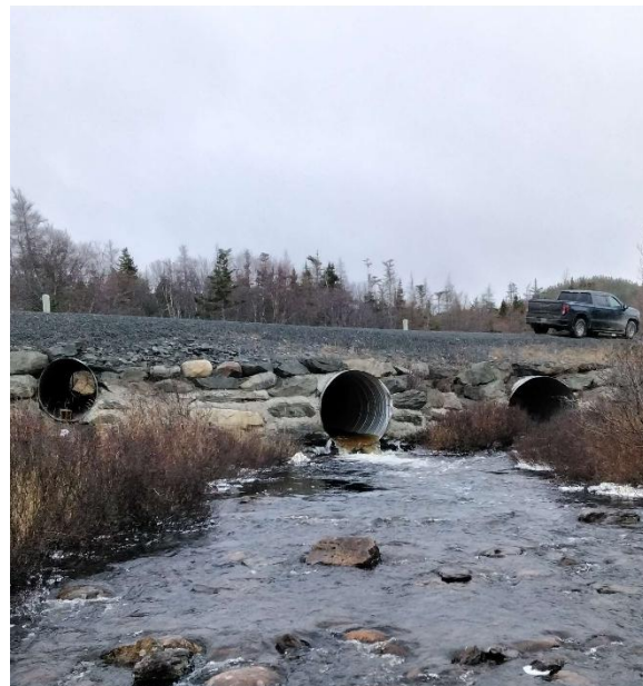
Photo 2: Downstream End of Structure
