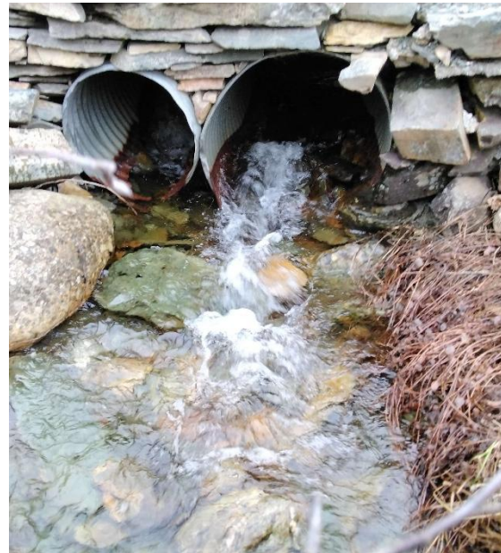
Photo 2: Downstream End of Structure
