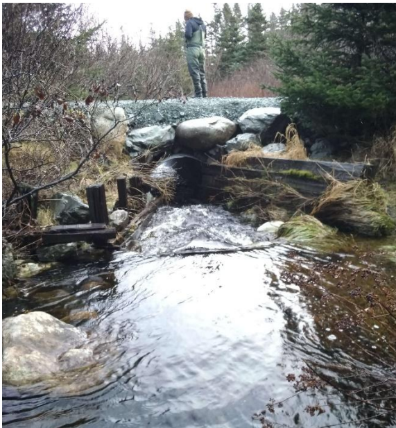
Photo 1: Upstream End of Structure
