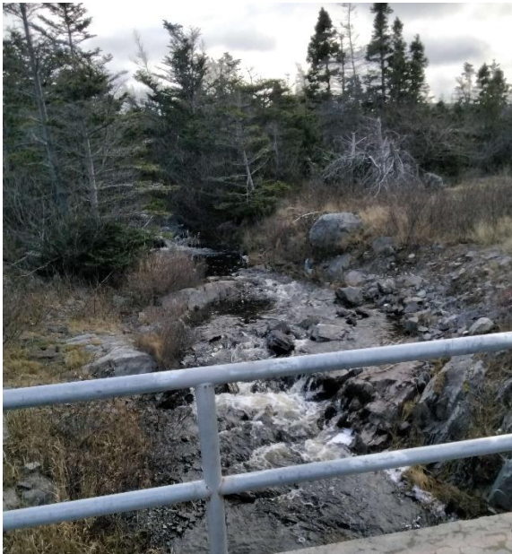
Photo 3: Looking Upstream from Structure
