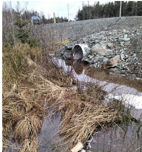
Photo 2: Downstream End of Structure
