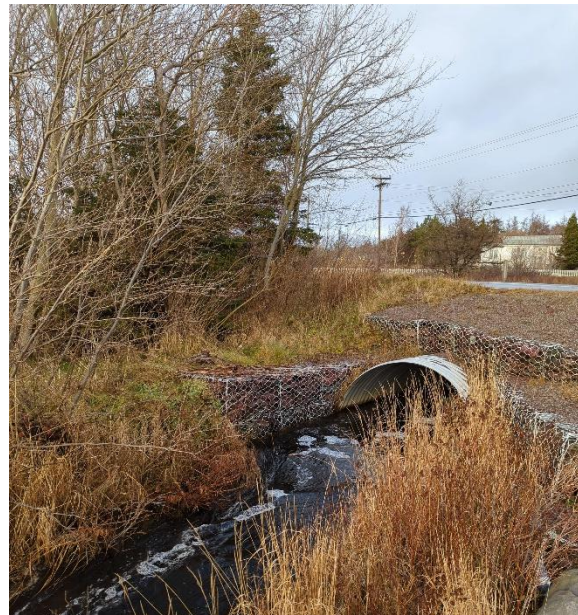
Photo 2: Downstream End of Structure
