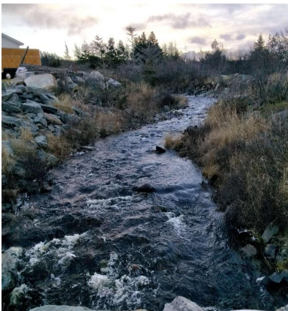
Photo 3: Looking Upstream from Structure
