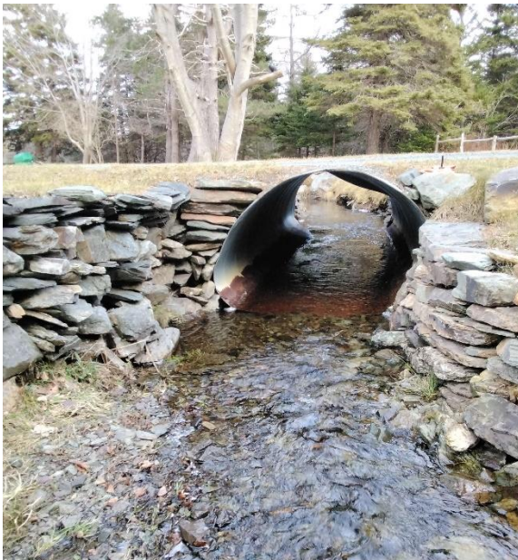
Photo 1: Upstream End of Structure
