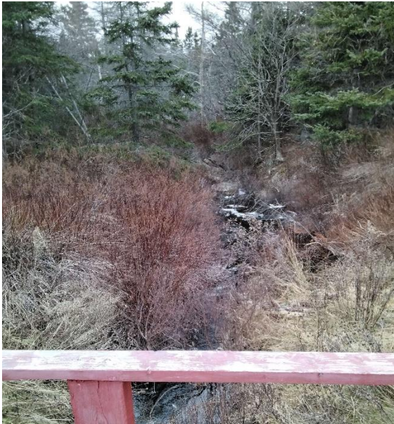
Photo 3: Looking Upstream from Structure
