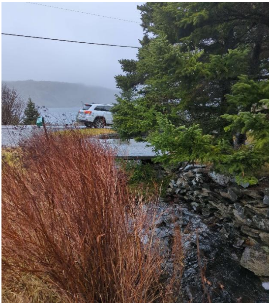
Photo 1: Upstream End of Structure
