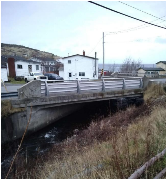
Photo 1: Upstream End of Structure
