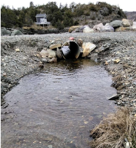
Photo 1: Upstream End of Structure
