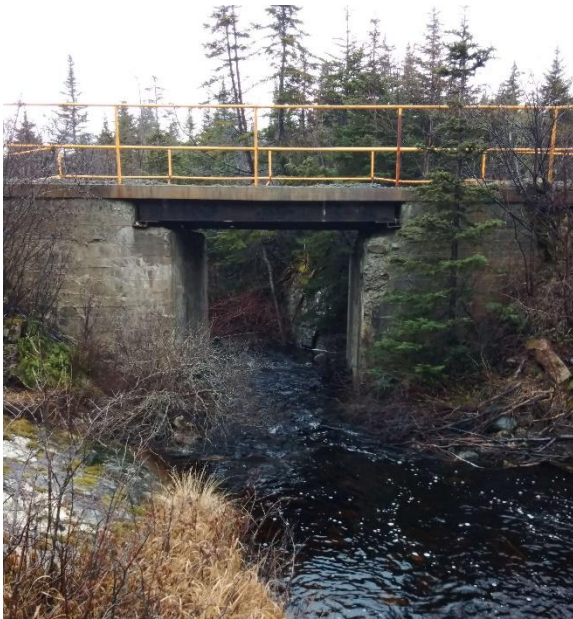
Photo 1: Upstream End of Structure
