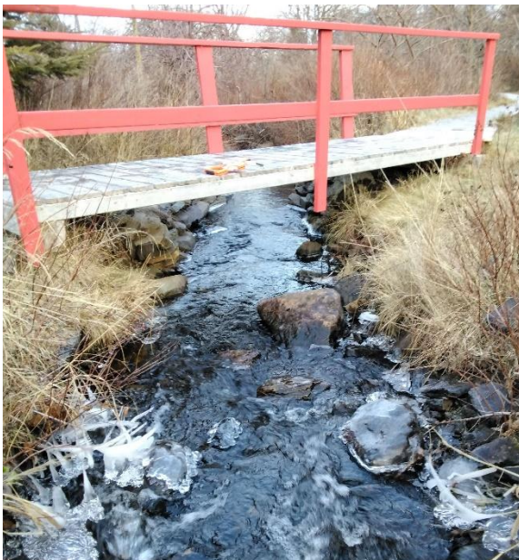
Photo 1: Upstream End of Structure
