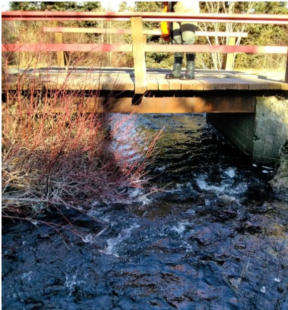
Photo 1: Upstream End of Structure
