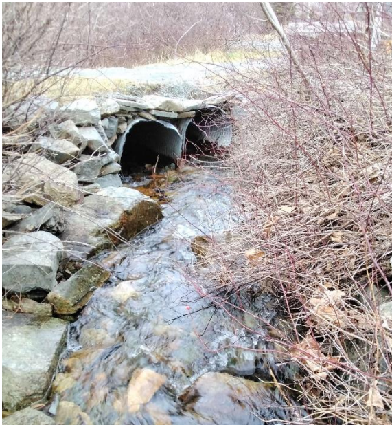
Photo 1: Upstream End of Structure
