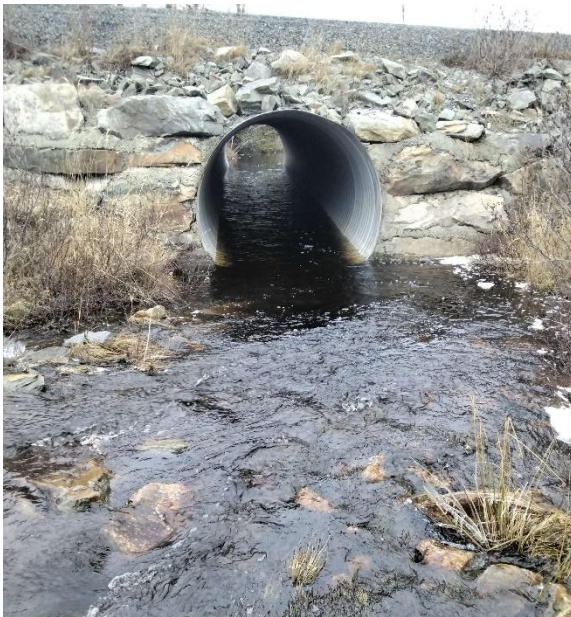
Photo 1: Upstream End of Structure
