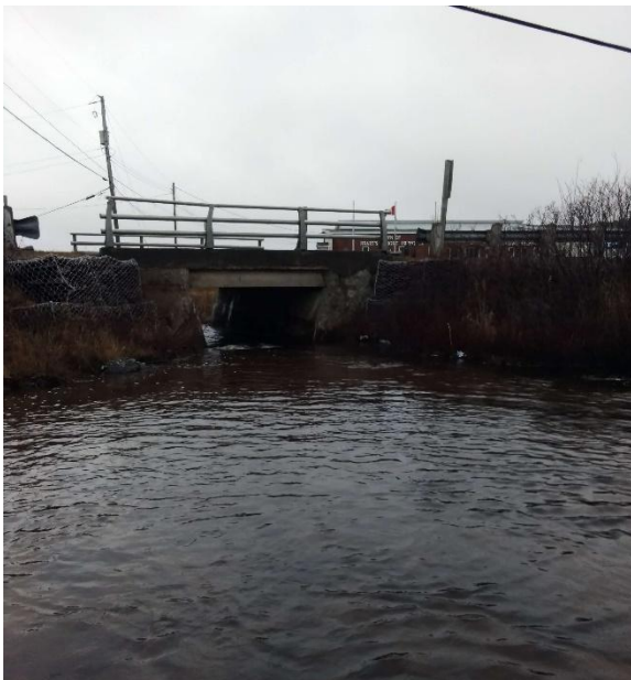
Photo 1: Upstream End of Structure
