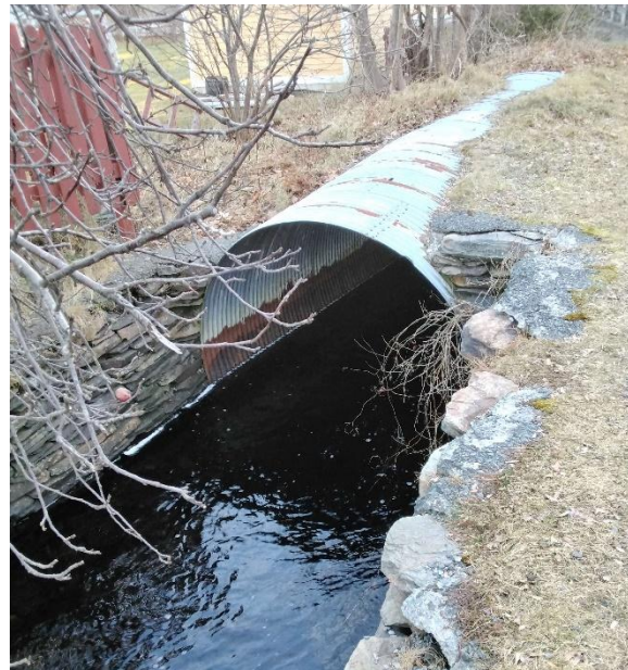
Photo 2: Downstream End of Structure
