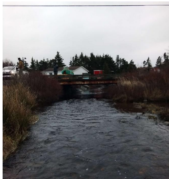
Photo 2: Downstream End of Structure
