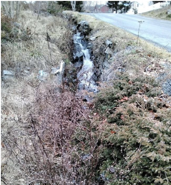
Photo 3: Looking Upstream from Structure
