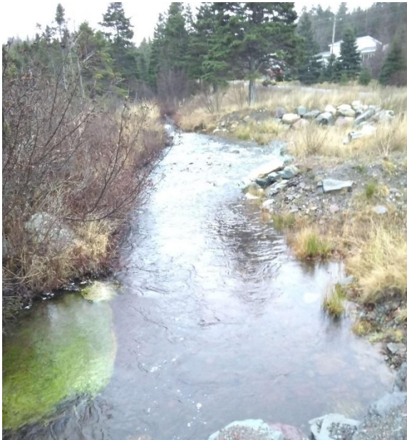
Photo 3: Looking Upstream from Structure
