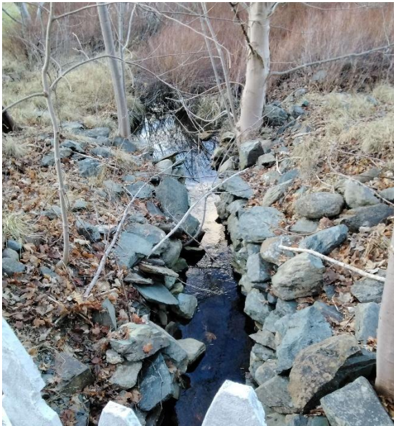
Photo 3: Looking Upstream from Structure
