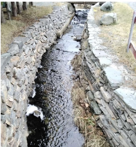
Photo 3: Looking Upstream from Structure
