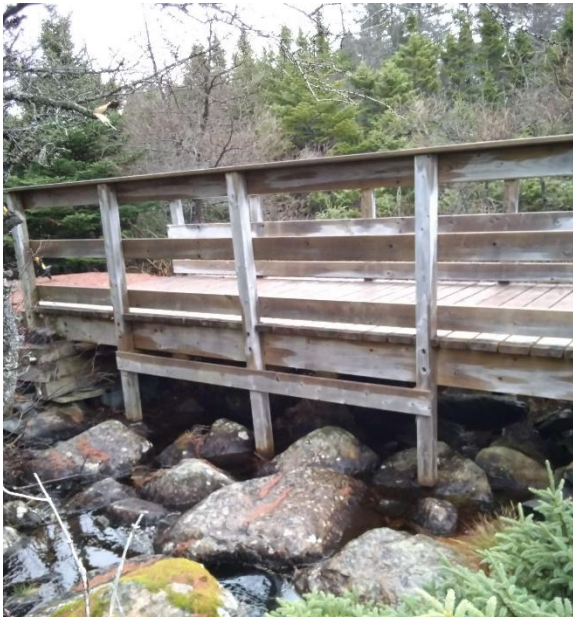
Photo 1: Upstream End of Structure
