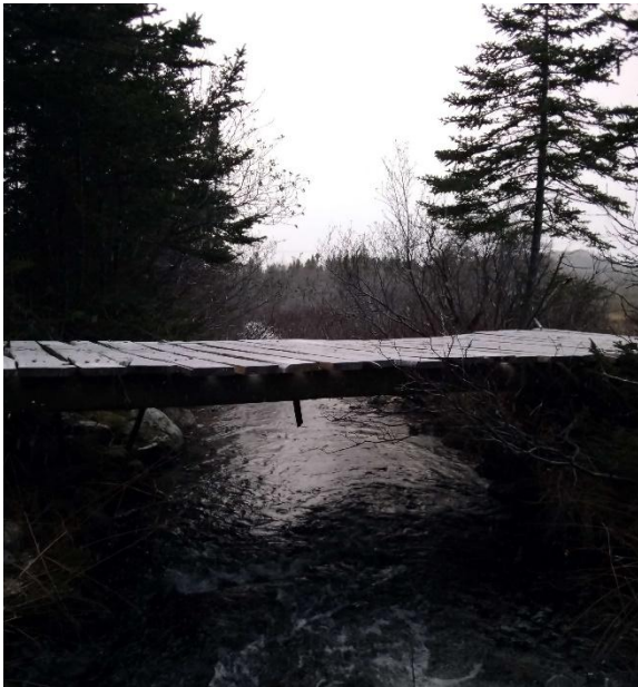
Photo 1: Upstream End of Structure
