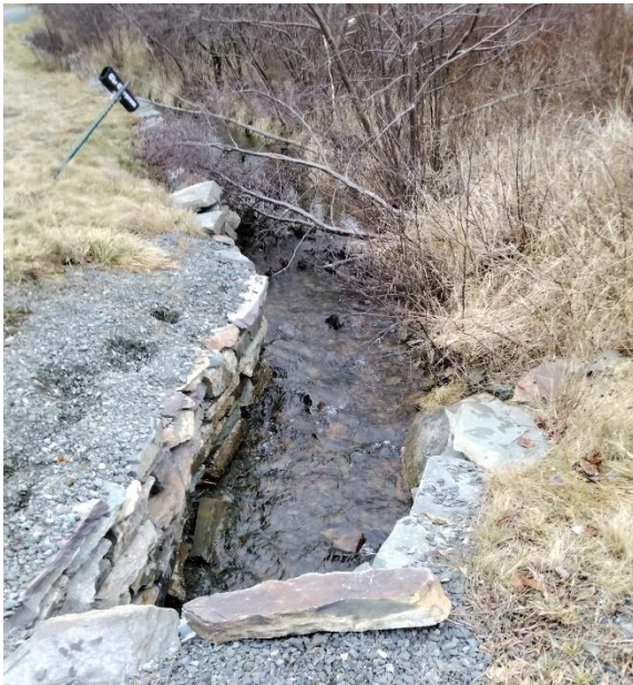
Photo 3: Looking Upstream from Structure
