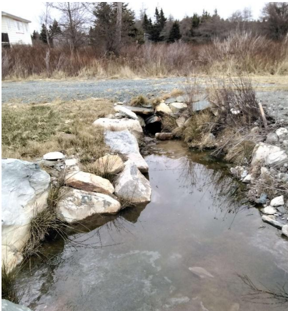
Photo 1: Upstream End of Structure
