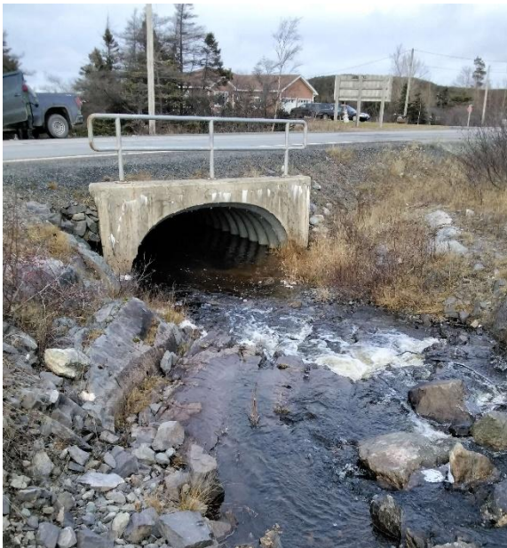
Photo 1: Upstream End of Structure
