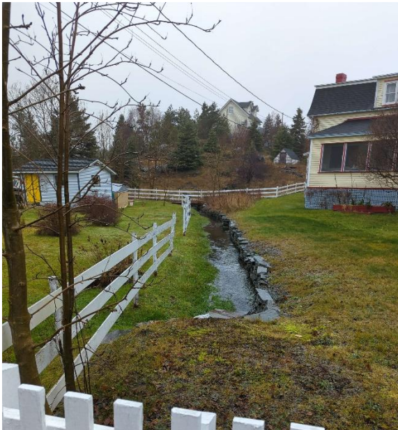
Photo 3: Looking Upstream from Structure
