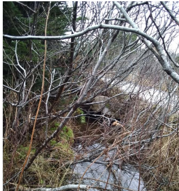
Photo 2: Downstream End of Structure
