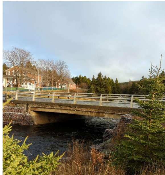
Photo 2: Downstream End of Structure
