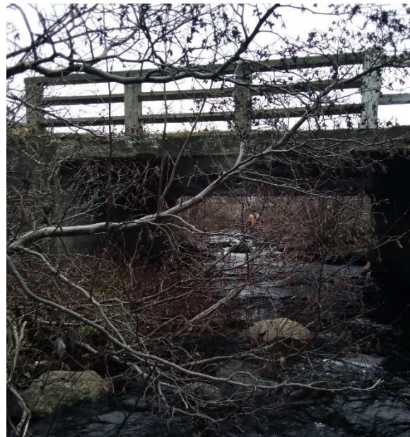
Photo 2: Downstream End of Structure
