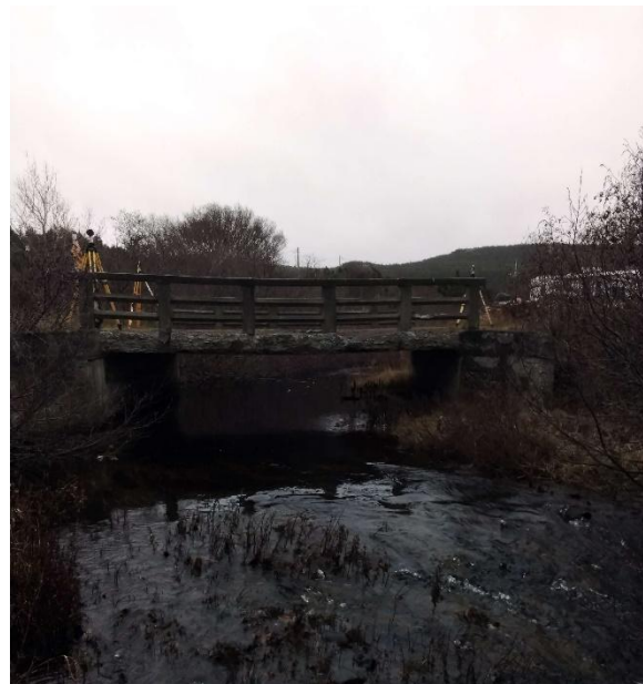
Photo 2: Downstream End of Structure
