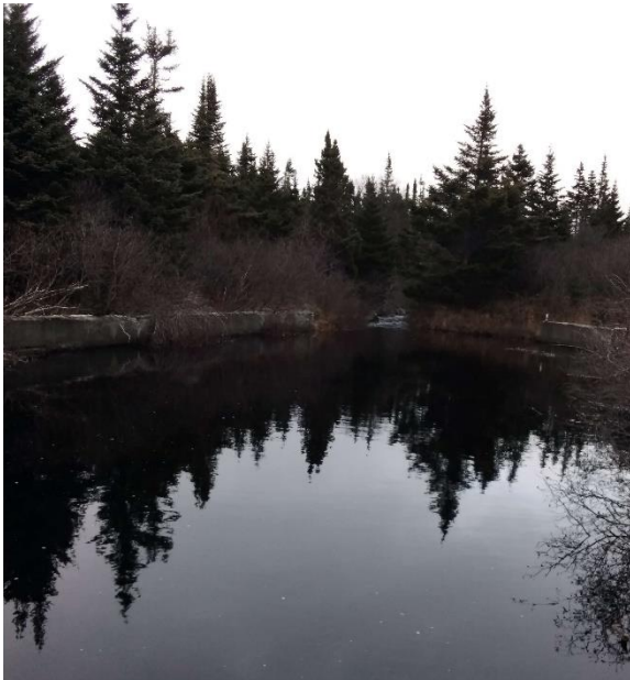
Photo 3: Looking Upstream from Structure
