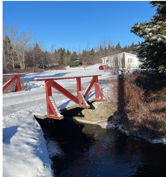
Photo 2: Downstream End of Structure
