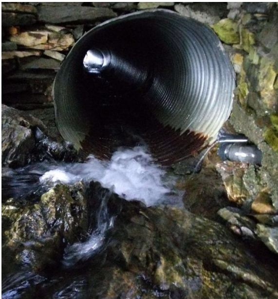
Photo 1: Upstream End of Structure
