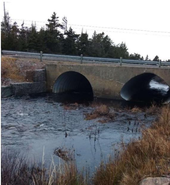
Photo 1: Upstream End of Structure
