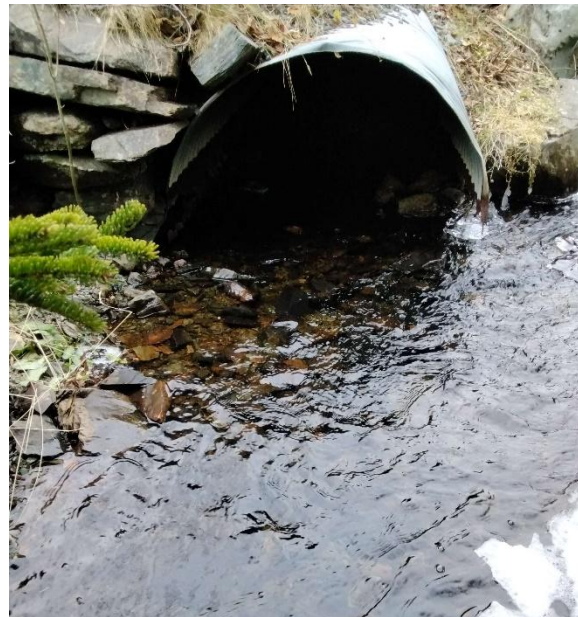
Photo 2: Downstream End of Structure
