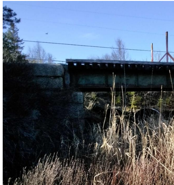
Photo 2: Downstream End of Structure
