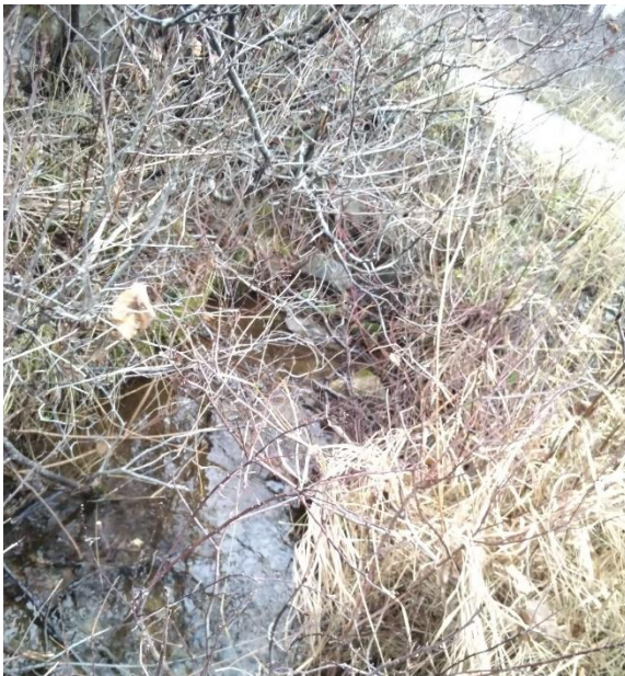
Photo 1: Upstream End of Structure
