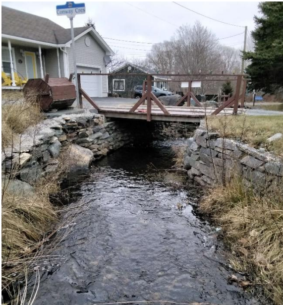
Photo 1: Upstream End of Structure
