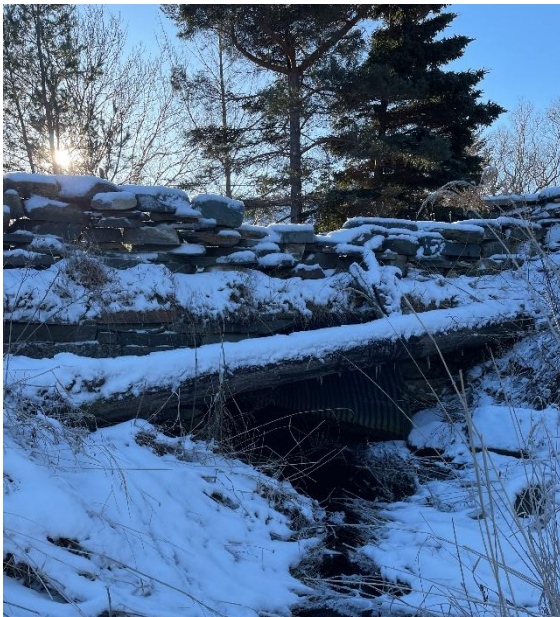
Photo 1: Upstream End of Structure
