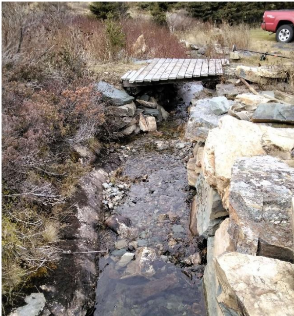
Photo 1: Upstream End of Structure
