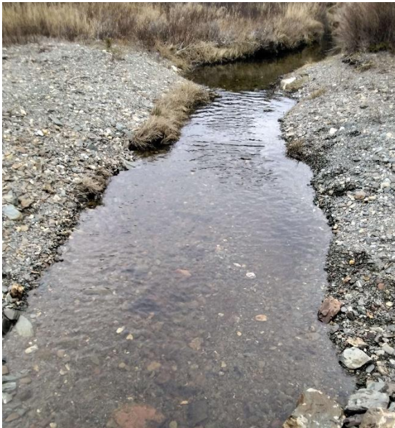
Photo 3: Looking Upstream from Structure
