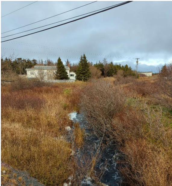
Photo 3: Looking Upstream from Structure
