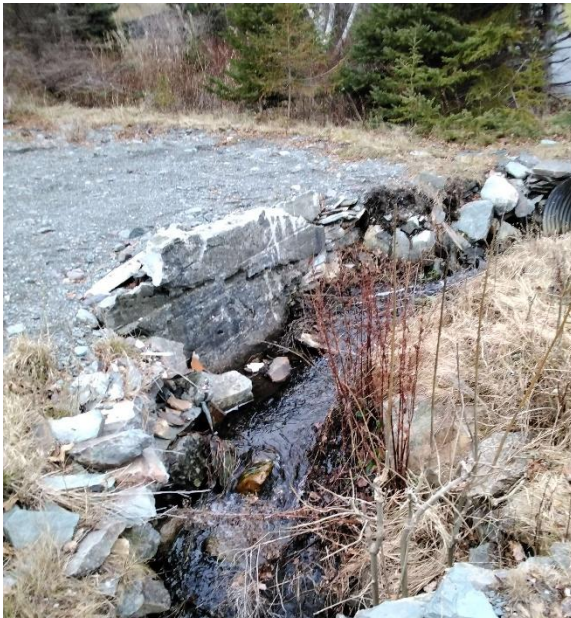
Photo 3: Looking Upstream from Structure
