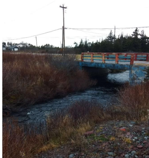
Photo 2: Downstream End of Structure
