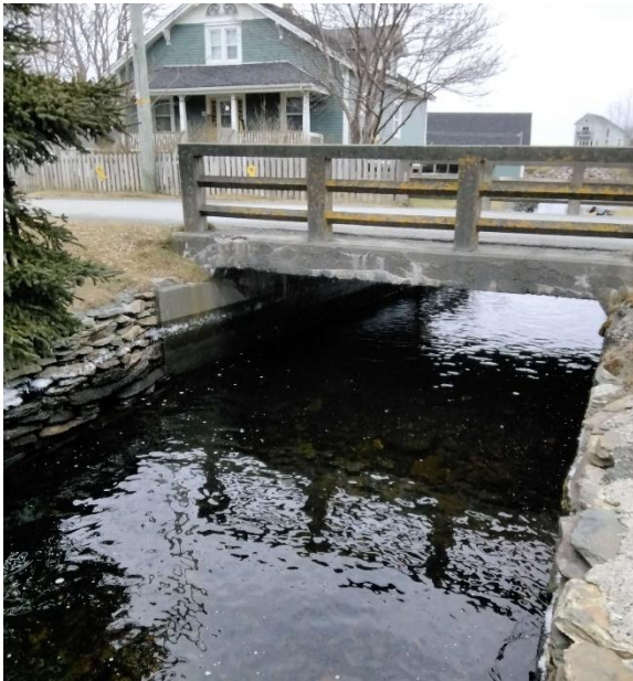
Photo 1: Upstream End of Structure
