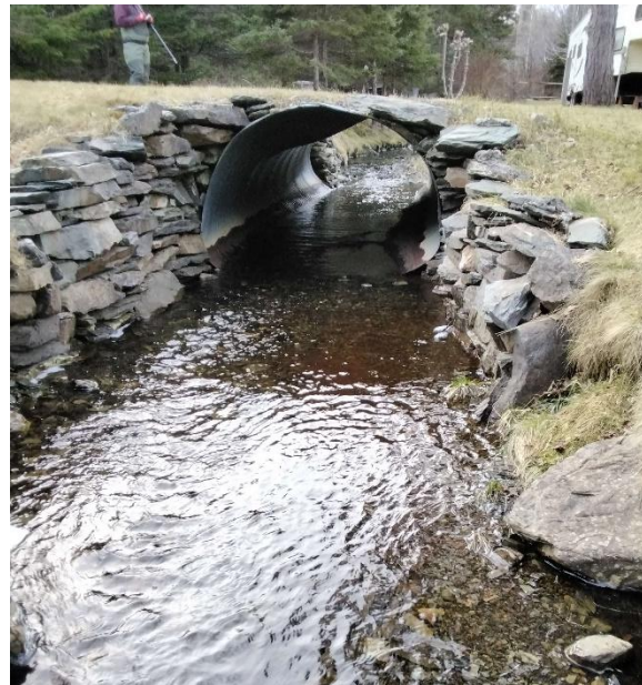
Photo 2: Downstream End of Structure
