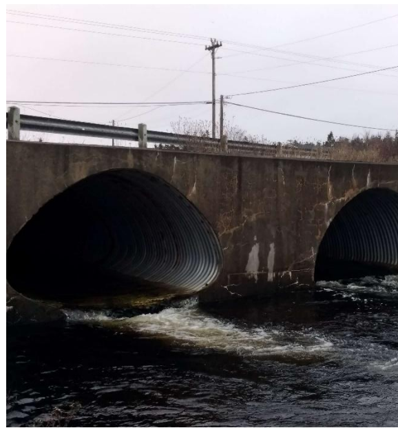
Photo 2: Downstream End of Structure
