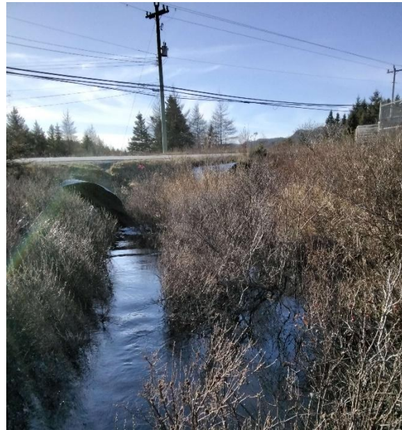
Photo 2: Downstream End of Structure
