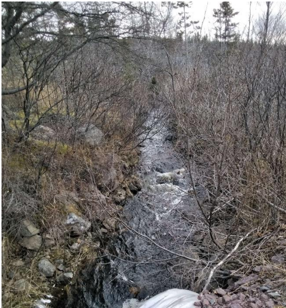
Photo 3: Looking Upstream from Structure
