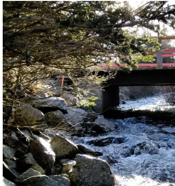
Photo 2: Downstream End of Structure
