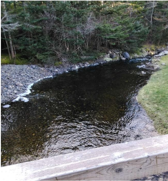
Photo 3: Looking Upstream from Structure
