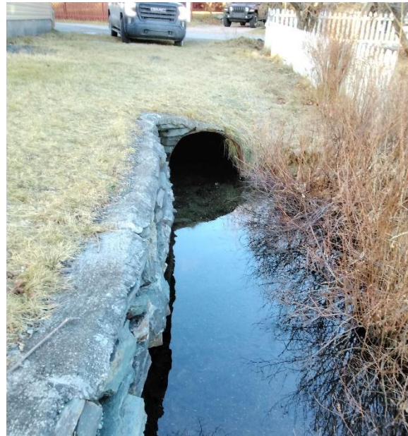
Photo 2: Downstream End of Structure
