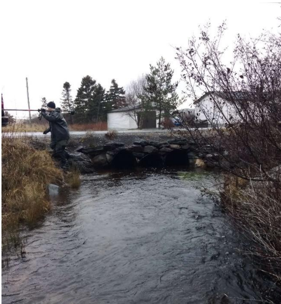
Photo 1: Upstream End of Structure
