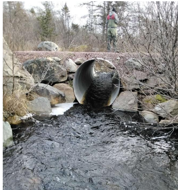
Photo 2: Downstream End of Structure
