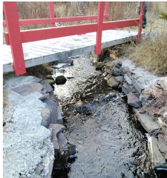
Photo 2: Downstream End of Structure
