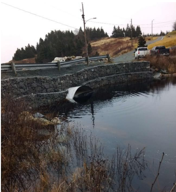
Photo 1: Upstream End of Structure
