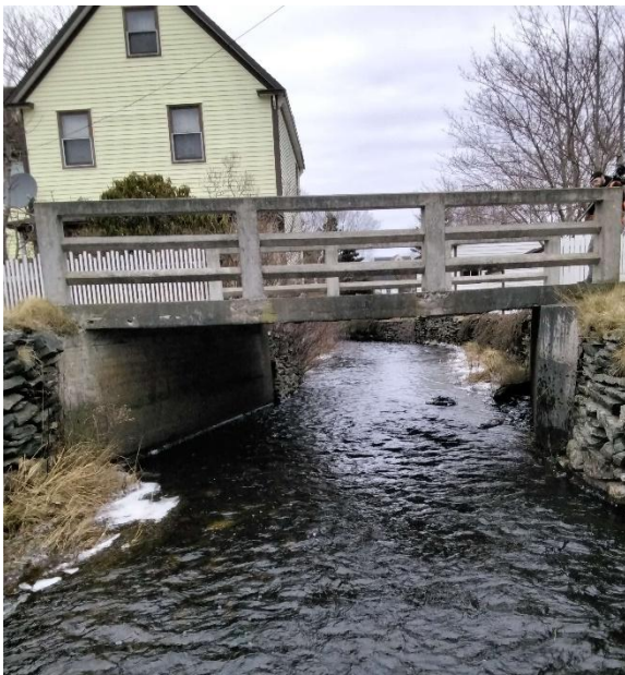
Photo 1: Upstream End of Structure
