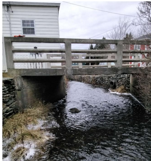
Photo 2: Downstream End of Structure
