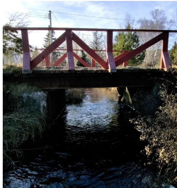
Photo 2: Downstream End of Structure
