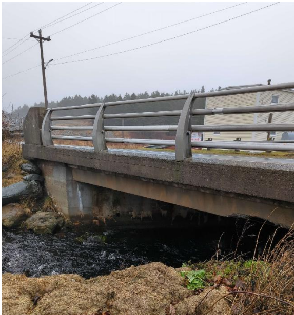
Photo 1: Upstream End of Structure
