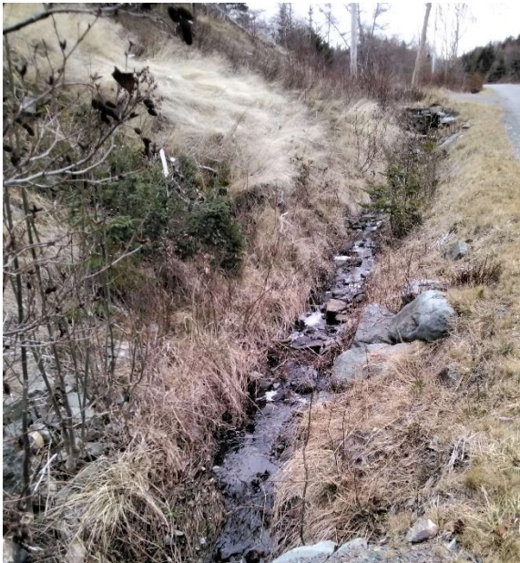
Photo 3: Looking Upstream from Structure
