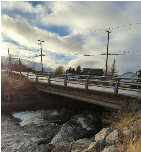
Photo 1: Upstream End of Structure
