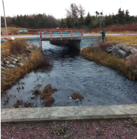
Photo 3: Looking Upstream from Structure
