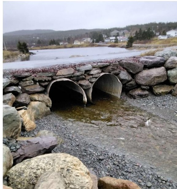
Photo 2: Downstream End of Structure
