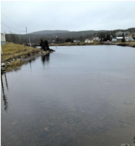
Photo 3: Looking Upstream from Structure
