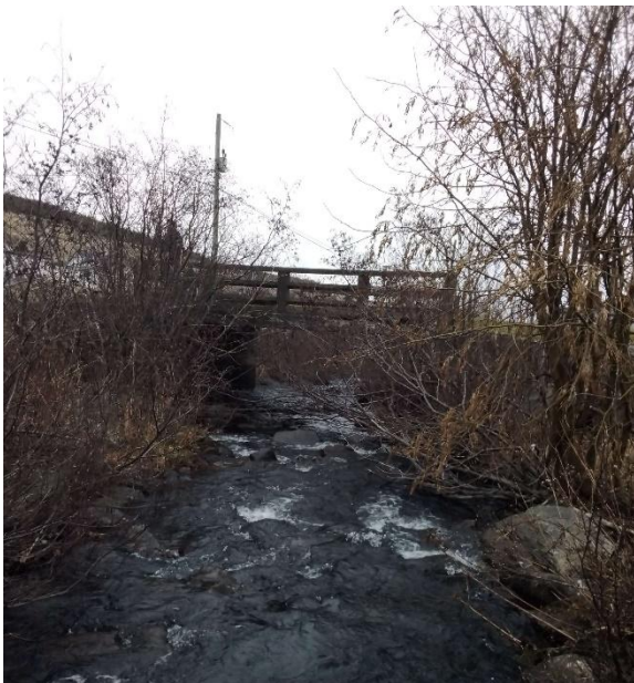
Photo 1: Upstream End of Structure
