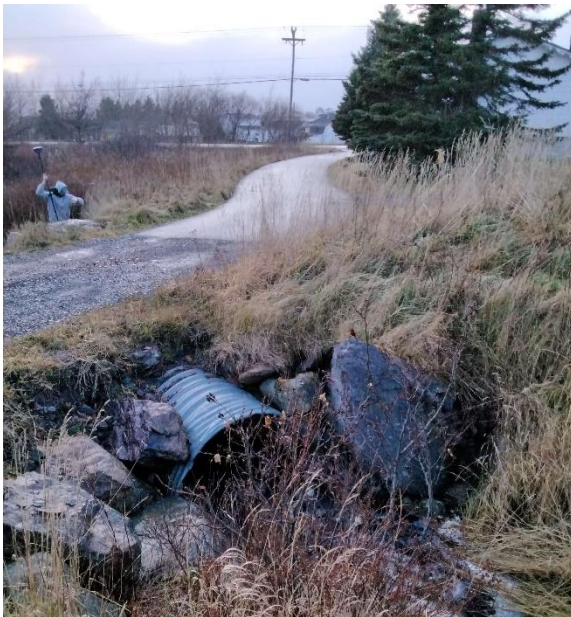
Photo 1: Upstream End of Structure
