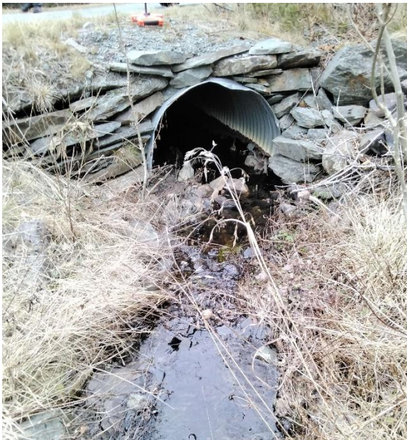
Photo 1: Upstream End of Structure
