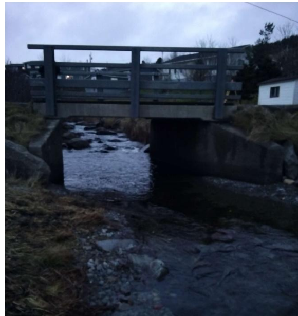
Photo 2: Downstream End of Structure
