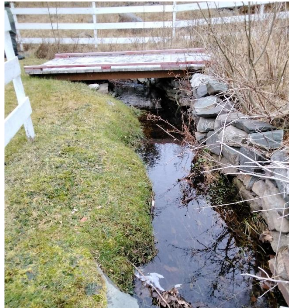
Photo 2: Downstream End of Structure
