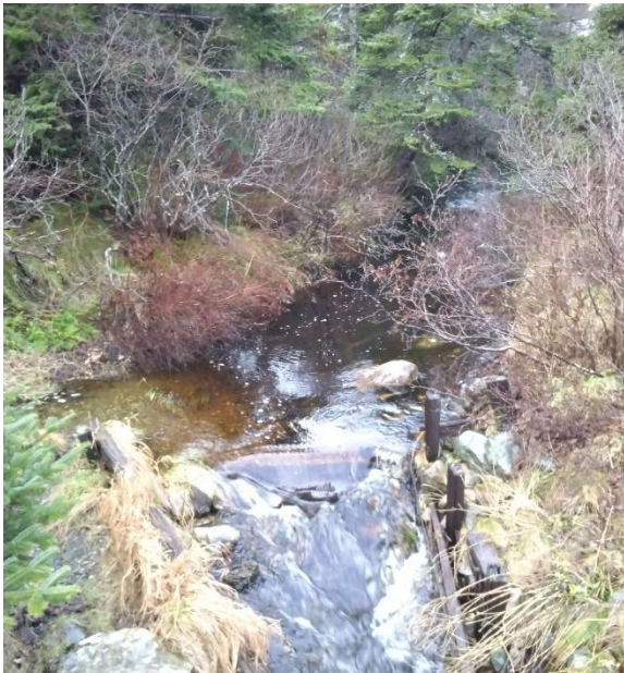
Photo 3: Looking Upstream from Structure
