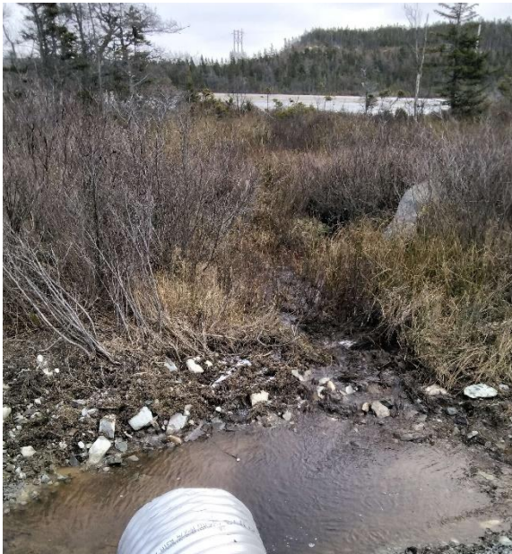
Photo 3: Looking Upstream from Structure
