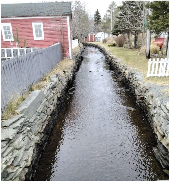
Photo 3: Looking Upstream from Structure
