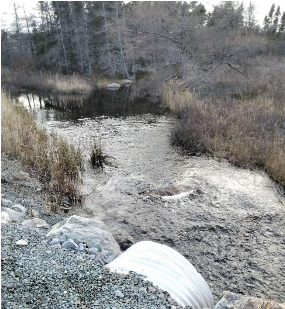
Photo 3: Looking Upstream from Structure
