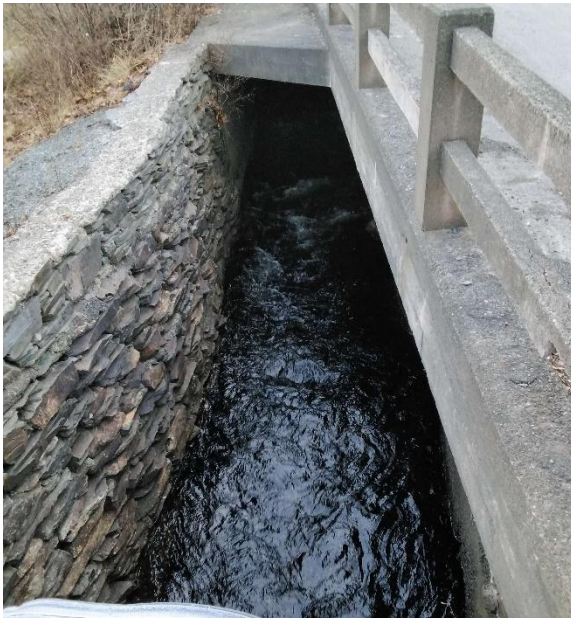
Photo 3: Looking Upstream from Structure
