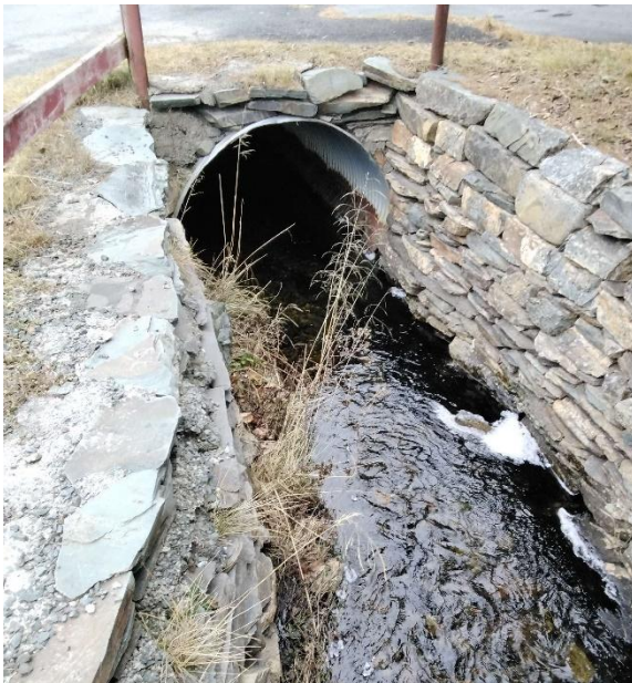
Photo 1: Upstream End of Structure
