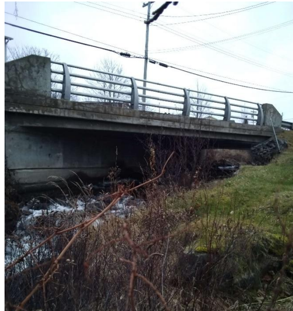
Photo 2: Downstream End of Structure
