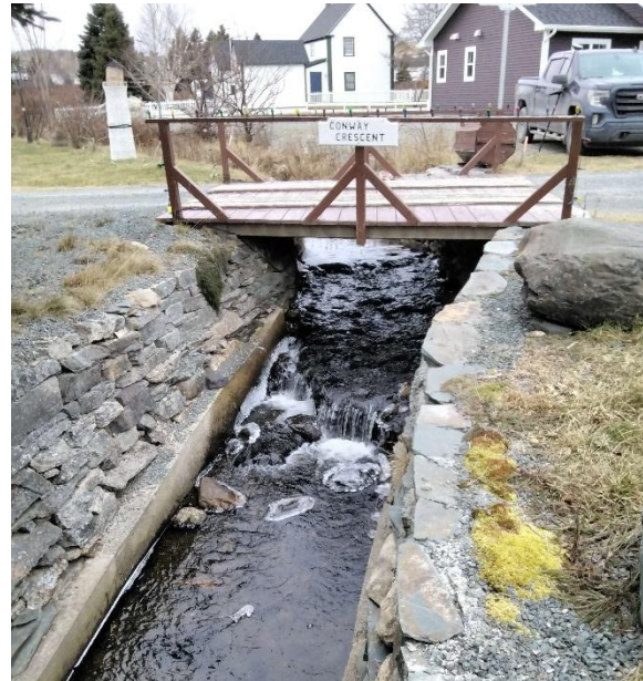
Photo 2: Downstream End of Structure
