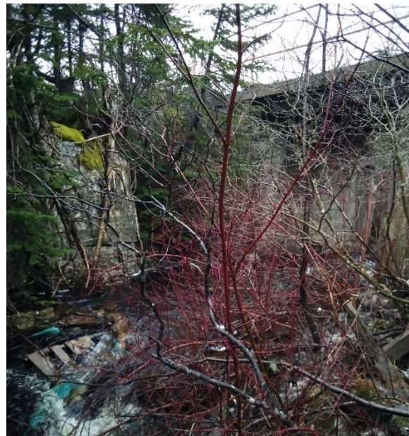
Photo 2: Downstream End of Structure
