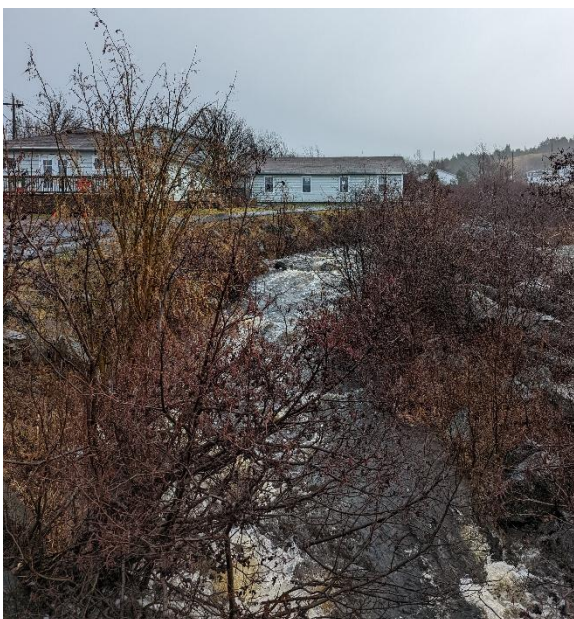
Photo 3: Looking Upstream from Structure
