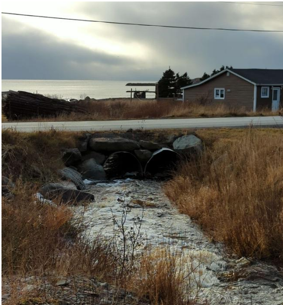
Photo 1: Upstream End of Structure
