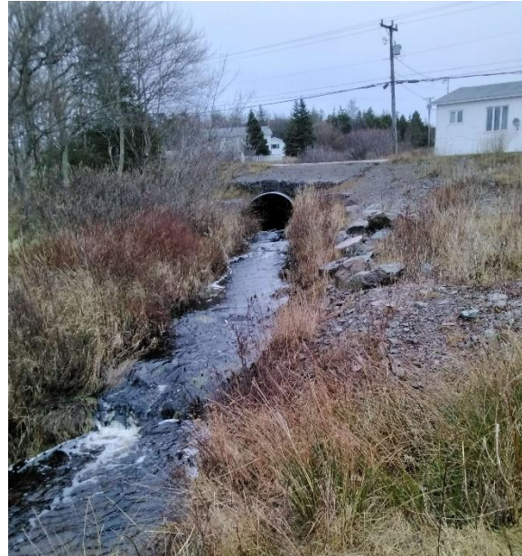
Photo 2: Downstream End of Structure
