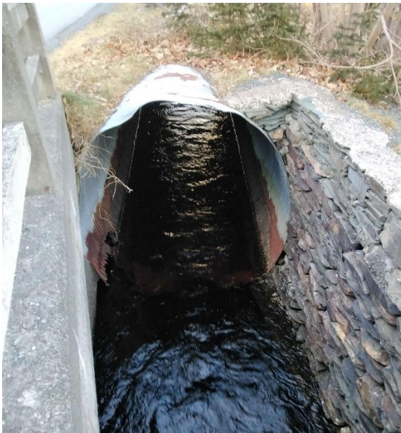
Photo 1: Upstream End of Structure
