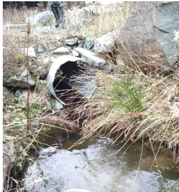
Photo 2: Downstream End of Structure
