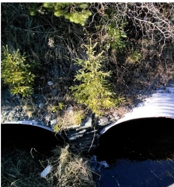
Photo 3: Looking Upstream from Structure
