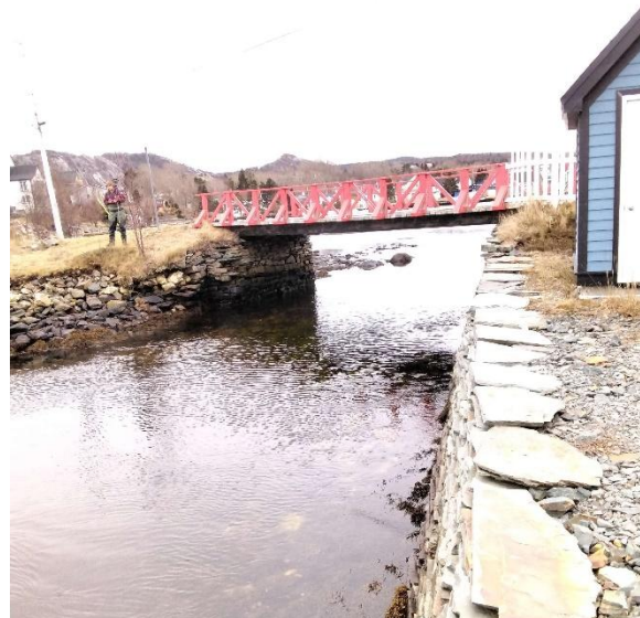
Photo 2: Downstream End of Structure
