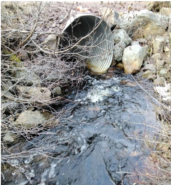
Photo 1: Upstream End of Structure
