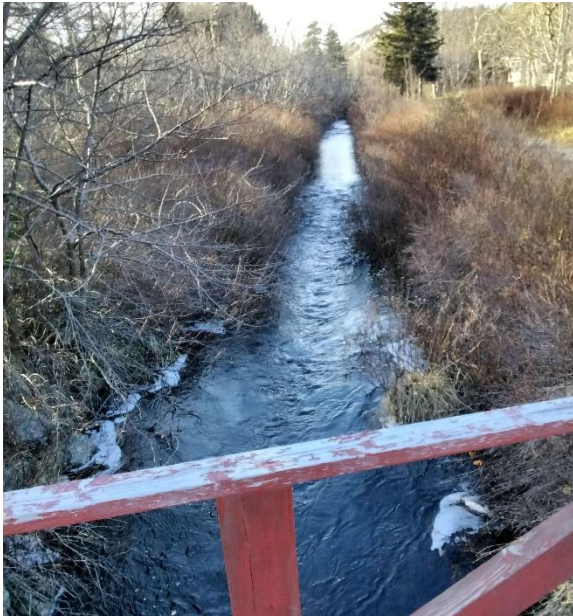
Photo 3: Looking Upstream from Structure
