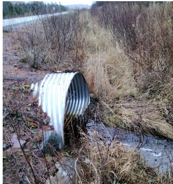
Photo 2: Downstream End of Structure
