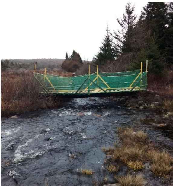
Photo 1: Upstream End of Structure
