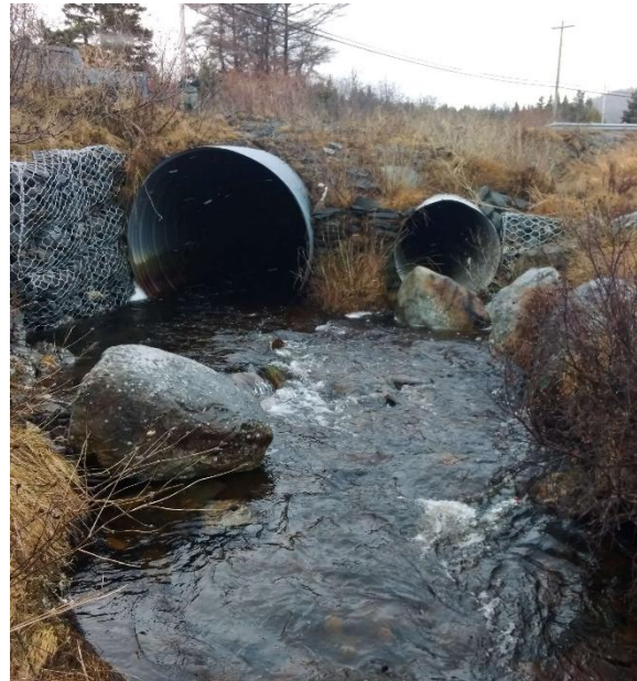
Photo 2: Downstream End of Structure
