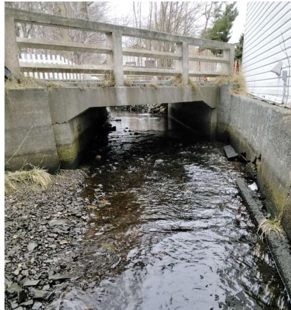
Photo 2: Downstream End of Structure
