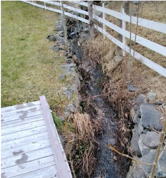
Photo 3: Looking Upstream from Structure
