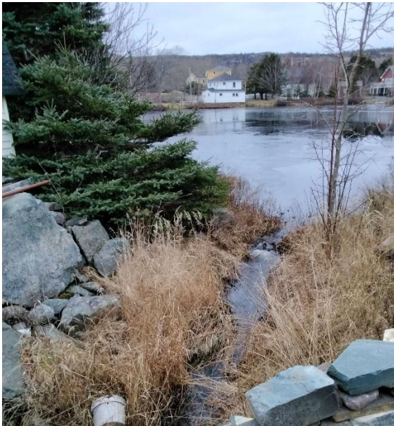
Photo 3: Looking Upstream from Structure
