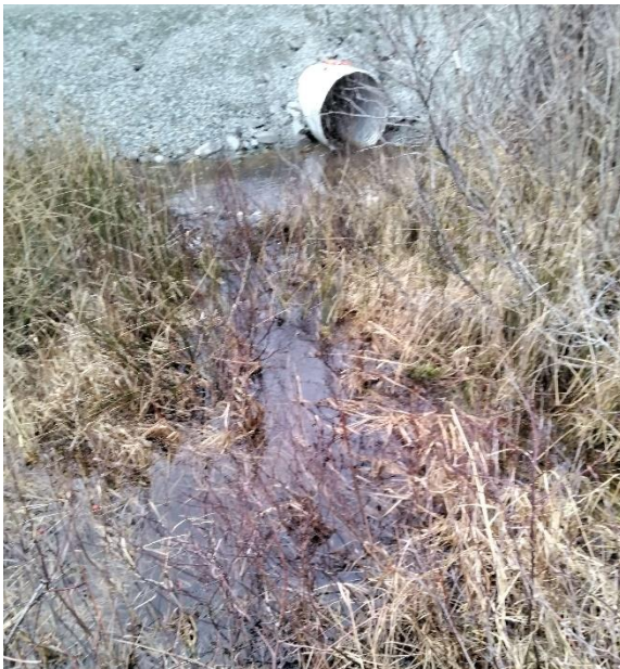
Photo 1: Upstream End of Structure
