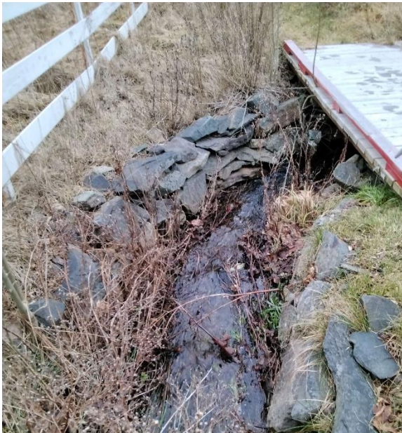
Photo 1: Upstream End of Structure
