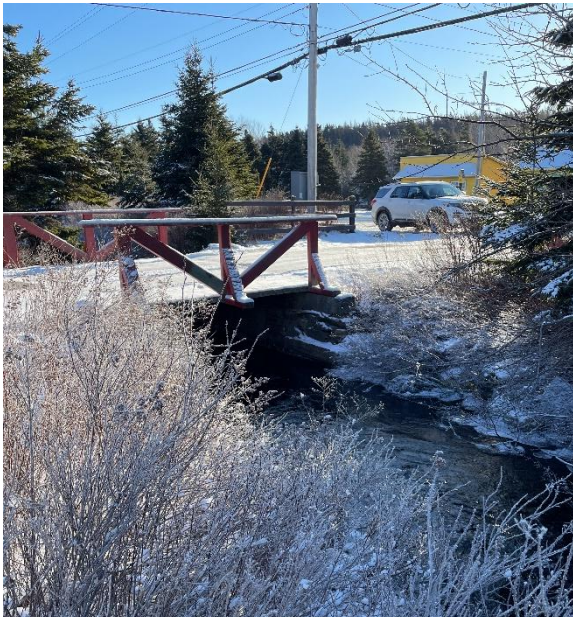
Photo 1: Upstream End of Structure
