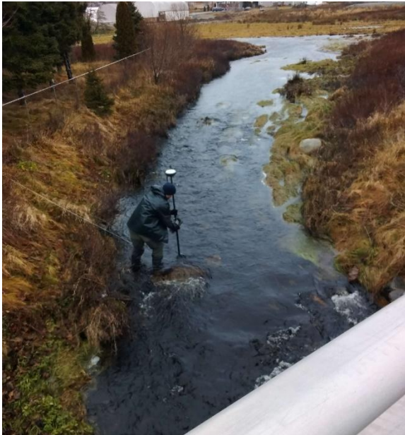
Photo 3: Looking Upstream from Structure
