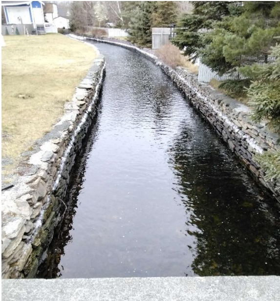
Photo 3: Looking Upstream from Structure
