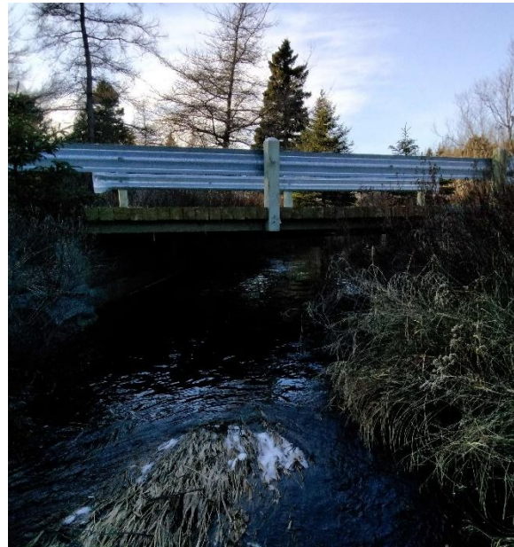
Photo 2: Downstream End of Structure
