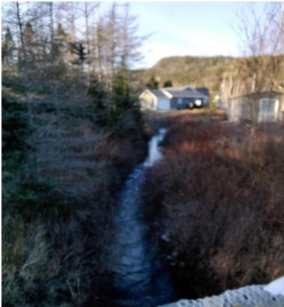
Photo 3: Looking Upstream from Structure
