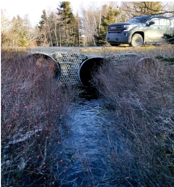
Photo 1: Upstream End of Structure
