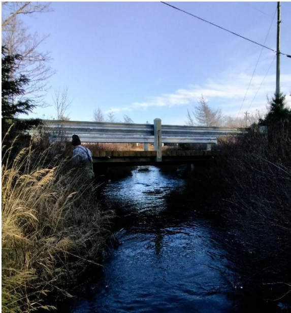
Photo 1: Upstream End of Structure
