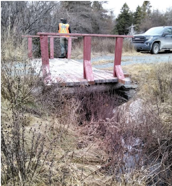
Photo 1: Upstream End of Structure
