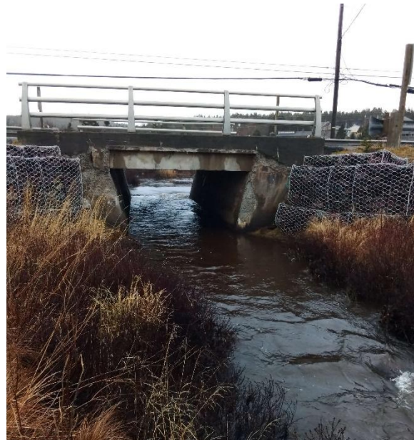
Photo 2: Downstream End of Structure
