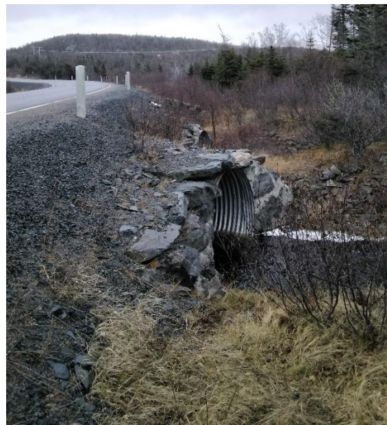
Photo 6: Side profile of Upstream End of Structure
