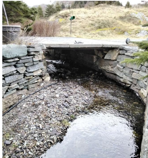
Photo 2: Downstream End of Structure
