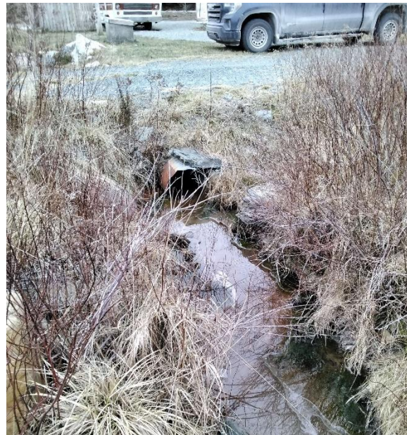
Photo 2: Downstream End of Structure
