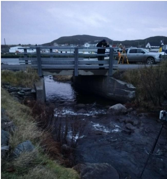
Photo 1: Upstream End of Structure
