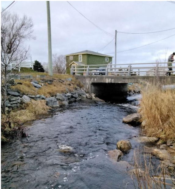
Photo 1: Upstream End of Structure
