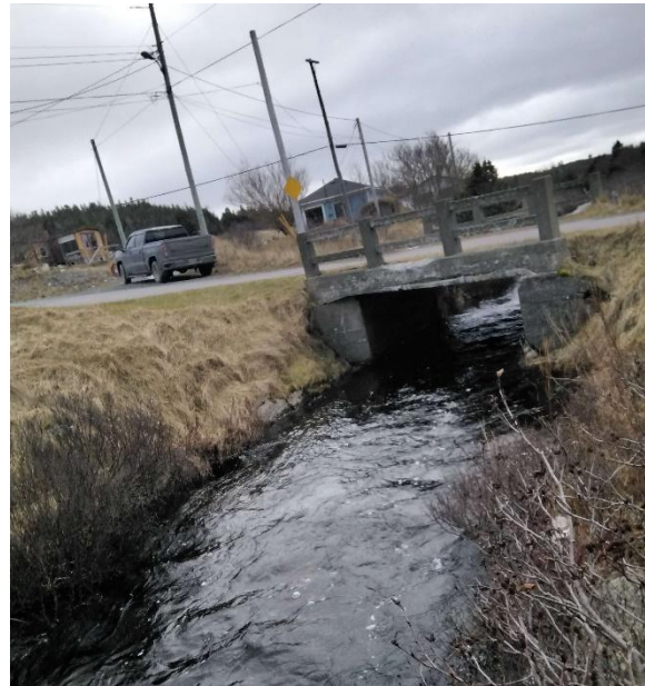
Photo 2: Downstream End of Structure
