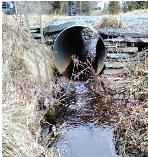
Photo 2: Downstream End of Structure
