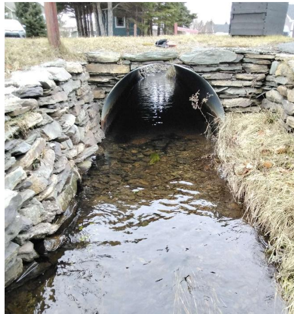
Photo 2: Downstream End of Structure
