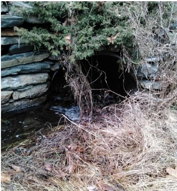
Photo 1: Upstream End of Structure
