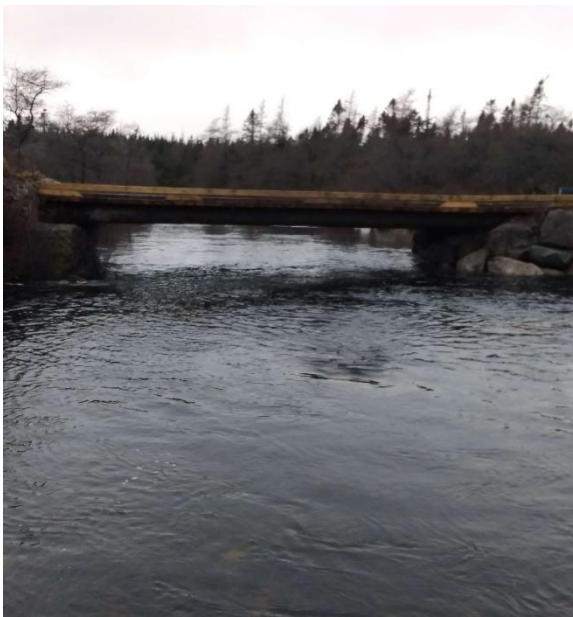
Photo 1: Upstream End of Structure
