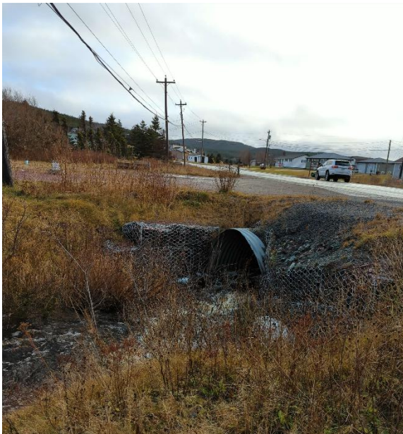
Photo 1: Upstream End of Structure
