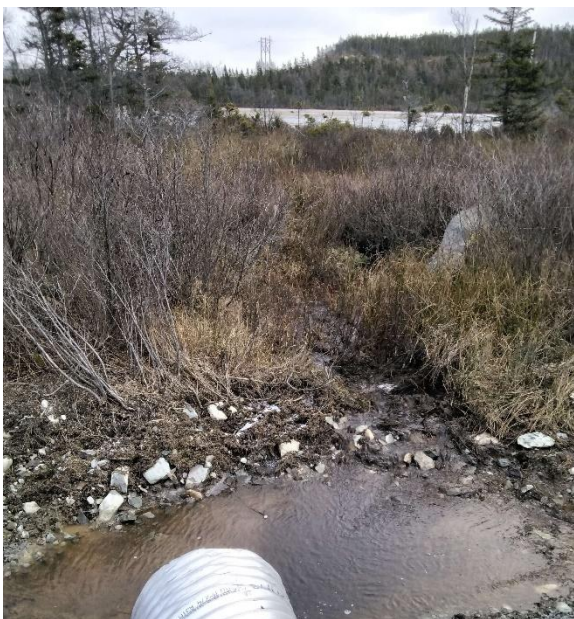
Photo 3: Looking Upstream from Structure
