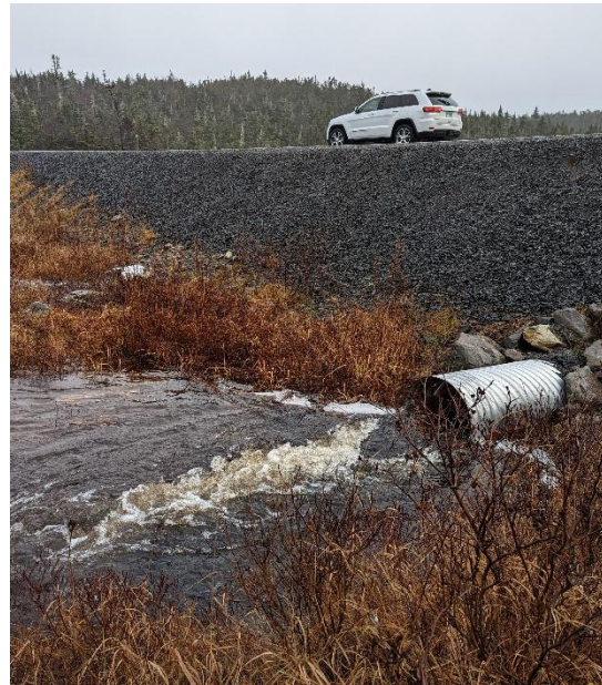
Photo 2: Downstream End of Structure
