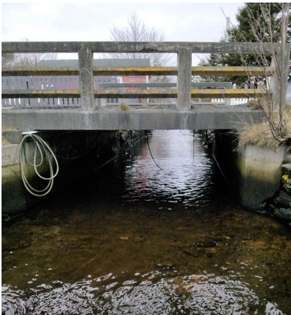
Photo 1: Upstream End of Structure
