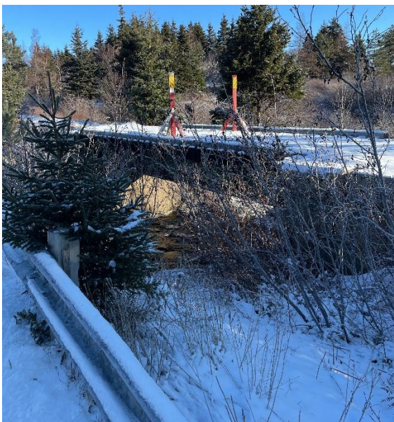
Photo 5: Upstream End of Structure 2
