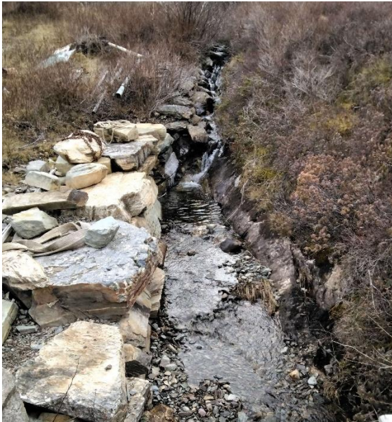
Photo 3: Looking Upstream from Structure
