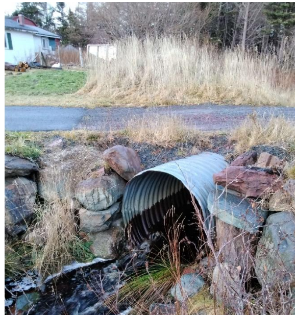
Photo 2: Downstream End of Structure
