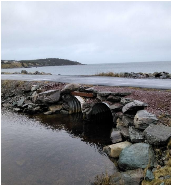
Photo 1: Upstream End of Structure
