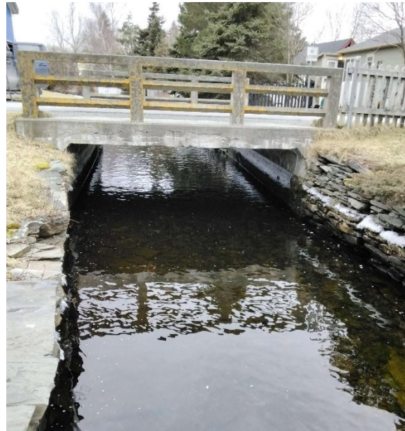
Photo 2: Downstream End of Structure
