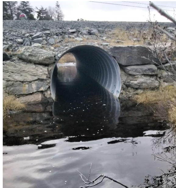
Photo 2: Downstream End of Structure
