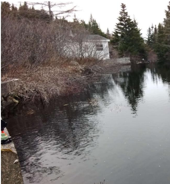
Photo 1: Upstream End of Structure
