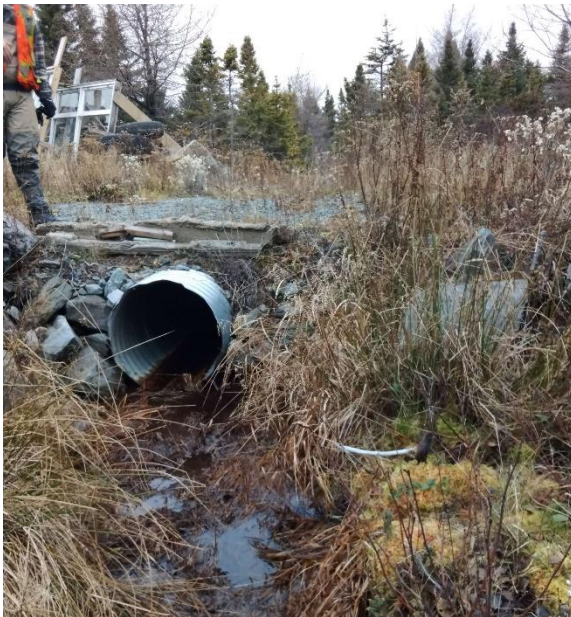
Photo 1: Upstream End of Structure
