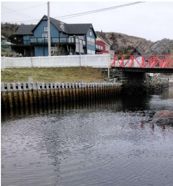
Photo 1: Upstream End of Structure
