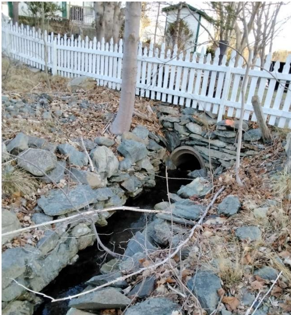
Photo 1: Upstream End of Structure
