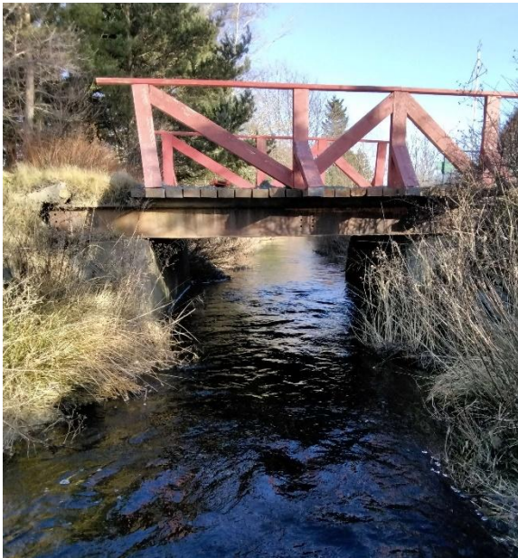
Photo 1: Upstream End of Structure
