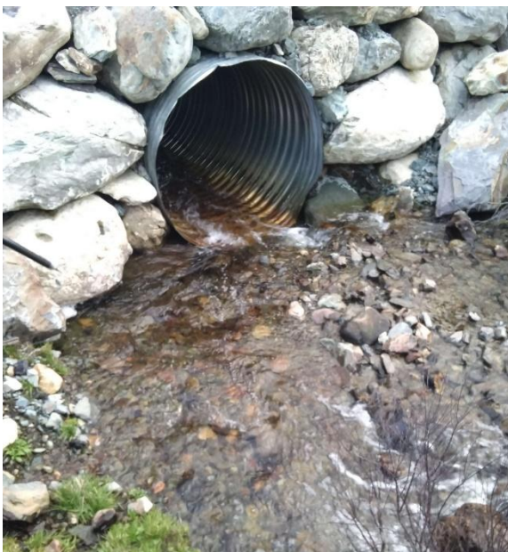
Photo 1: Upstream End of Structure
