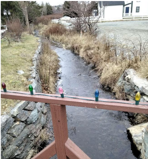
Photo 3: Looking Upstream from Structure
