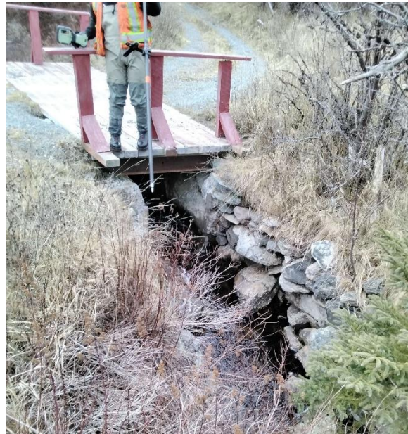
Photo 2: Downstream End of Structure
