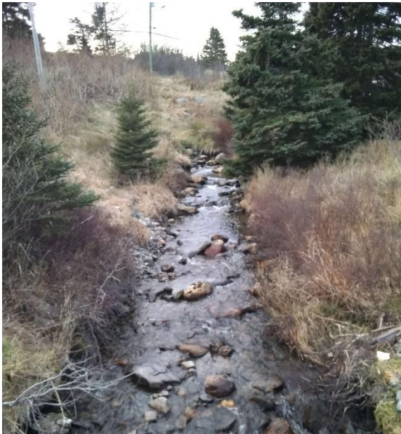
Photo 3: Looking Upstream from Structure
