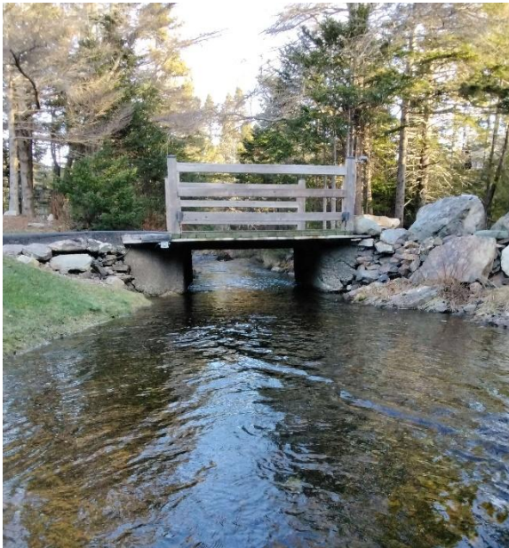
Photo 1: Upstream End of Structure
