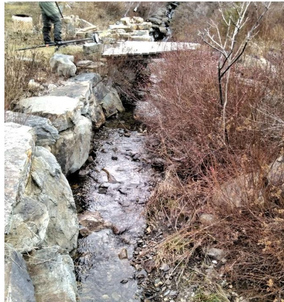
Photo 2: Downstream End of Structure
