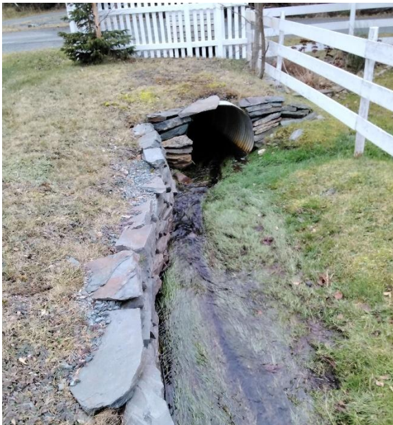
Photo 1: Upstream End of Structure
