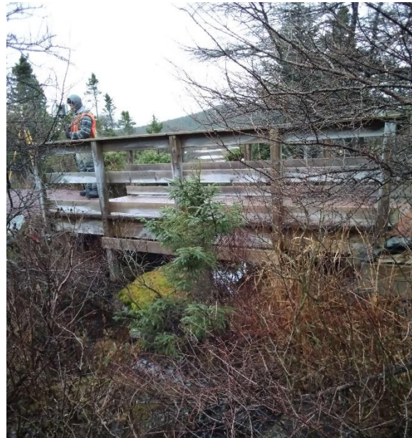
Photo 2: Downstream End of Structure
