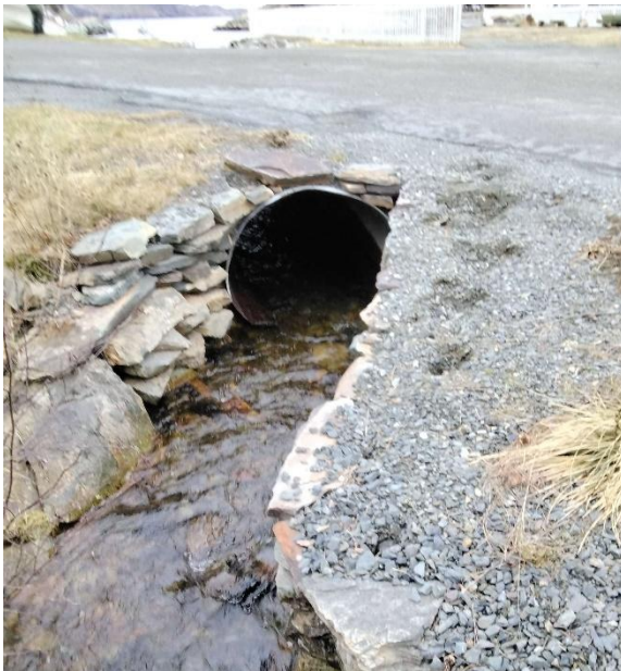
Photo 1: Upstream End of Structure
