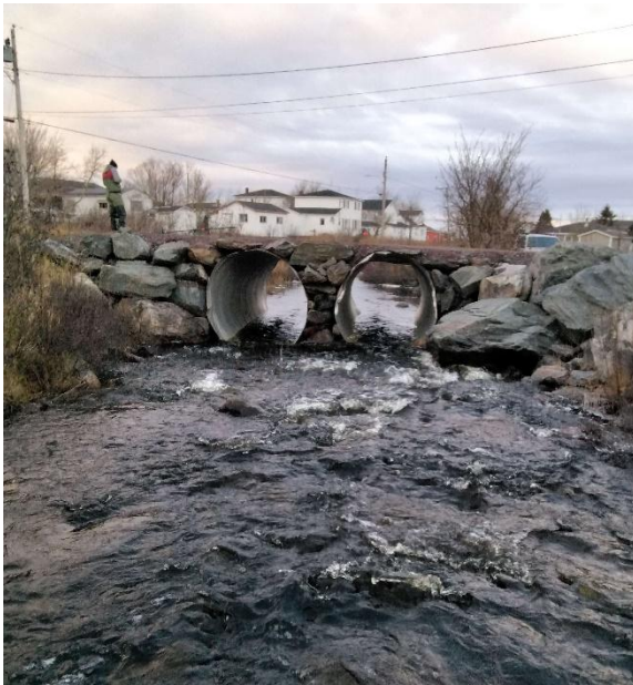
Photo 1: Upstream End of Structure
