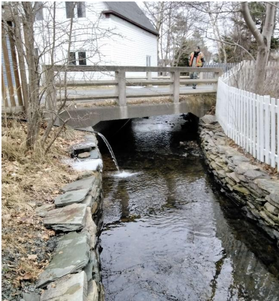
Photo 1: Upstream End of Structure
