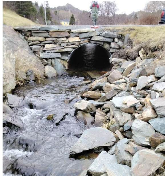
Photo 2: Downstream End of Structure
