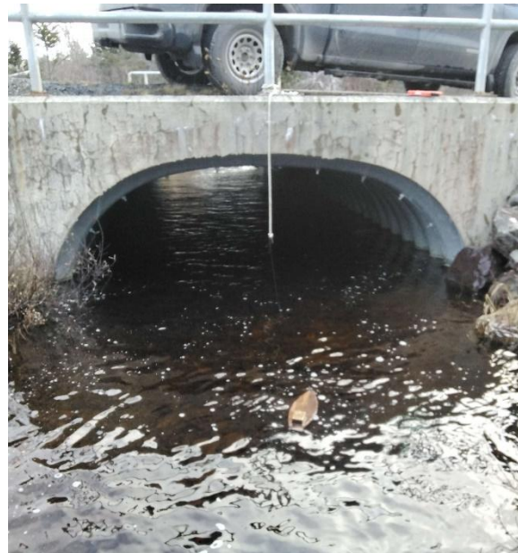
Photo 2: Downstream End of Structure
