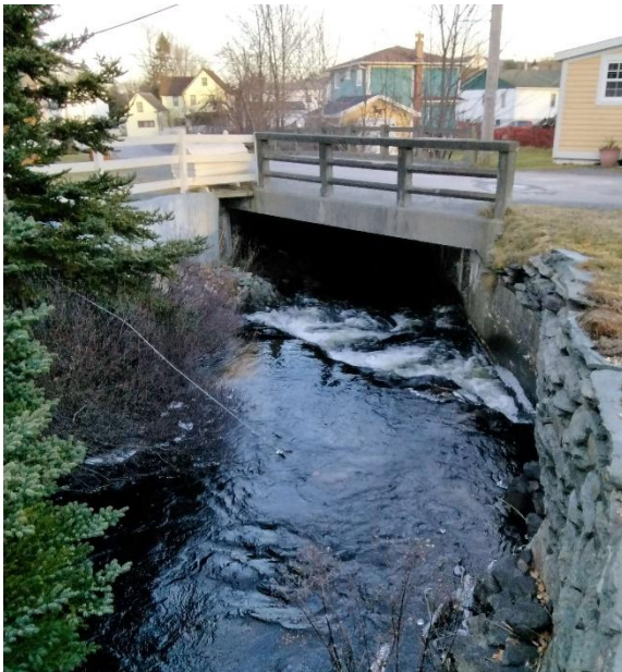
Photo 1: Upstream End of Structure
