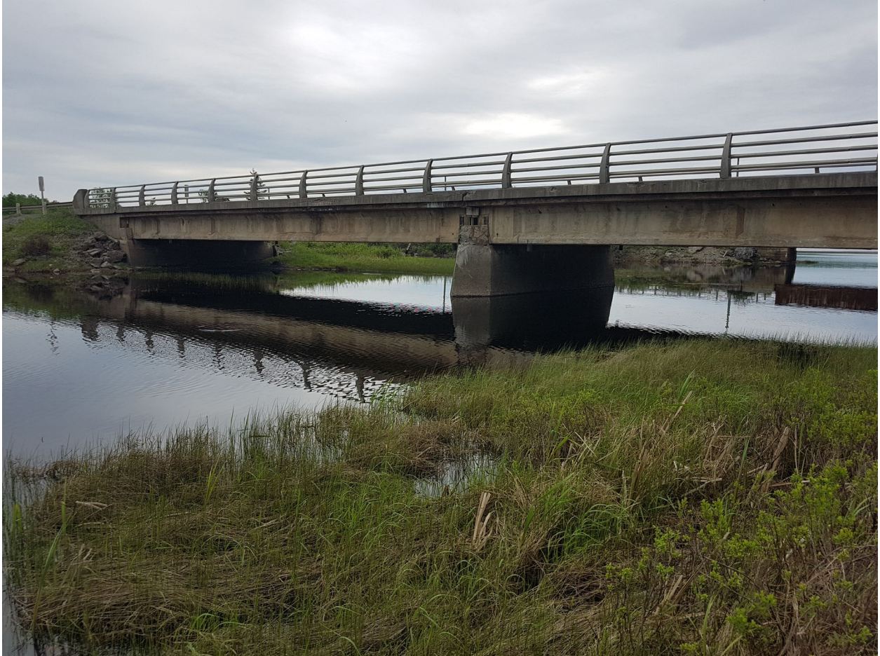
Photo 2: Upstream looking West
