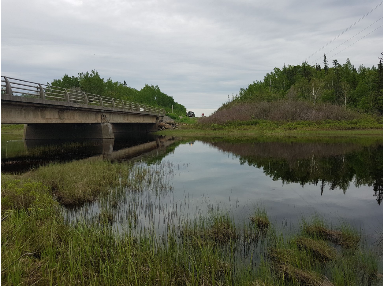
Photo 1: Upstream looking East
