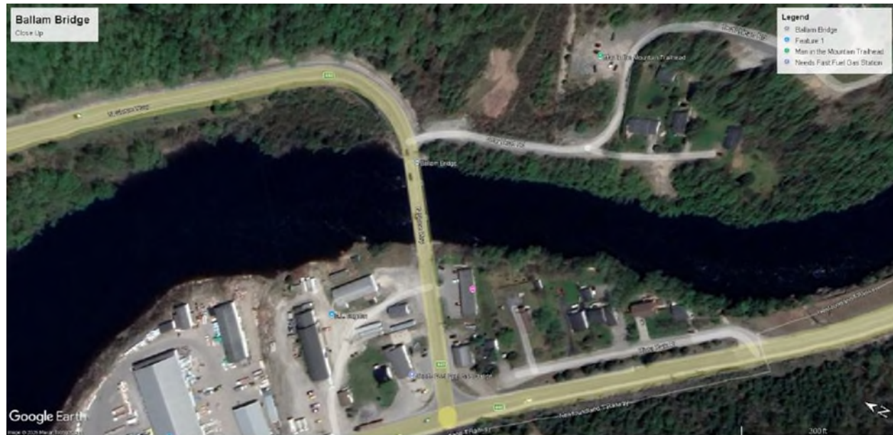
Google Earth Image 4: Close-up of Bridge Site
