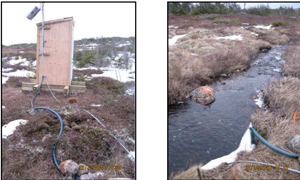
Figure 2: Real-Time Water Quality and Quantity Station at Outflow of Unnamed Pond south of Long Pond. Station hut (left) and instrument deployed in brook (right).
