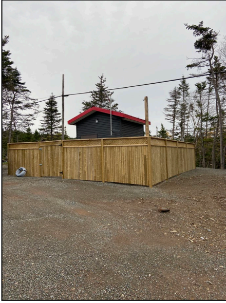
Figure 2: Hut Structure for groundwater well
