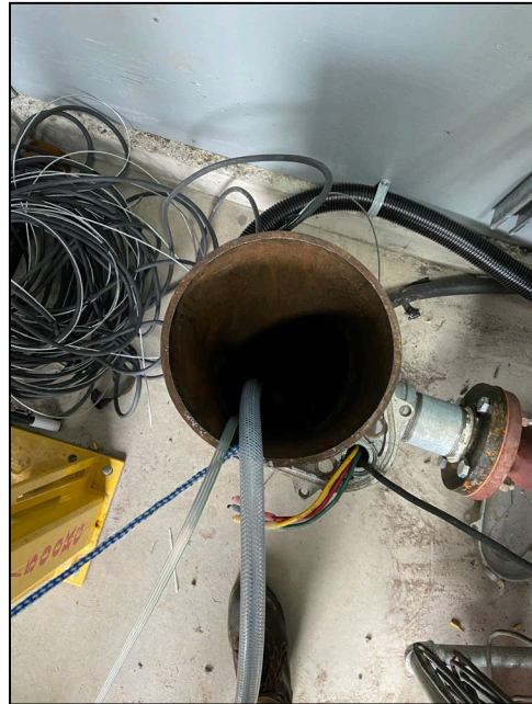
Figure 5: View looking into well
