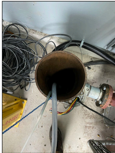
Figure 5: View looking into well
