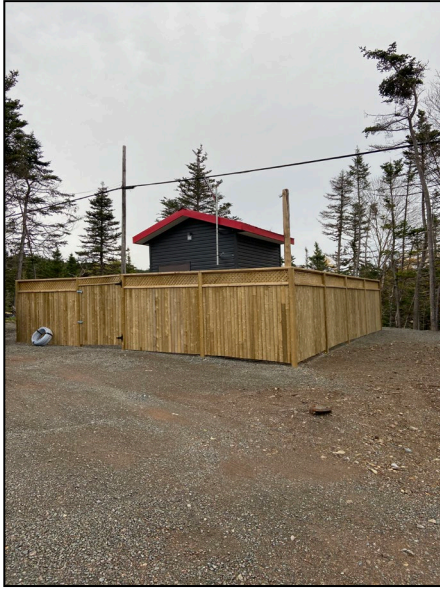
Figure 2: Hut Structure for groundwater well
