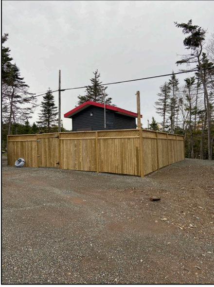
Figure 2: Hut Structure for groundwater well
