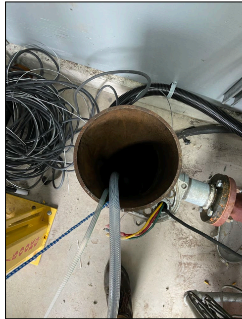
Figure 5: View looking into well
