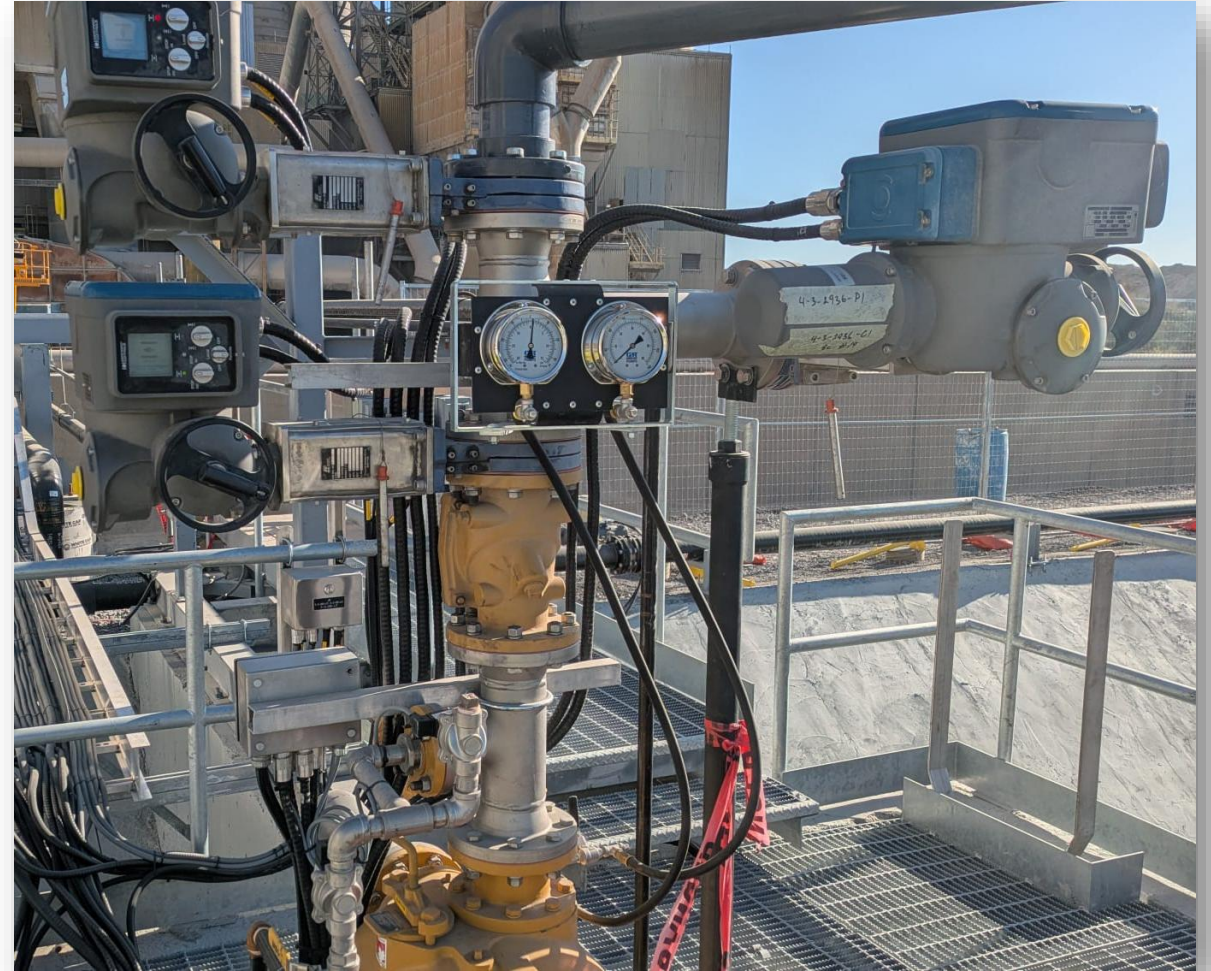
CASE STUDY: BT Series on Knife Gate Valves at St. Mary's Cement, Bowmanville ON
