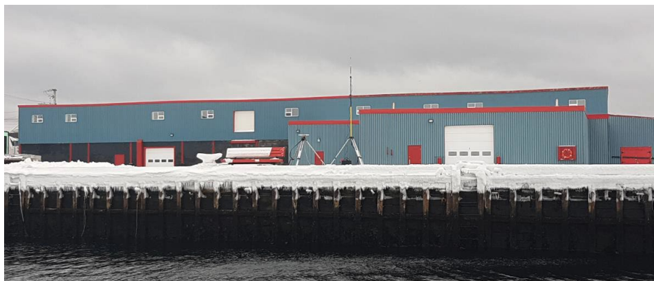
Figure 3.3.2 – Station de base GPS RTK Trimble installée sur le CSR1945 BS1f.
