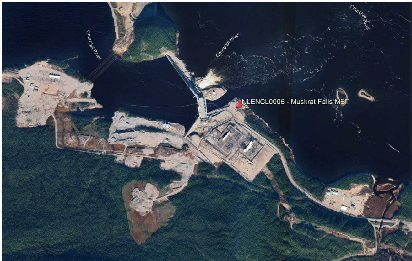
Figure 5: Muskrat Falls Weather Station Location
