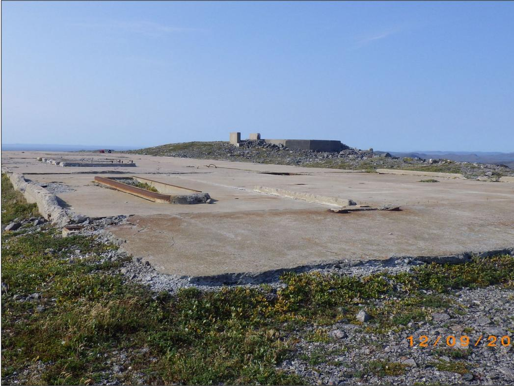
PHOTO 95 - APEC #10: Concrete slab of former main building foundation. Soil is exposed in various location within the slab. (September, 2017)
