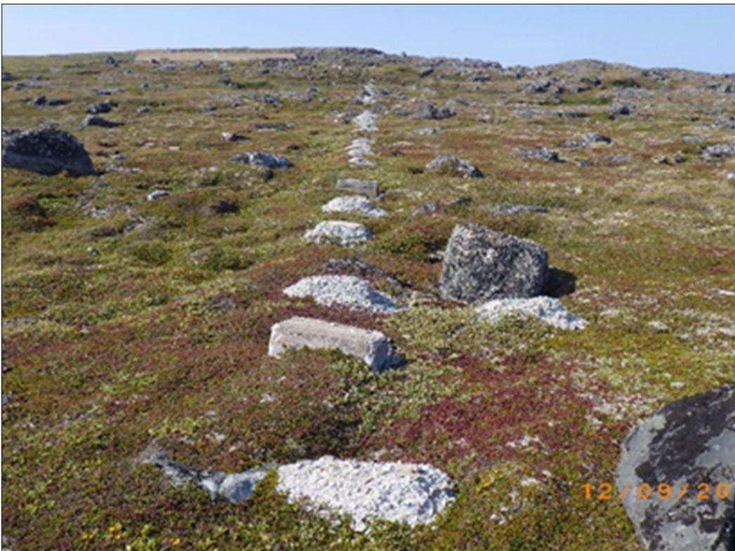
PHOTO 70 - APEC #8: View of concrete blocks used to support water piping uphill. (September, 2017)
