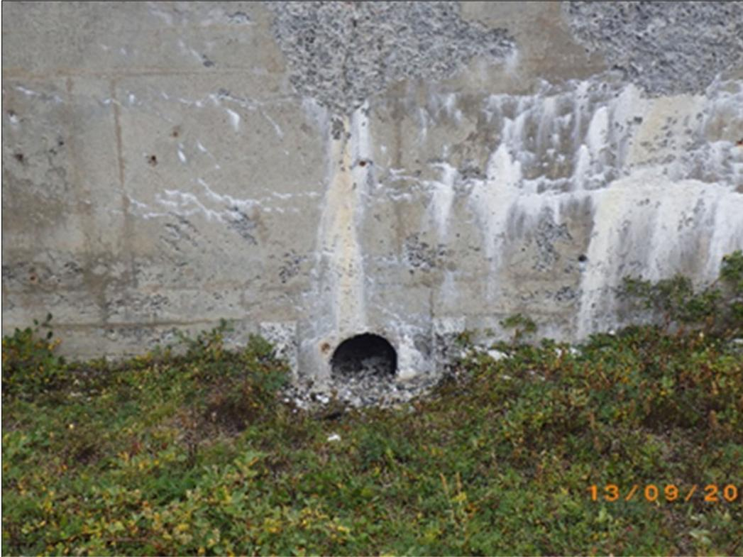
PHOTO 19 - APEC #2: View of pipe, likely for draining water through the concrete berm. (September, 2017)
