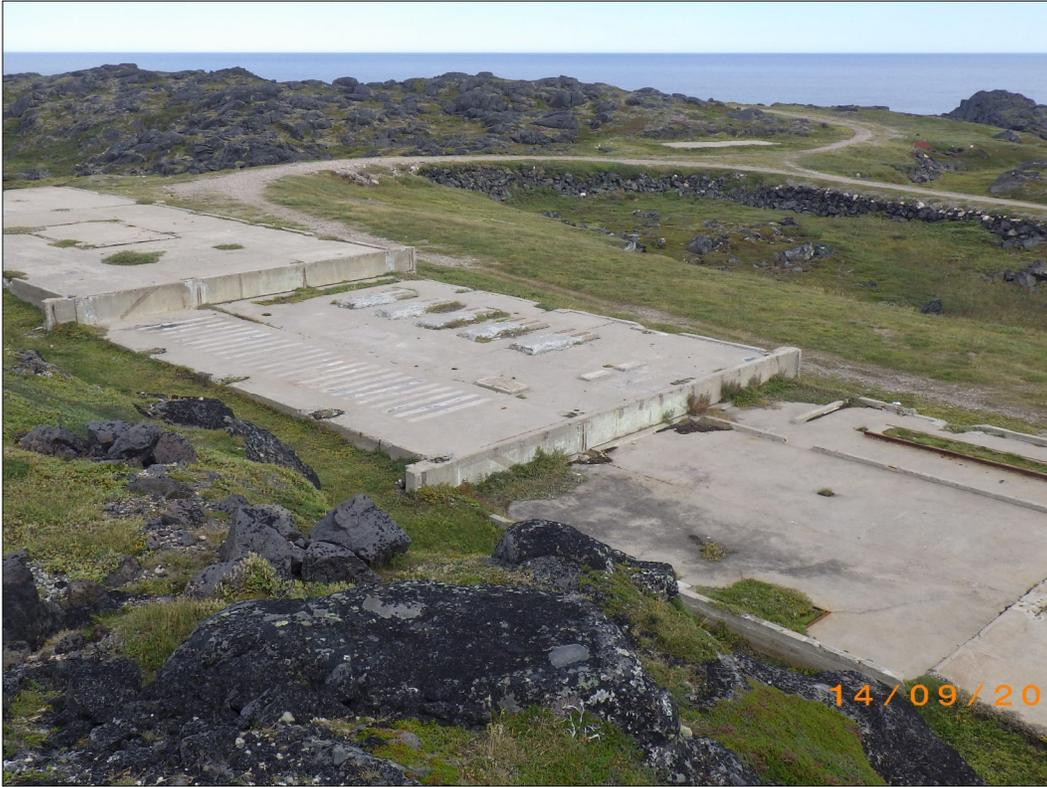
PHOTO 25 - APEC #5: Main building showing step foundation. (September, 2017)
