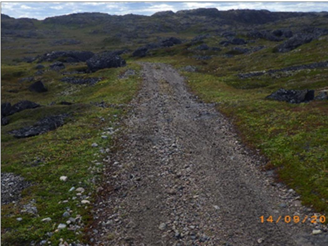
PHOTO 50 - APEC #7: Gravel access road that connects the Upper Site to the Lower Site, still in good condition. (September, 2017)
