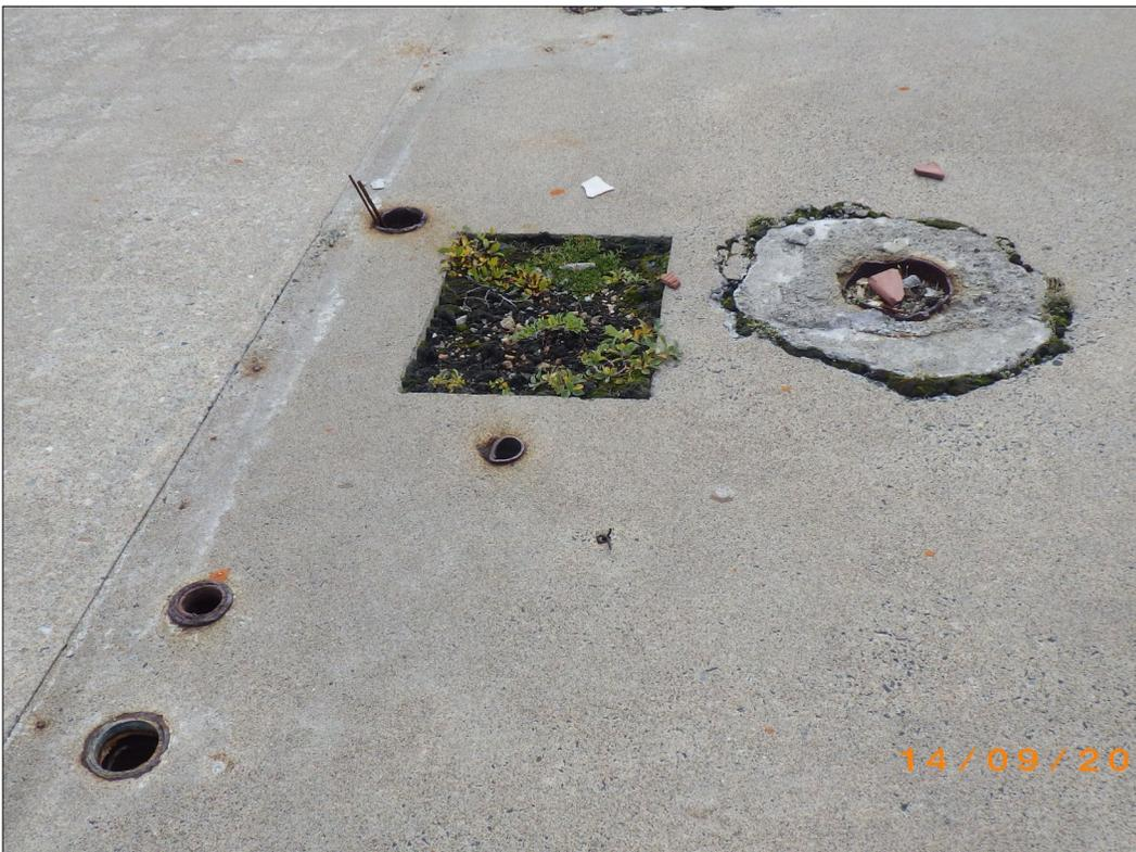
PHOTO 26 - APEC #5: View of penetrations through the slab of the Main building. Metal fittings presumed to be lead-containing. (September, 2017)
