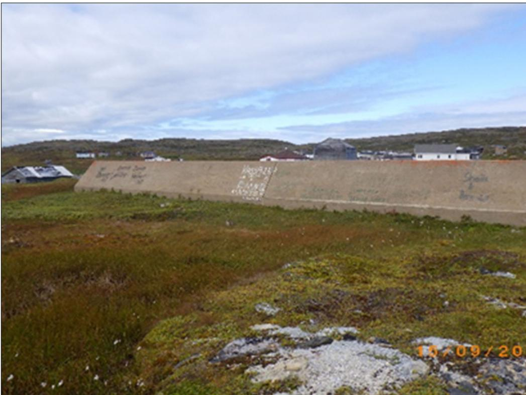
PHOTO 86— APEC #12: Concrete berm around former AST location at the Lower Site.
