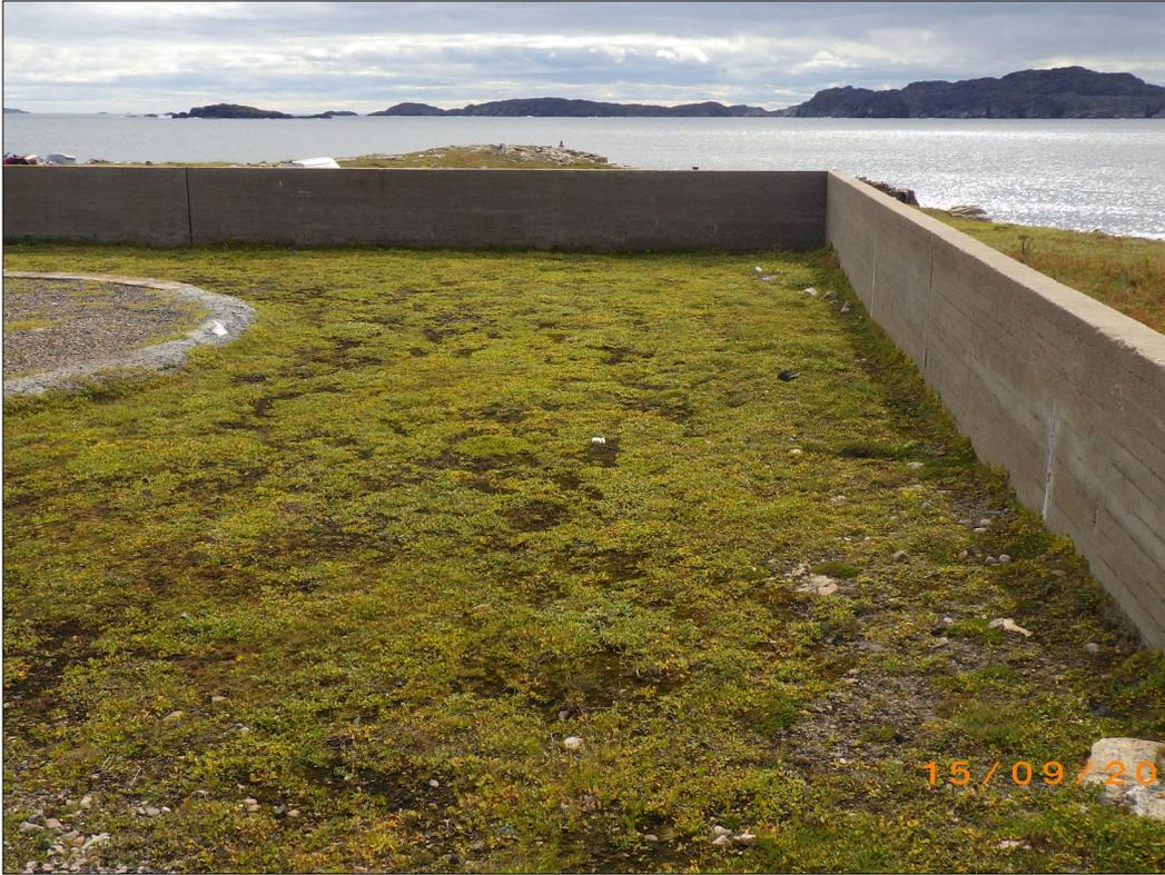
PHOTO 85— APEC #12: Pad and berm surrounding former AST at the Lower Site.
