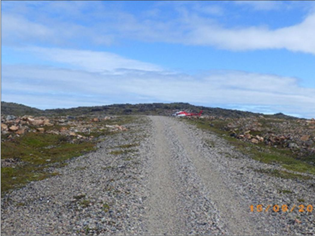
PHOTO 51 – APEC #7: Gravel access road that connects the Upper Site to the lower Site, still in good condition. (September, 2017)
