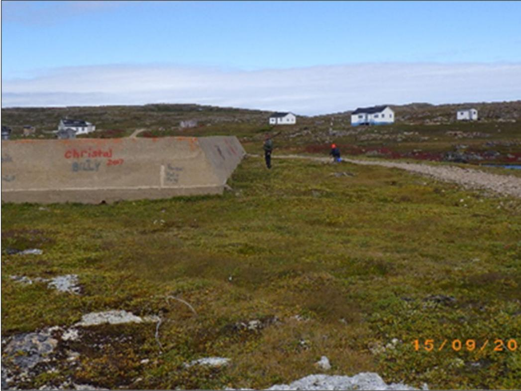
PHOTO 87– APEC #12: Concrete berm around former AST location at the Lower Site, with the gravel access road to the right. (September, 2017)
