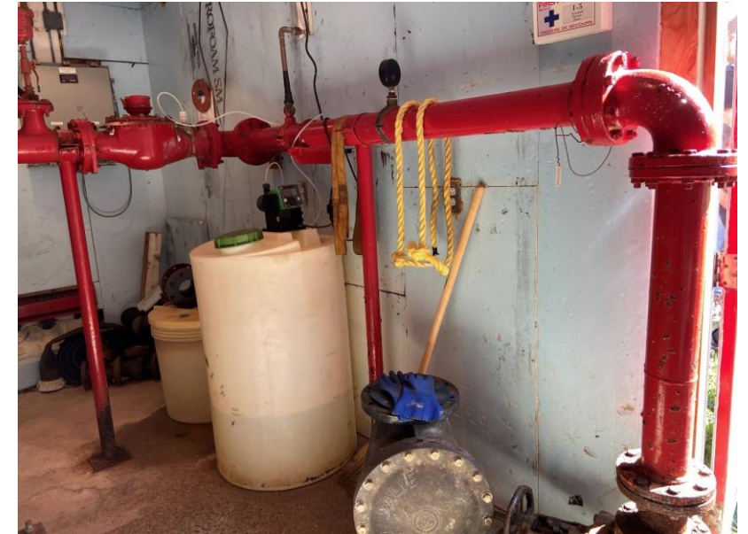
Above; disinfection equipment Fixed speed pump (~4 L/s) to standpipe
