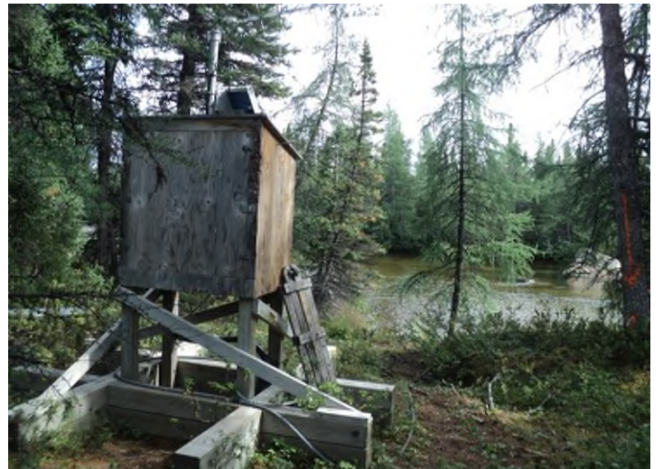
Figure 18: RTWQ hut at Reid Brook below Tributary
