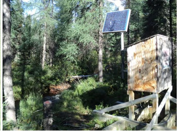
Figure 13: RTWQ hut at Tributary to Reid Brook
