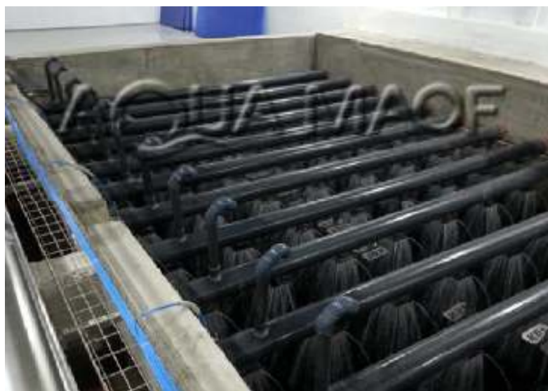
Biofilter spray nozzles distributing water over media of the trickling filter in a trout production facility. Note the air blower for CO 2 degassing at middle left side of biofilter. Multiple blower fans supply water to an air space below the media stack. Technicians adjusting the controls for water flow to the biofilter nozzles. View of the tube settler on the far right that supplies water to the nozzles with gravity flow.
