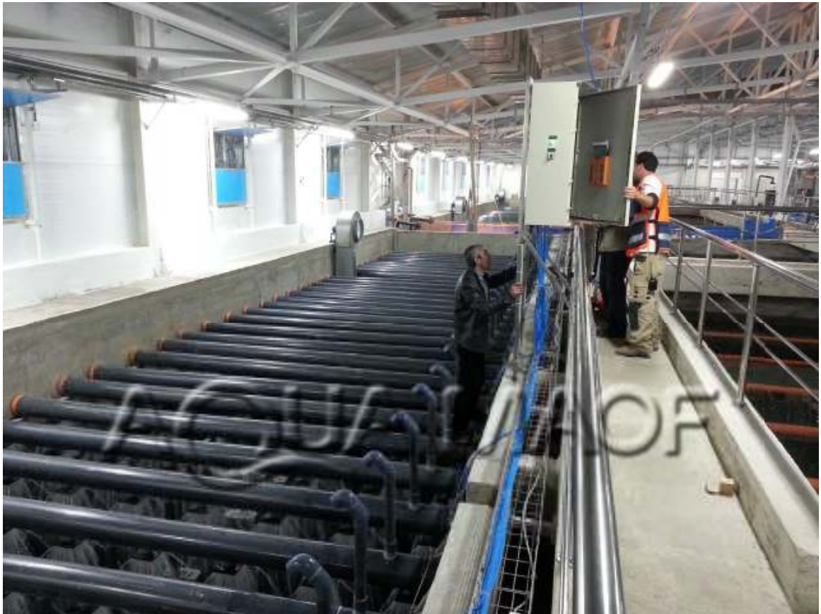
Biofilter spray nozzles distributing water over media of the trickling filter in a trout production facility. Note the air blower for CO 2 degassing at middle left side of biofilter. Multiple blower fans supply water to an air space below the media stack. Technicians adjusting the controls for water flow to the biofilter nozzles. View of the tube settler on the far right that supplies water to the nozzles with gravity flow.
