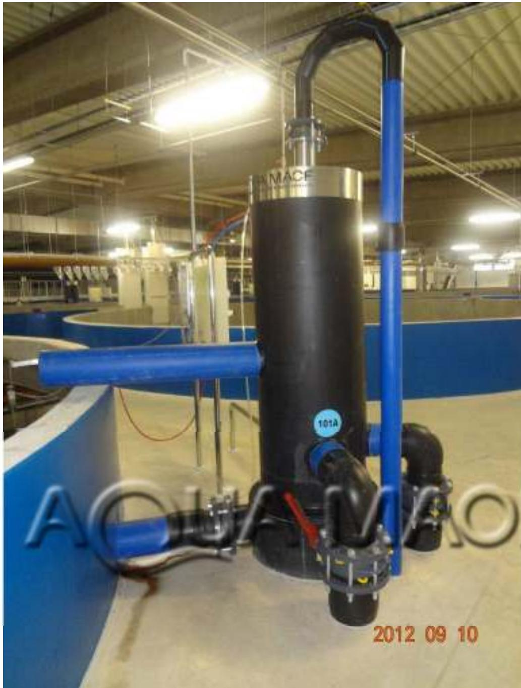
AquaMaof oxygen dissolving system (ODS) showing duplicate water supply from the pipes on lower portion. The duplicate water supply pipes are connected separately to duplicate water pumps. The pipe extending to the top is for adding new water as required. Oxygenated water flows from the ODS through the tank sidewall. The pipe extending from the ODS over the tank sidewall is an overflow pipe.
