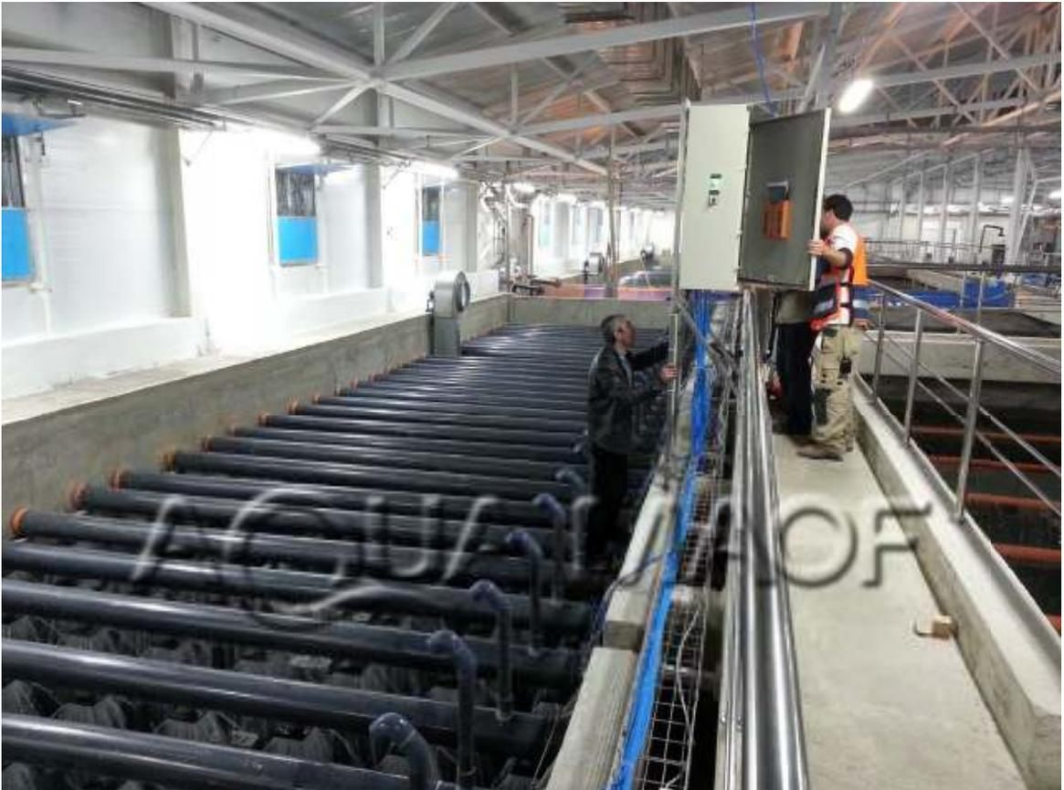
Biofilter spray nozzles distributing water over media of the trickling filter in a trout production facility. Note the air blower for CO<sub>2</sub> degassing at middle left side of biofilter. Multiple blower fans supply water to an air space below the media stack. Technicians adjusting the controls for water flow to the biofilter nozzles. View of the tube settler on the far right that supplies water to the nozzles with gravity flow.
