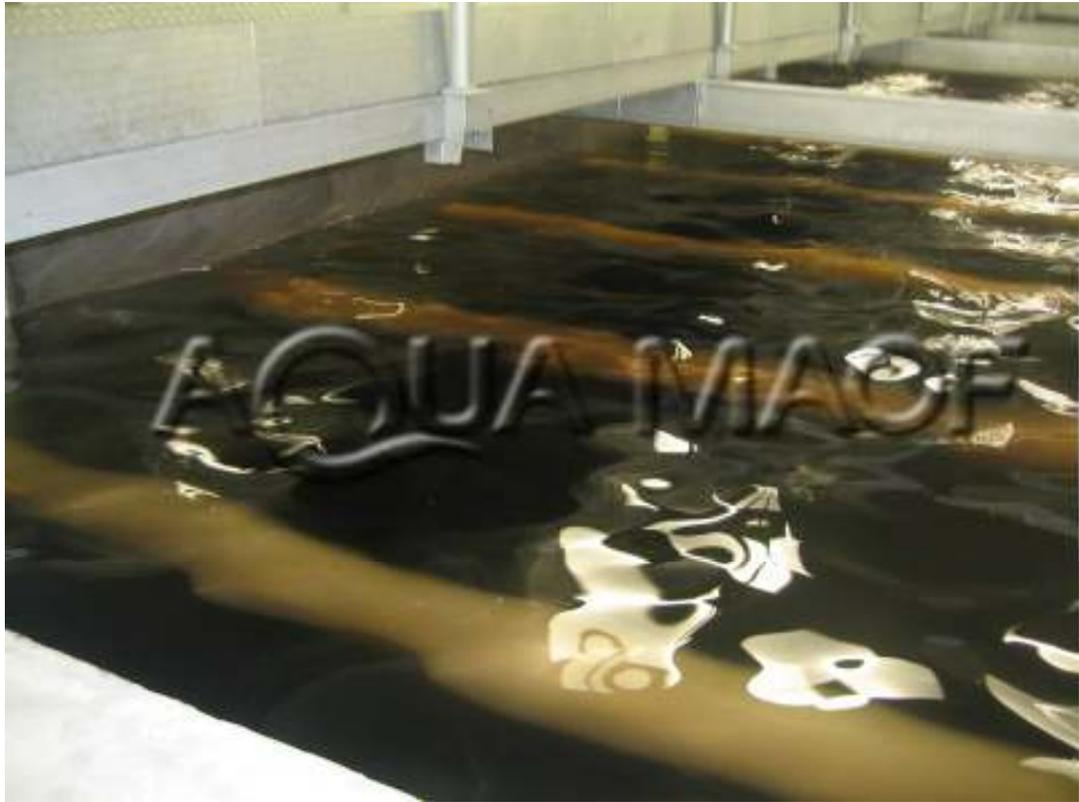
AquaMaof solid waste settler in operation. The pipes visible below the water surface are the water collection pipes distributing water to the biofilter spray nozzles. Water pressure for the spray nozzles is supplied by gravity flow.
