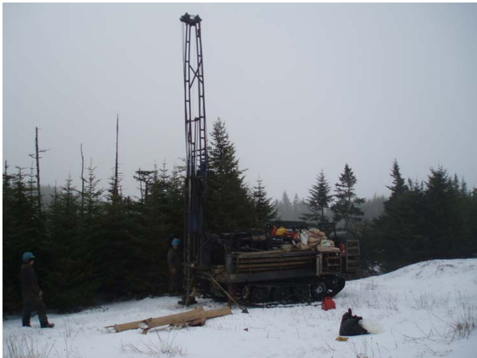
Photograph 4 –Preparing For Borehole Drilling
