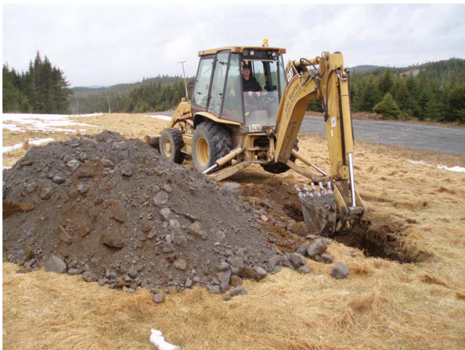
Photograph 2: Typical Test Pit
