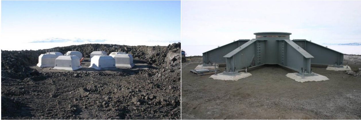
Figure 4-3 Antarctica Wind Turbine Foundations
