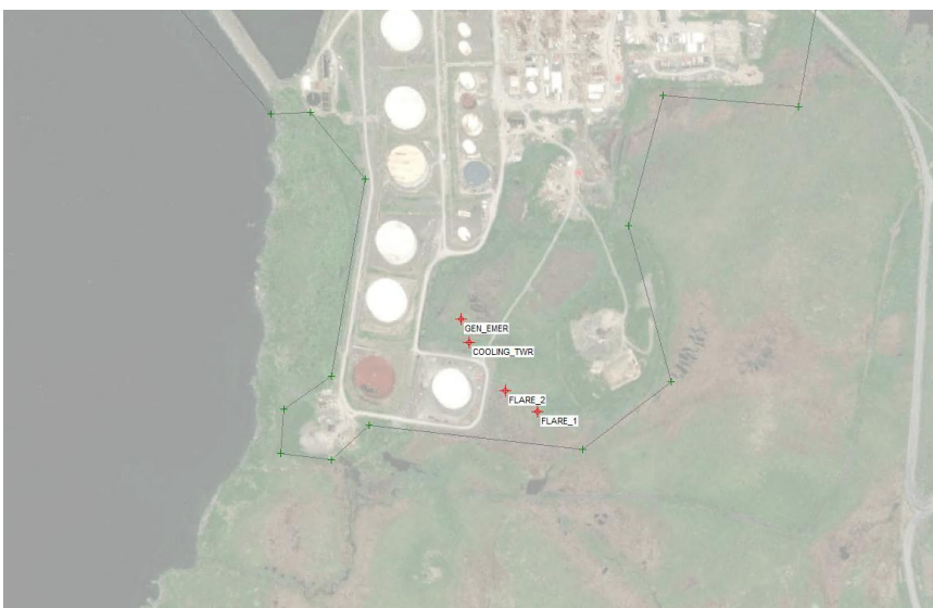
Figure 1 Approximate location of the cooling towers (labelled COOLING_TWR)
