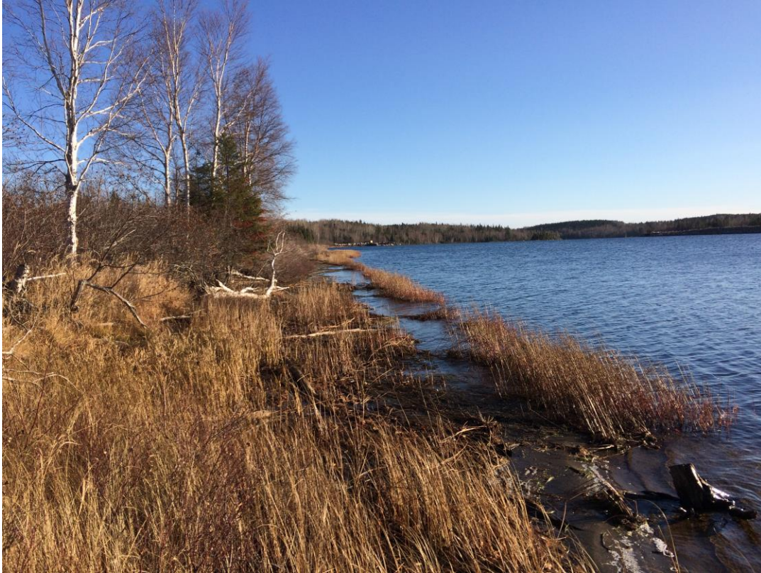
Figure 3.8. East View Toward Dam Showing Shoreline Fronting Areas 4 and 5 (note evidence of inundation)
