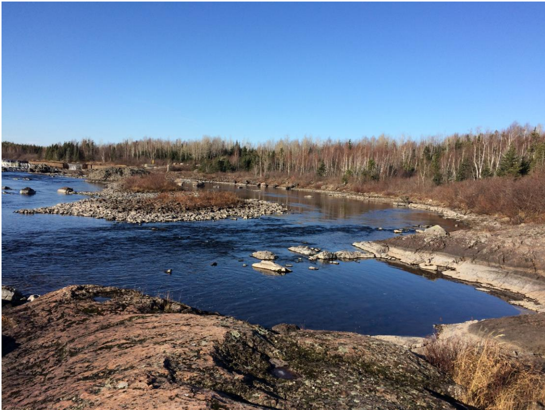
Figure 3.10. Northwest View of Area 5 Below the Dam (note rocky and steep shoreline)
