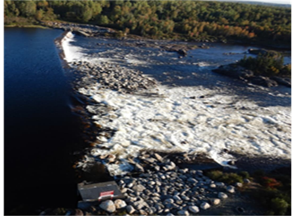
Repaired with large riprap
