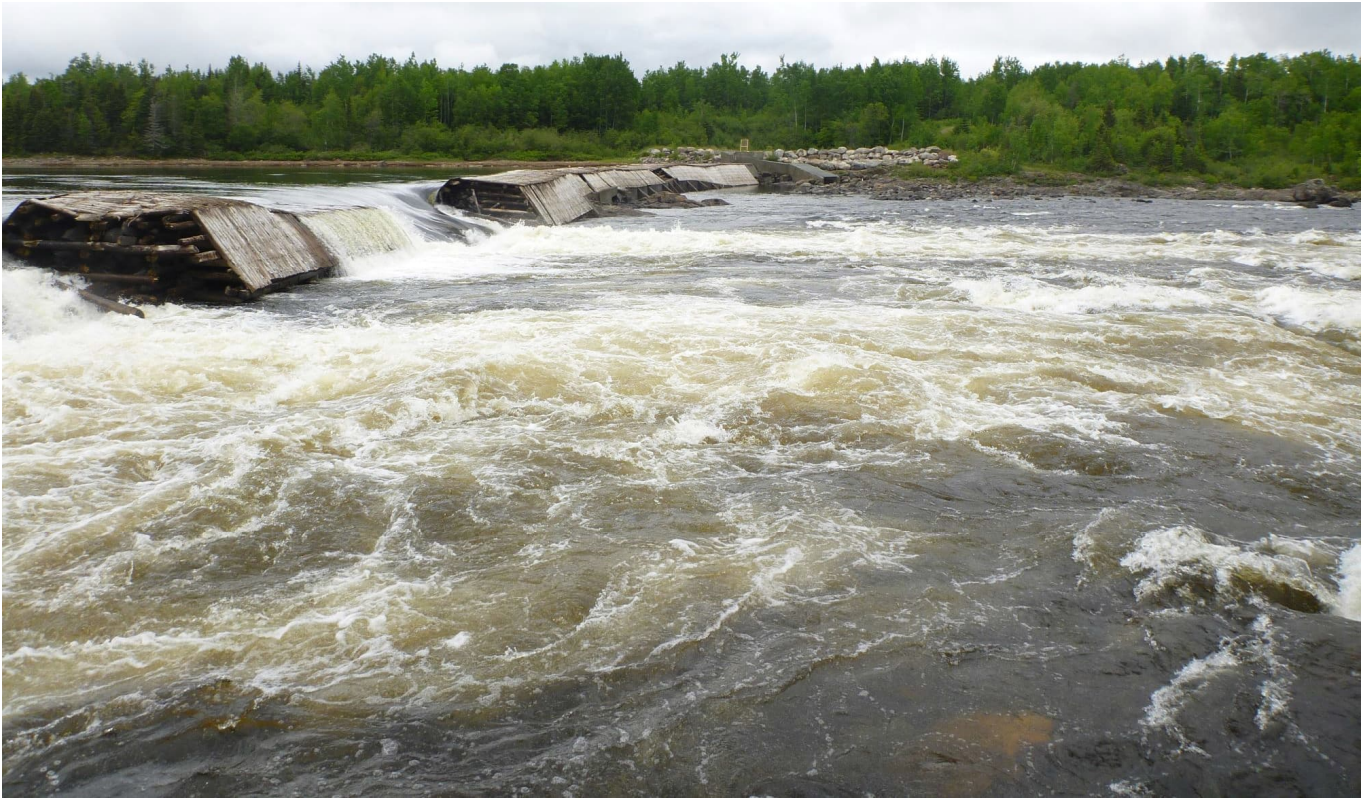
Figure 5-5: Image of Goodyears Dam (looking north) during 2015 breach (June 23, 2025) showing flows along the southern section
