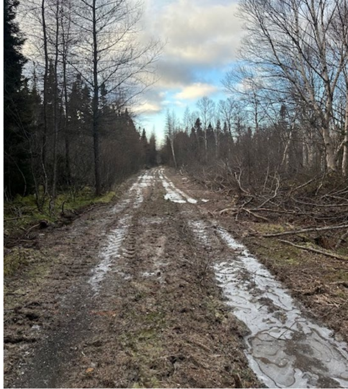
Figure 7 Site Access Road
