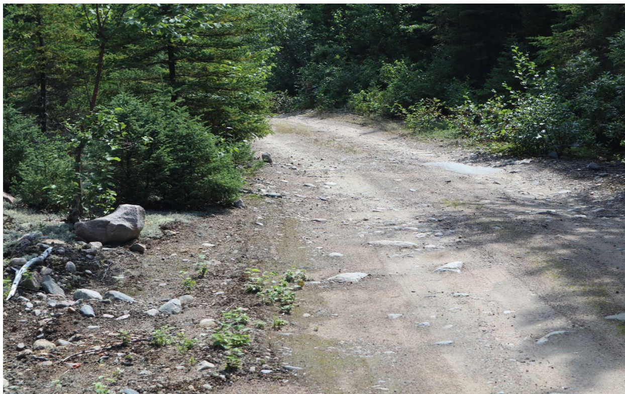
Photograph 1 - Existing Side Access Road
