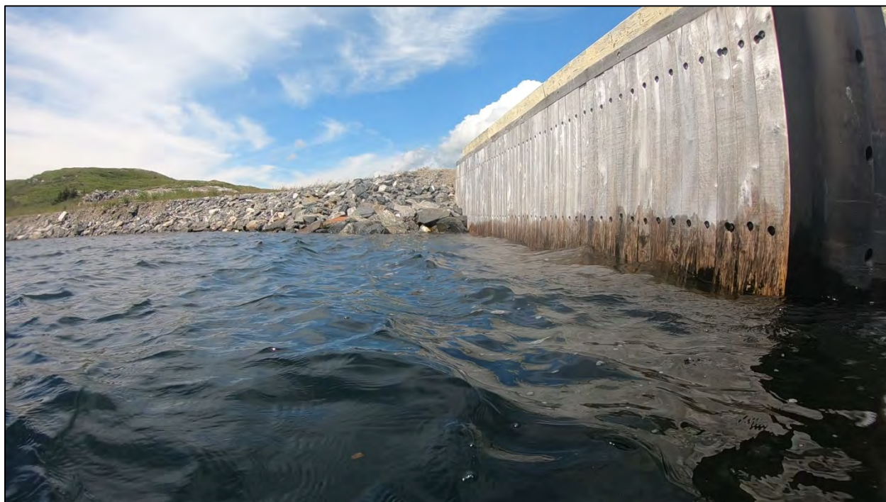
Photo 52: Wharf section and riprap shoreline in ST4
