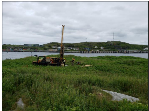
Photograph A: View of the drilling operations on the south side of the island.
