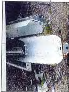
FLOURESCENT LIGHT FIXTURE CONTAINING PCB BALLASTS UNDER CAMP BUILDING #1
