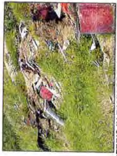
DEBRIS IN BANK OF DISPOSAL AREA, NOTE DRUM
