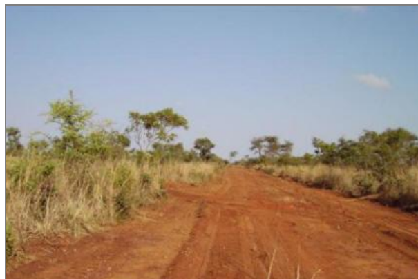
Figure 11-13 - Example of Grubbed and Cleared Path
