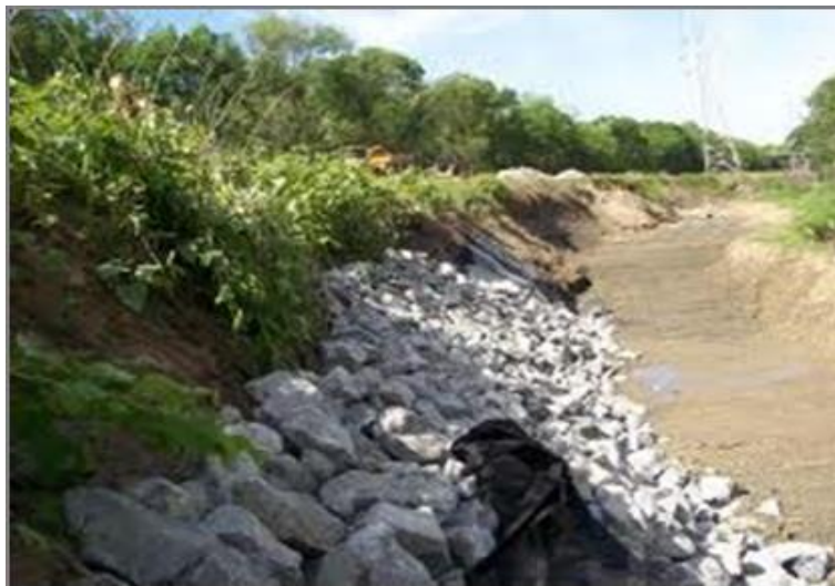
Figure 11-26 - Photograph of Rip Rap Placed Along a Slope
