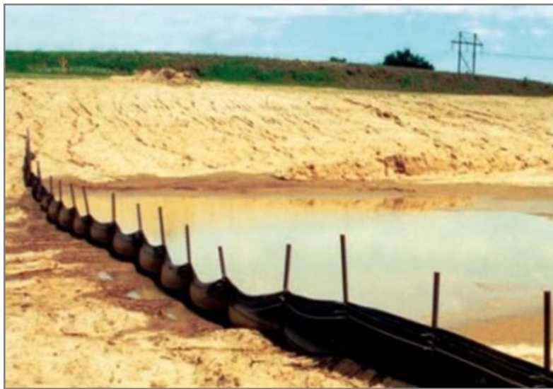
Figure 11-32 - A Well Constructed Silt Fence
