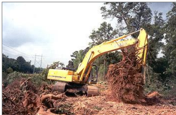
Figure 11-12 - Example of Grubbing Activities
