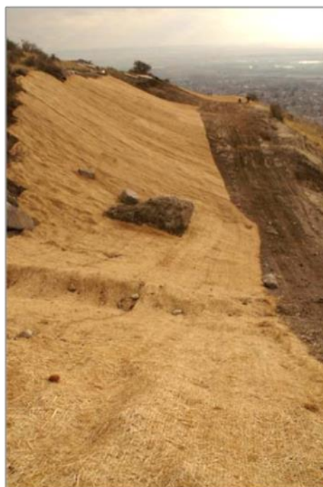
Figure 11-223 - Photograph of Erosion Control Blanket used on a Slope
