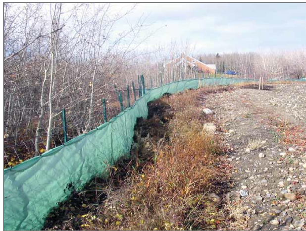
Figure 11-9 - Tarp Fence Outlining a Vegetation Buffer Zone
