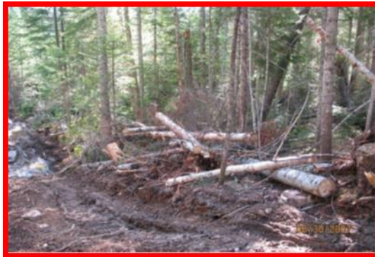
Figure 11-1 - Poorly Cut and Piled Wood
