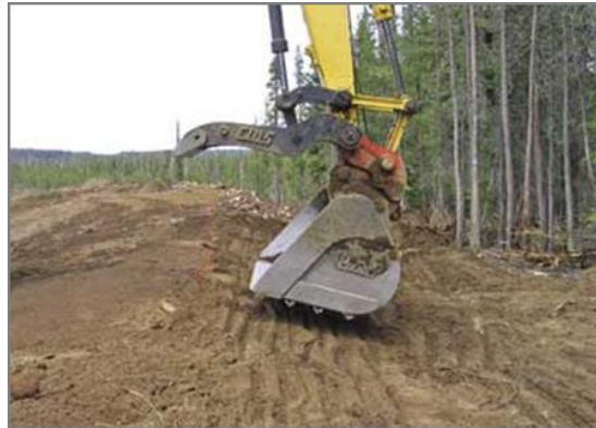
Figure 11-20 - Photograph of Grooving Slope Treatment Method
