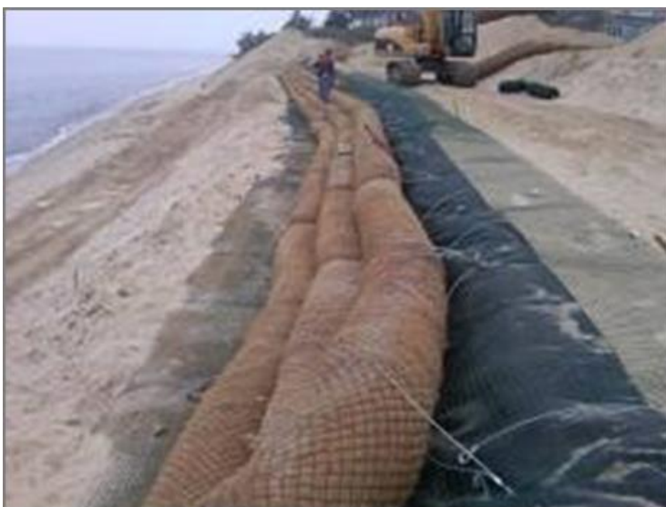
Figure 11-34 - Photograph of Fibre Rolls used to Stabilize
