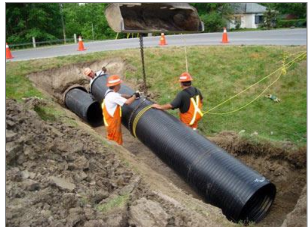
Figure 11-8 - Example of Culvert Installation
