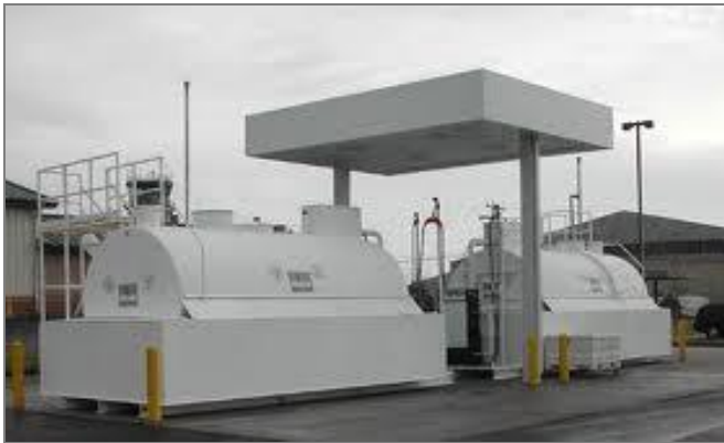
Figure 11-5 - Acceptable Fuel Storage with Dykes
