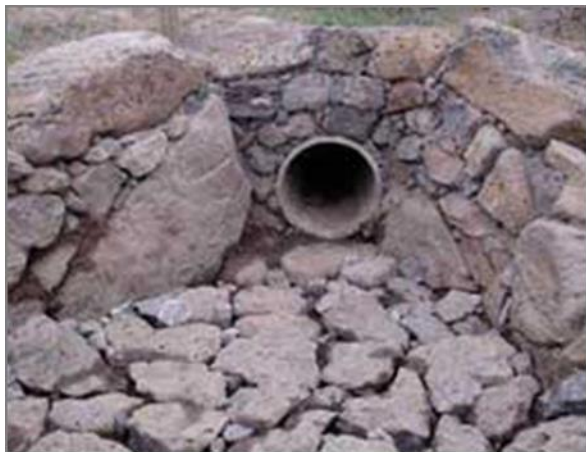
Figure 11-30 - Correct Construction of Rock Energy Dissipaters
