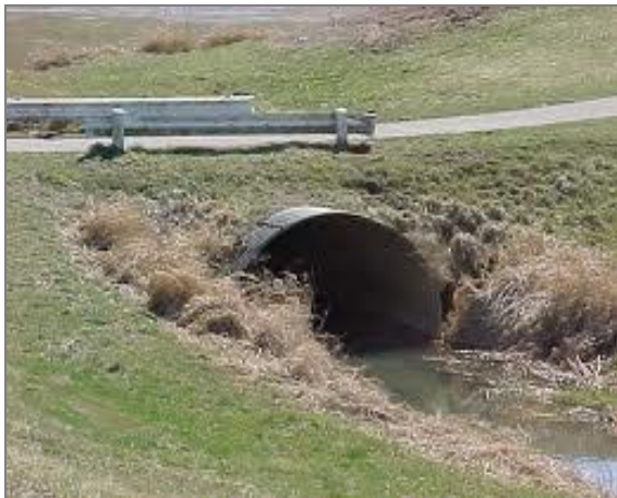
Figure 11-7 - Example of Well Installed Culvert
