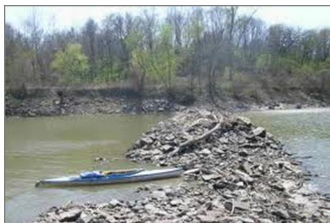
Figure 11-29 - Photograph of a Rock Constructed Dike
