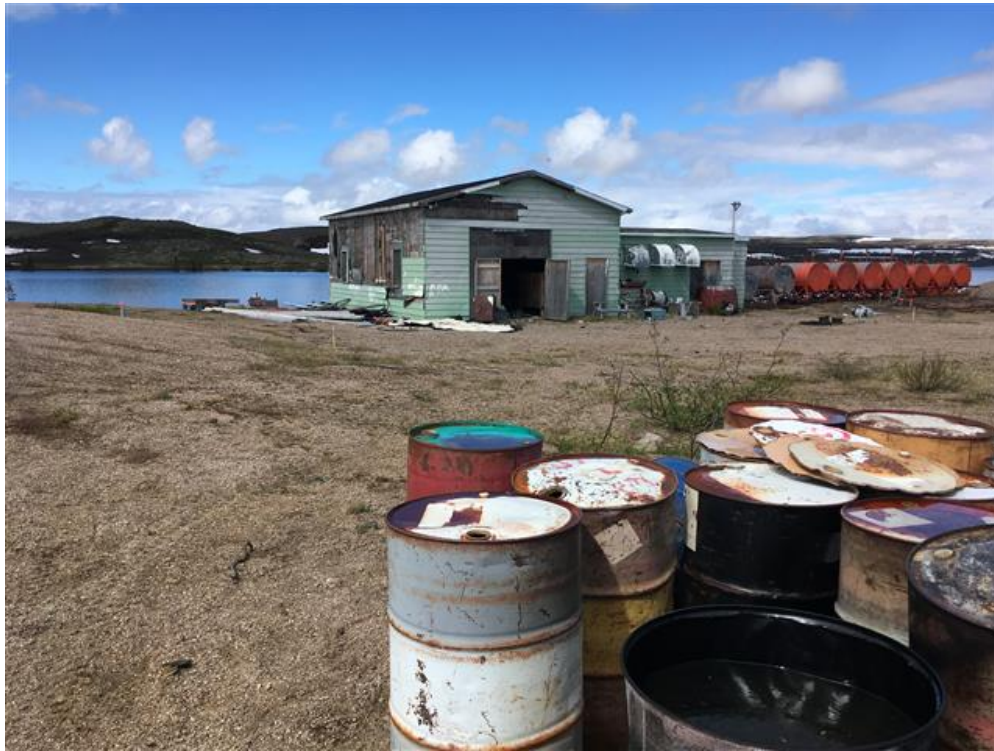
Photo 5 – Camp / Antenna Areas and AES Compound: Camp Garage Building with approximately 30 empty or partially filled drums on the south side of the structure (emptied and removed as part of the current assessment). Looking northeast.
