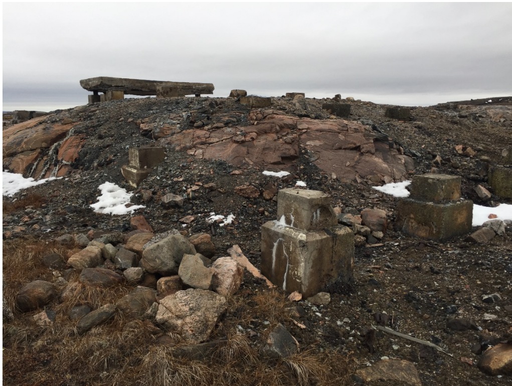
Photo 22 – Upper Site: concrete slab and pillars of Former Operations Building. Looking northwest.
