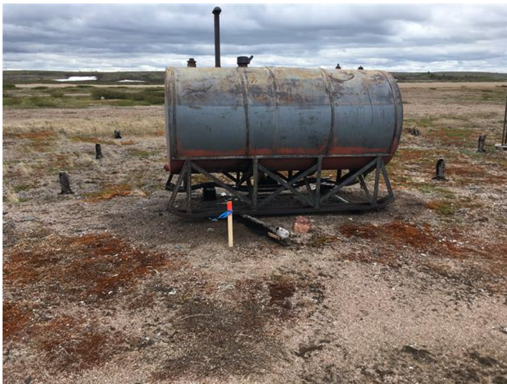
Photo 6 – Camp / Antenna Areas and AES Compound: empty 4,546 L AST on east end of area. Looking south.
