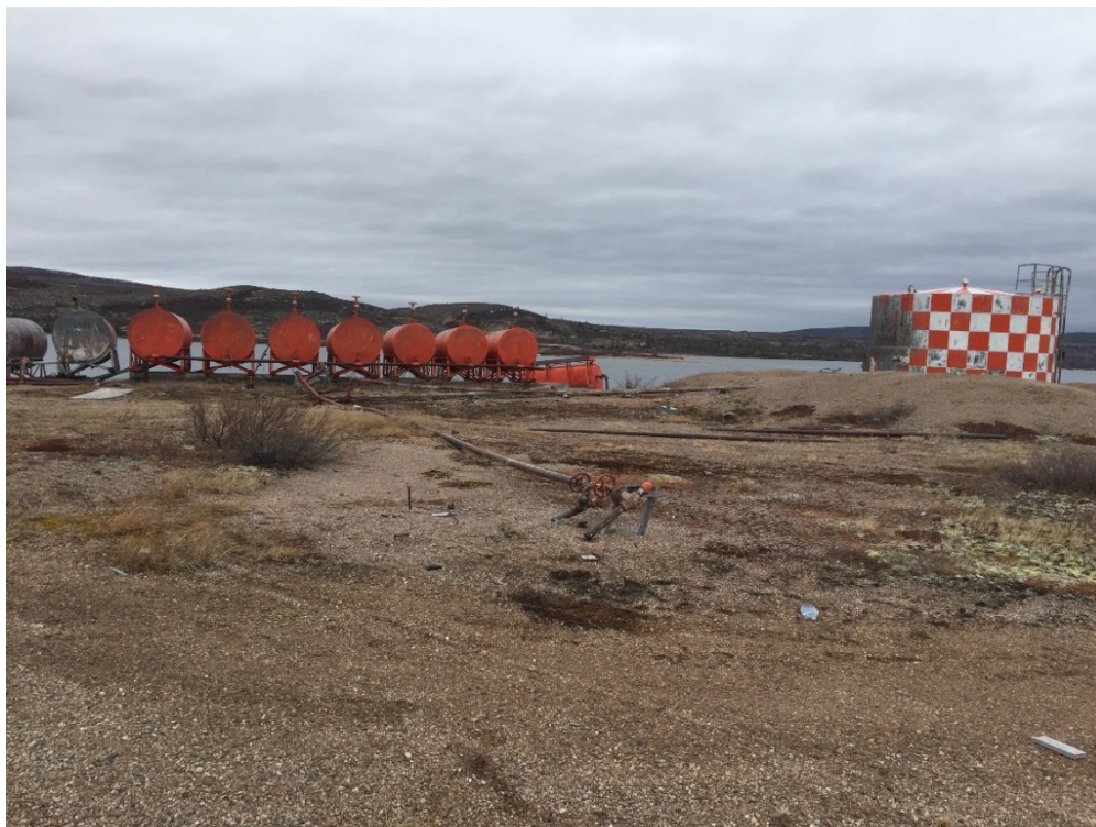
Photo 10 – Camp / Antenna Areas and AES Compound: ten 4,500 L ASTs and Dyked 113,516 L Tank in background, re-fueling Area in foreground. Looking north.
