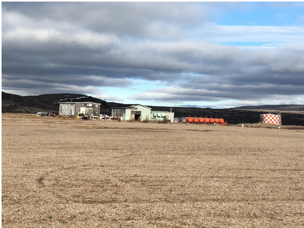
Photo 4 – Camp / Antenna Areas and AES Compound: from left to right, Camp Fuel Shed, Camp Garage Building, Ten 4,500 L ASTs, and Dyked 113,516 L Tank. Looking north.
