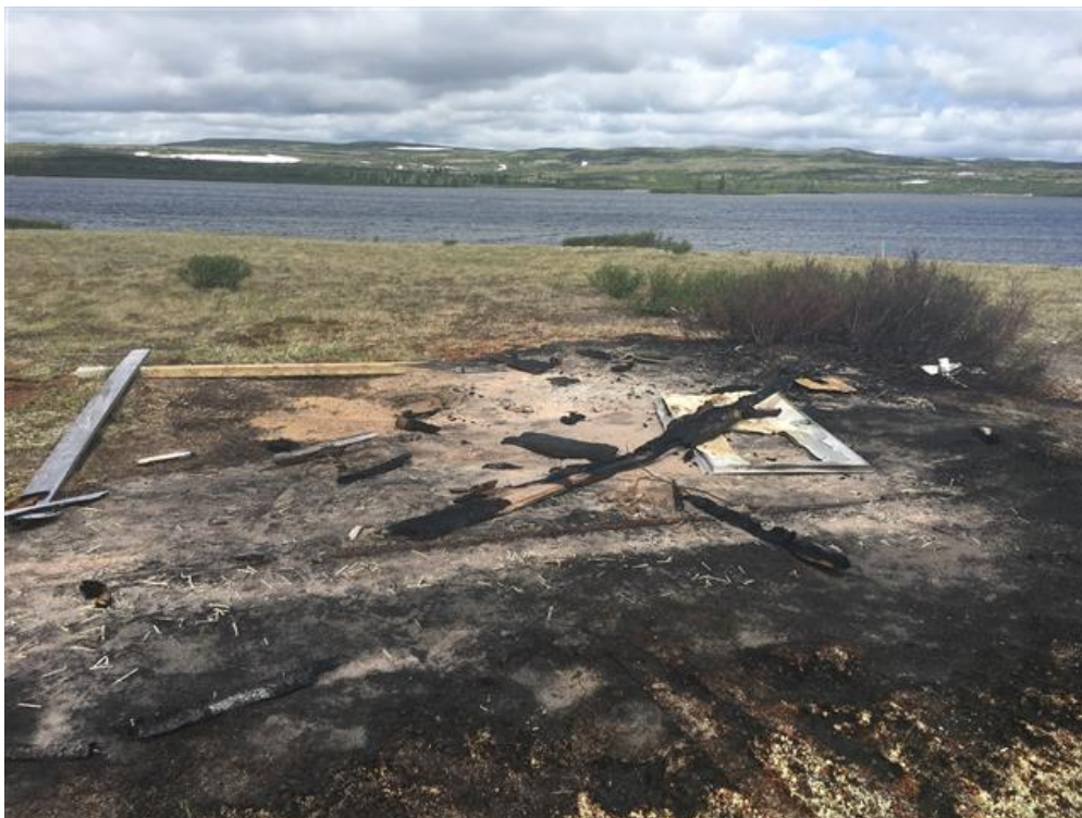
Photo 12 – Unknown Foundation / Building: Burned remains of former building. Looking east.
