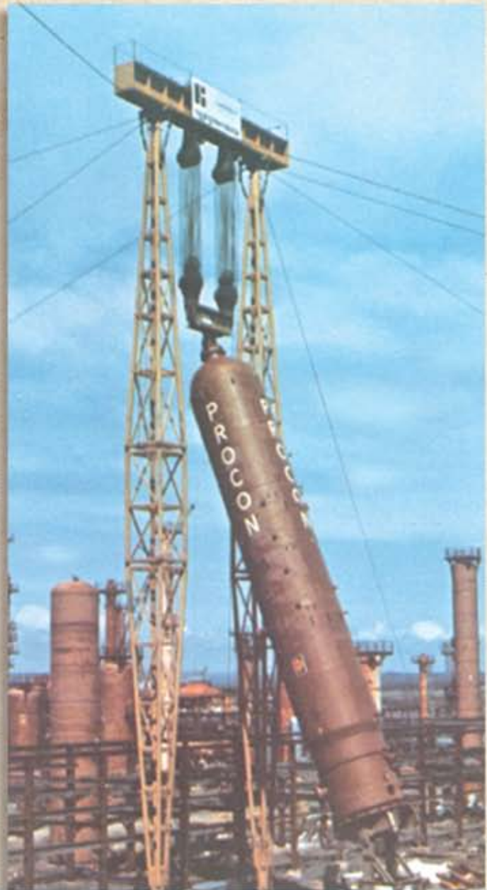
6.41 In 1972, the Isomax reactor lift, part of the Come By Chance refinery's gasoline-producing unit, was the heaviest single lift in North America at 644 metric tonnes (710 tons).
