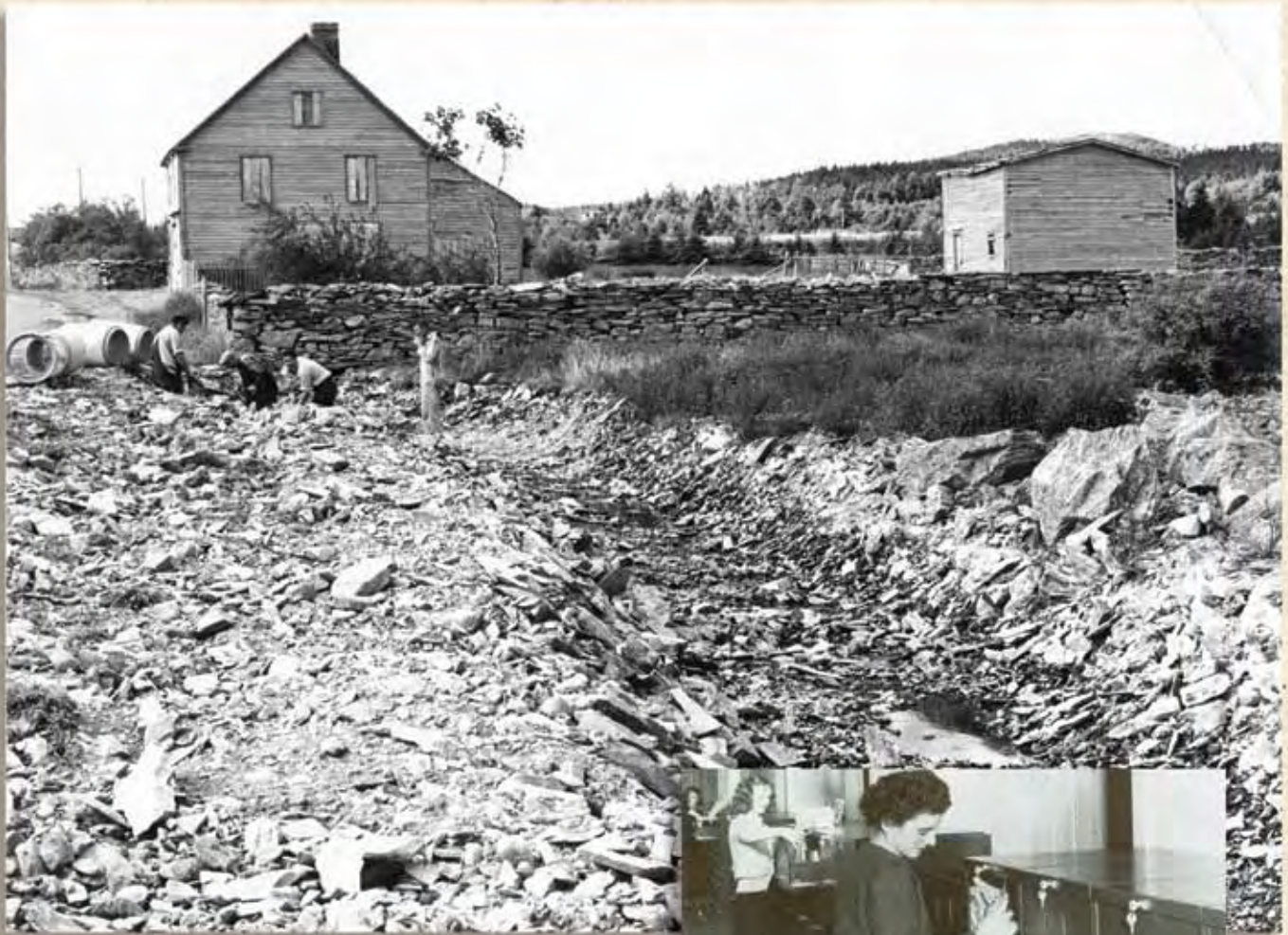
6.50 Constructing a sewer pipe
