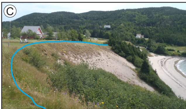
Plate 10. Surveys can be conducted on shore-normal transects, cliff tops or breaks in slope, indicated in blue. A) Shore-normal transect at Port au Port; B) Well-defined cliff top at Parsons Pond; C) Break in a vegetated slope at Sandy Cove.
