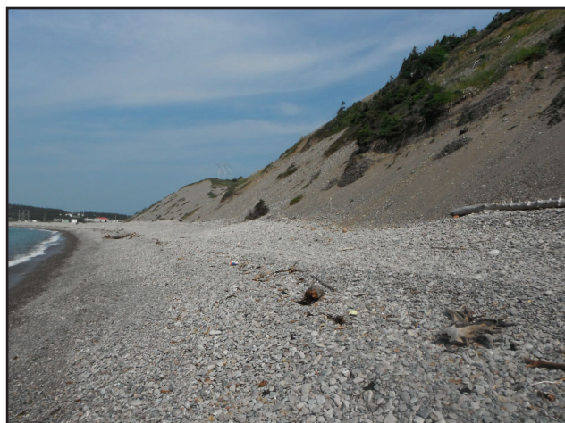
Plate 12. Partly vegetated gravel and sand cliff at Port au Port fronted by a gravel beach, July 2011. Erosion has been minimal along this coastline. Typically, waves do not reach the base of the cliff and groundwater is not present.
