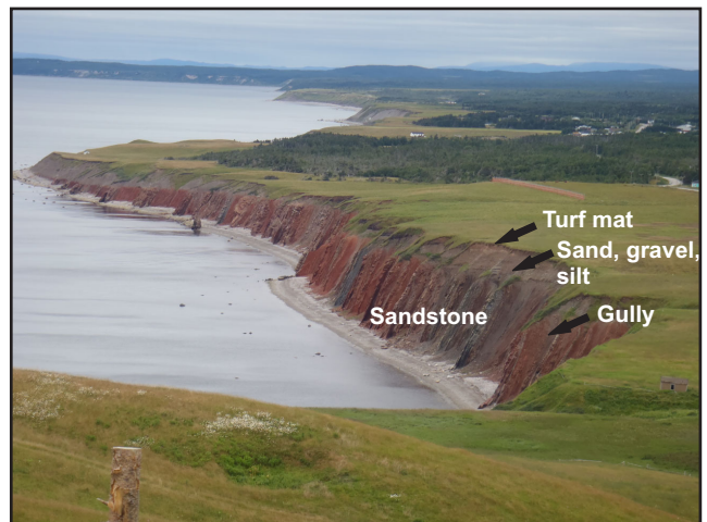
Plate 21. Coastal cliff at Robinsons, June 2013. In contrast to the other monitored sites, the cliff is composed of sedimentary rocks overlain by sand and gravel. Although the sedimentary rocks are soft compared to many other types of bedrock, they are harder and more resistant to erosion than unconsolidated sediment. Wind and water can loosen and move rock fragments from the cliff face.
