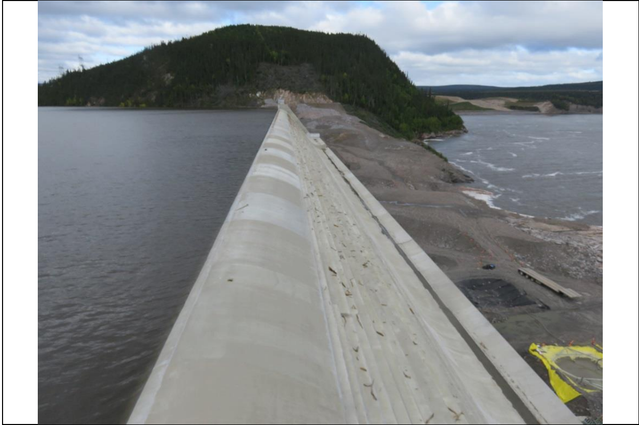
Photo A.3: Northerly view along north RCC dam.
