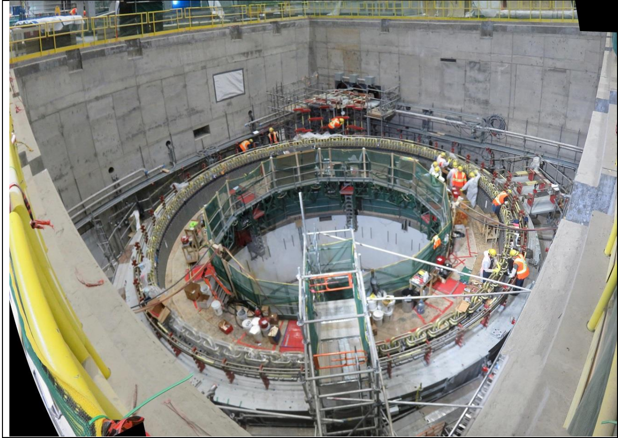
Photo B.3: Unit 2 with stator winding installation in progress.
