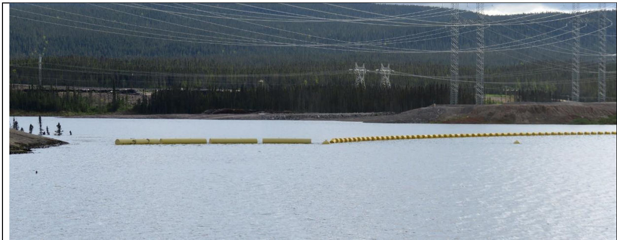
Photo A.5: Downstream view of temporary boom, with no accumulated debris.
