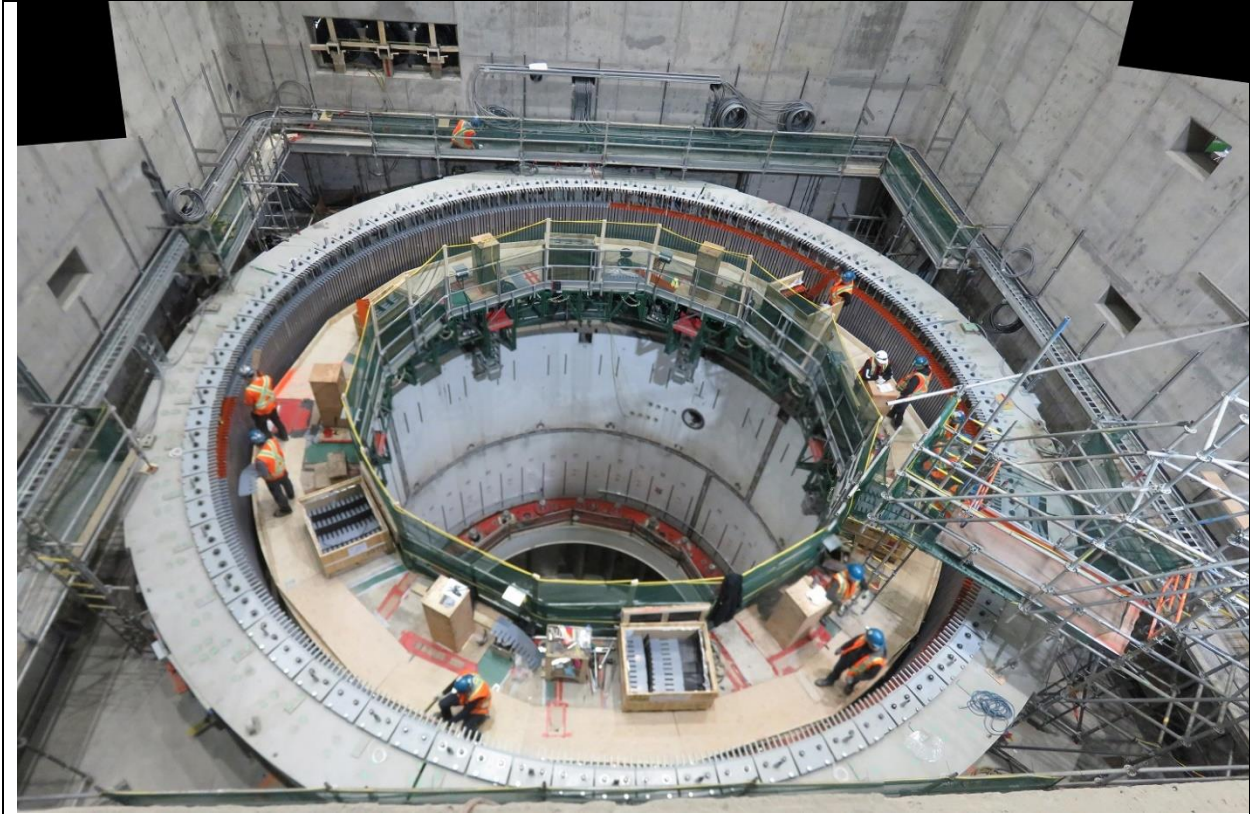
Photo B.4: Unit 3, with stator core stacking in progress.
