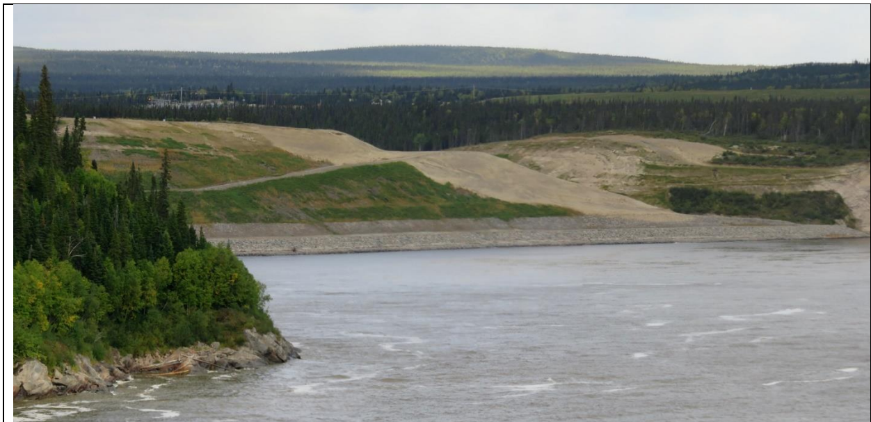
Photo D.2: Downstream side of North Spur.
