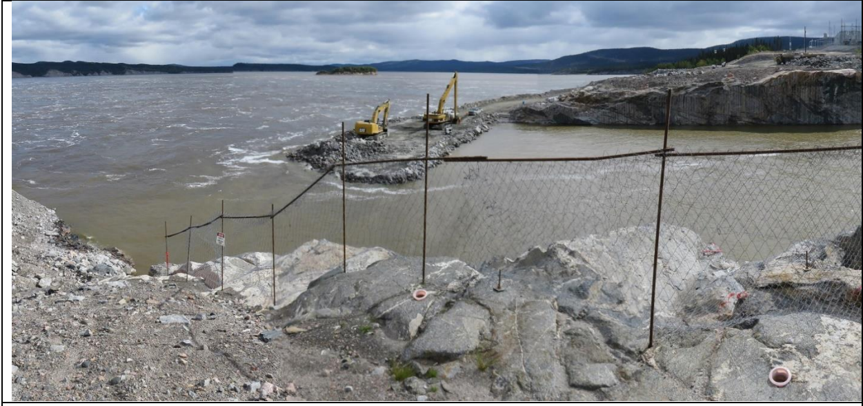
Photo C.3: Removal of tailrace rock plug in progress.
