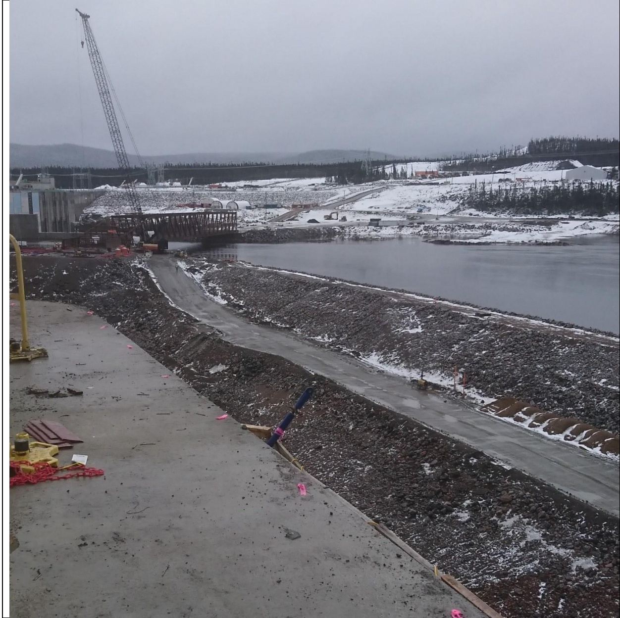
Photo D.5: Upstream cofferdam.
