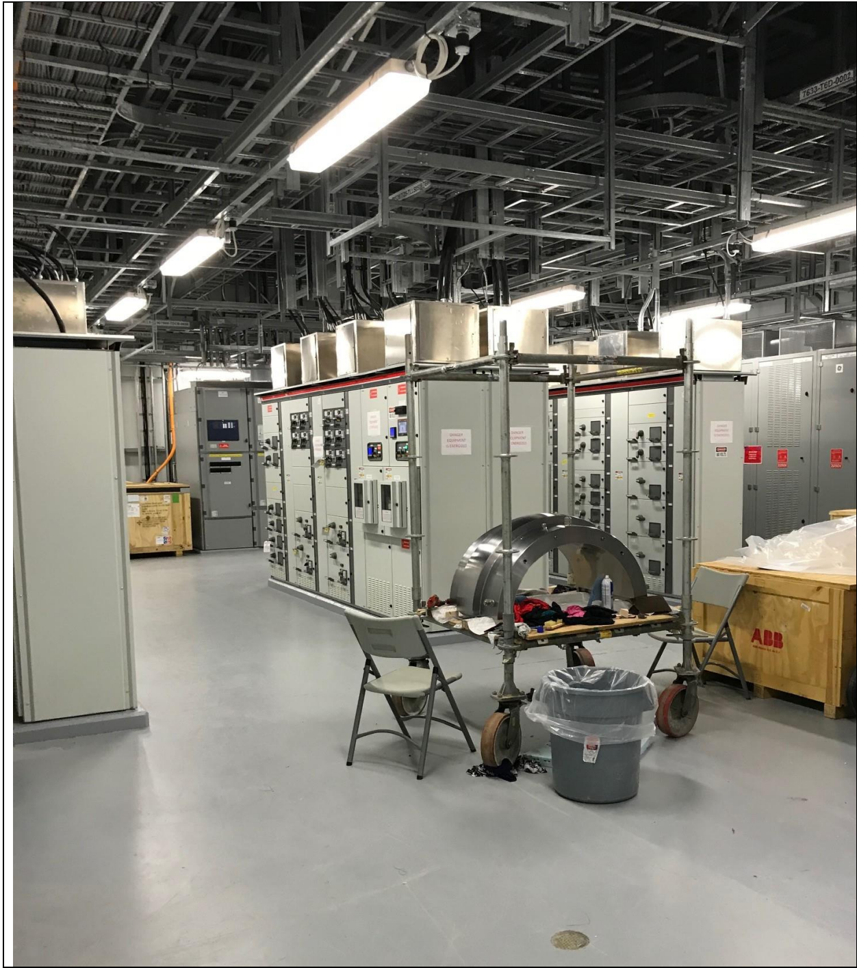
Photo F.2: . SOP Unit 1 bearing shell.
