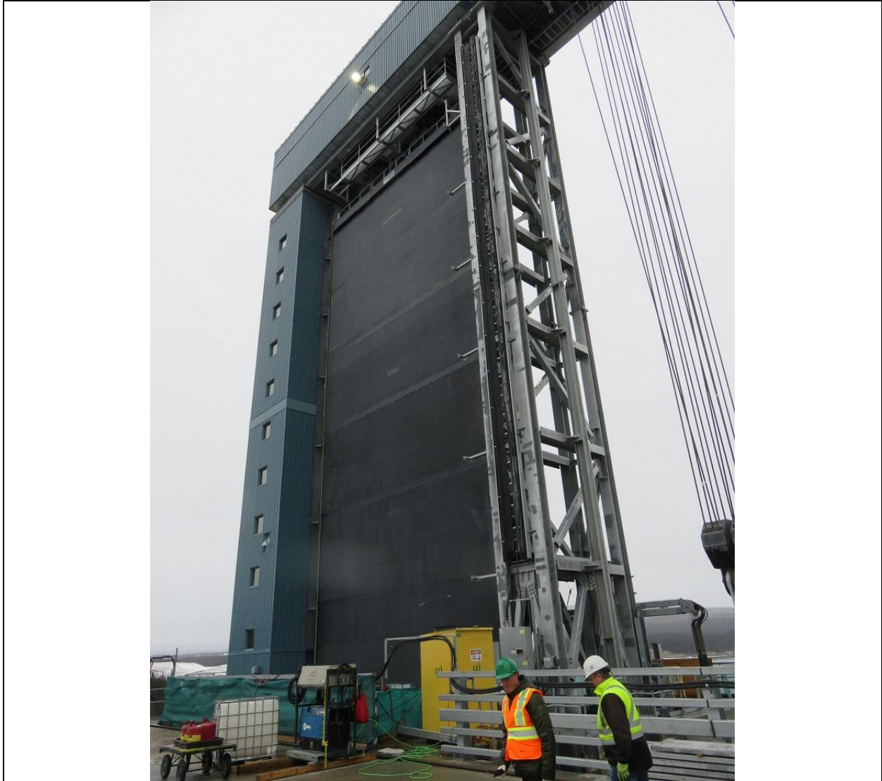
Photo C.2: Spillway gate in raised position in Bay 5.
