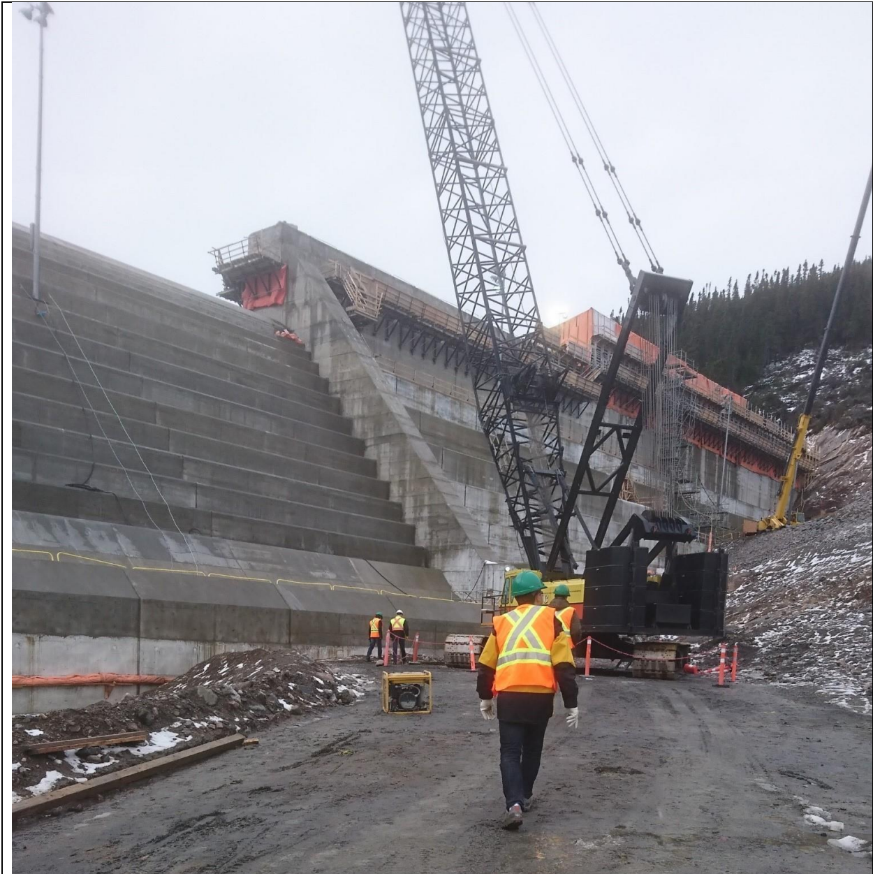
Photo D.2: Non-overflow section of north RCC dam.
