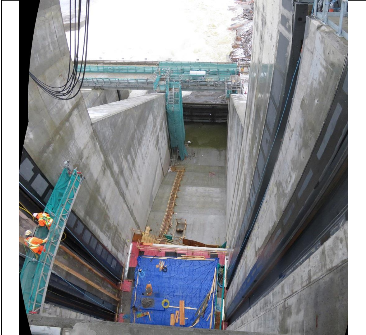
Photo C.1: Local concrete repair between gate guides in spillway bay 1.
