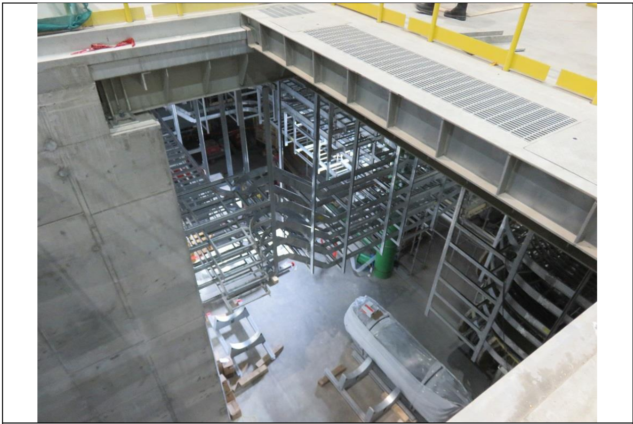
Photo B.7: Cable trays installed below generator floor.
