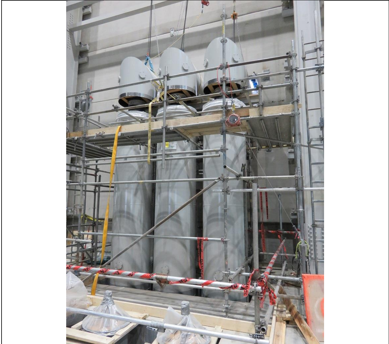
Photo B.8: Installation of isolated phase bus in progress.
