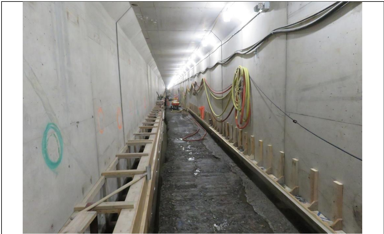
Photo D.4: Drainage gallery inside north RCC dam.
