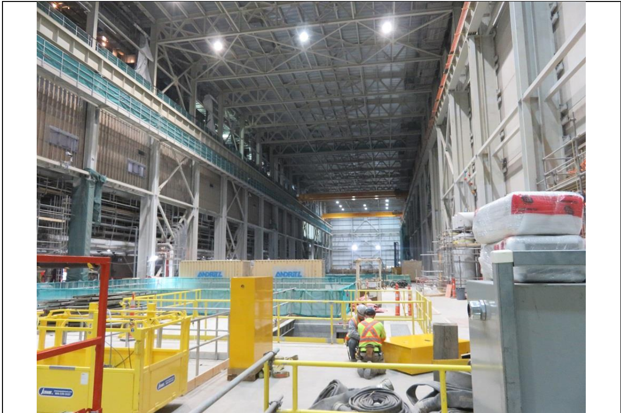
Photo B.3: Interior view of powerhouse from main service bay.
