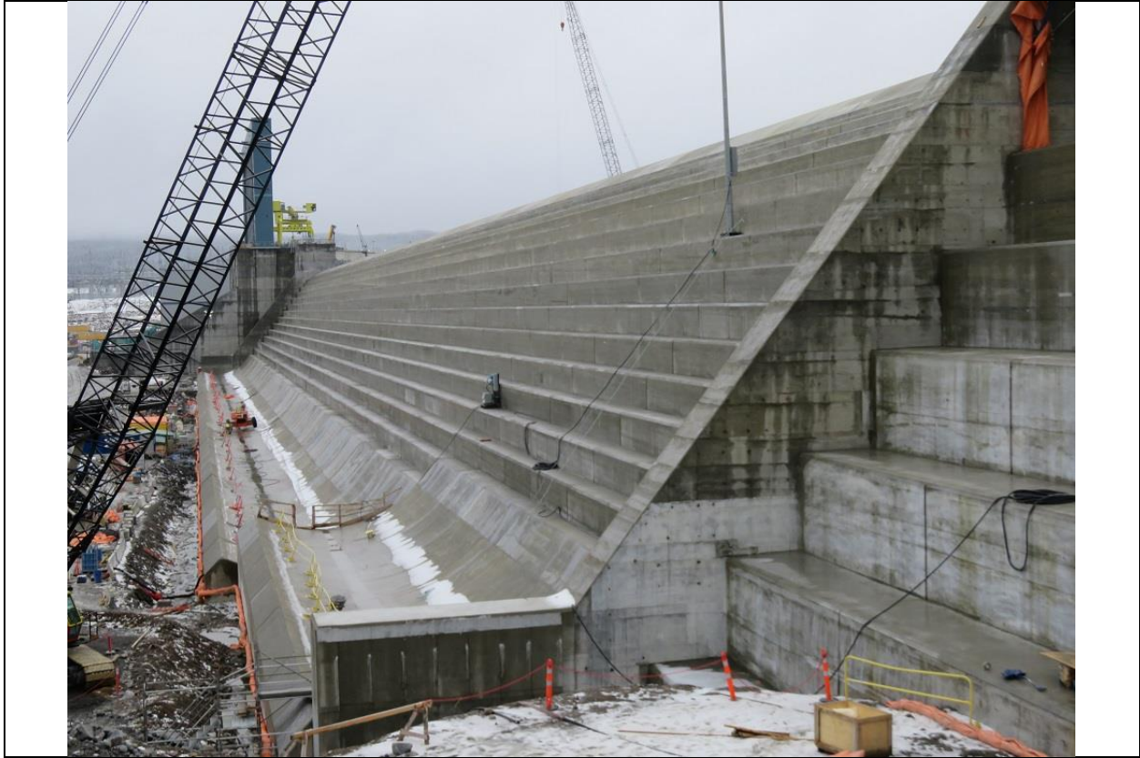
Photo D.3: Downstream side of north RCC dam.
