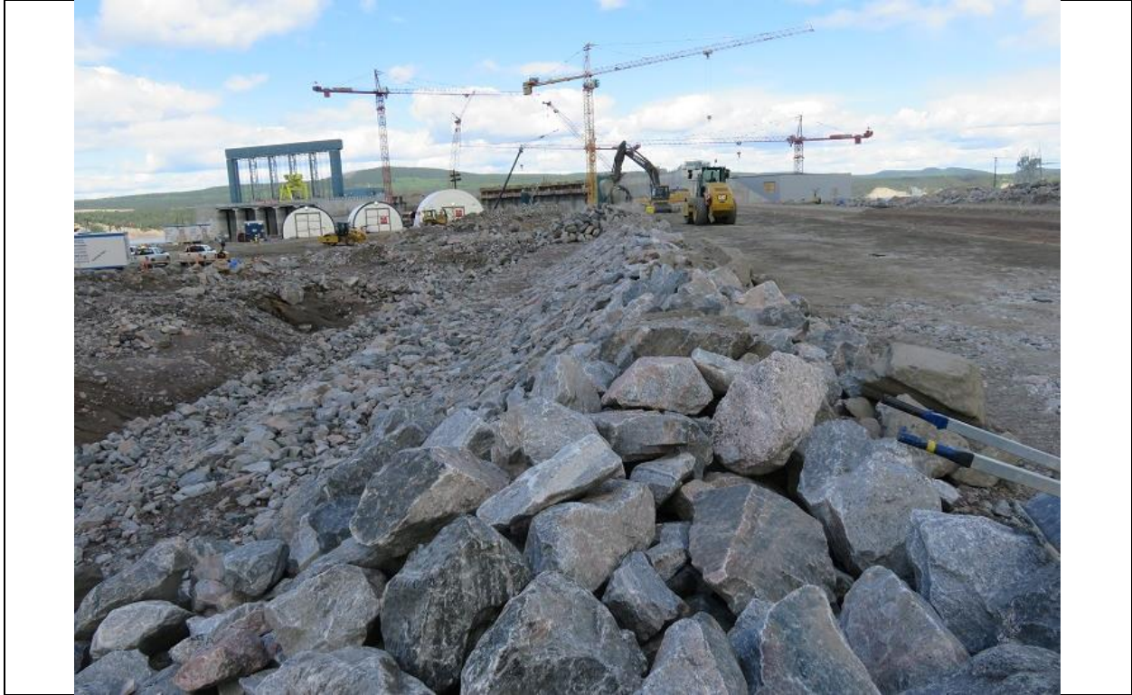
Photo D.5: Neatly-placed riprap along upstream side of south embankment dam.
