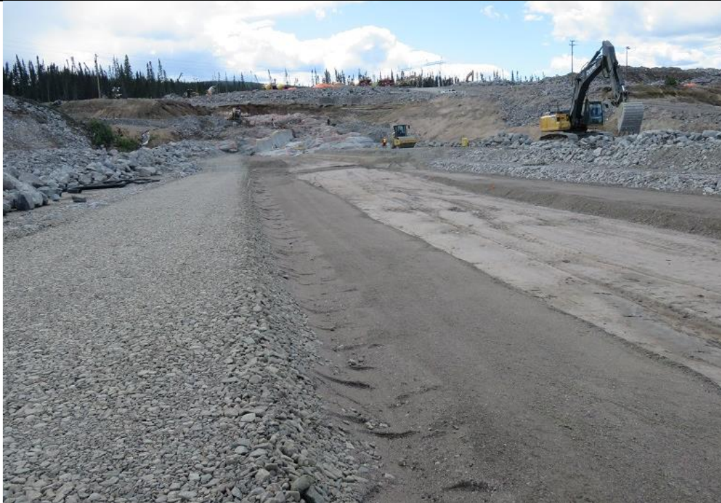
Photo D.1: Southerly view along south embankment dam towards right abutment.
