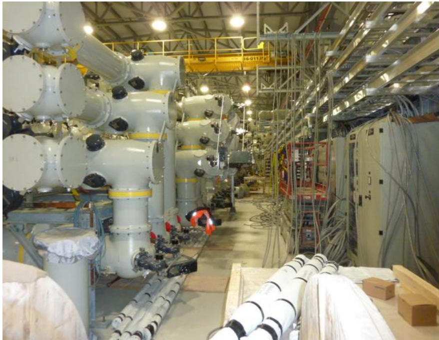
Photo F.8: GIS Equipment and control cabinets installation
