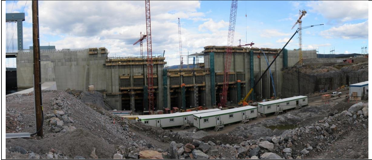
Photo A.1: Panoramic view of upstream side of power intake structure.
