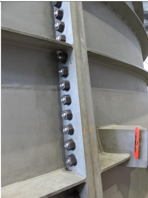
Photo A.12: Bolting details for draft tube liner segments.
