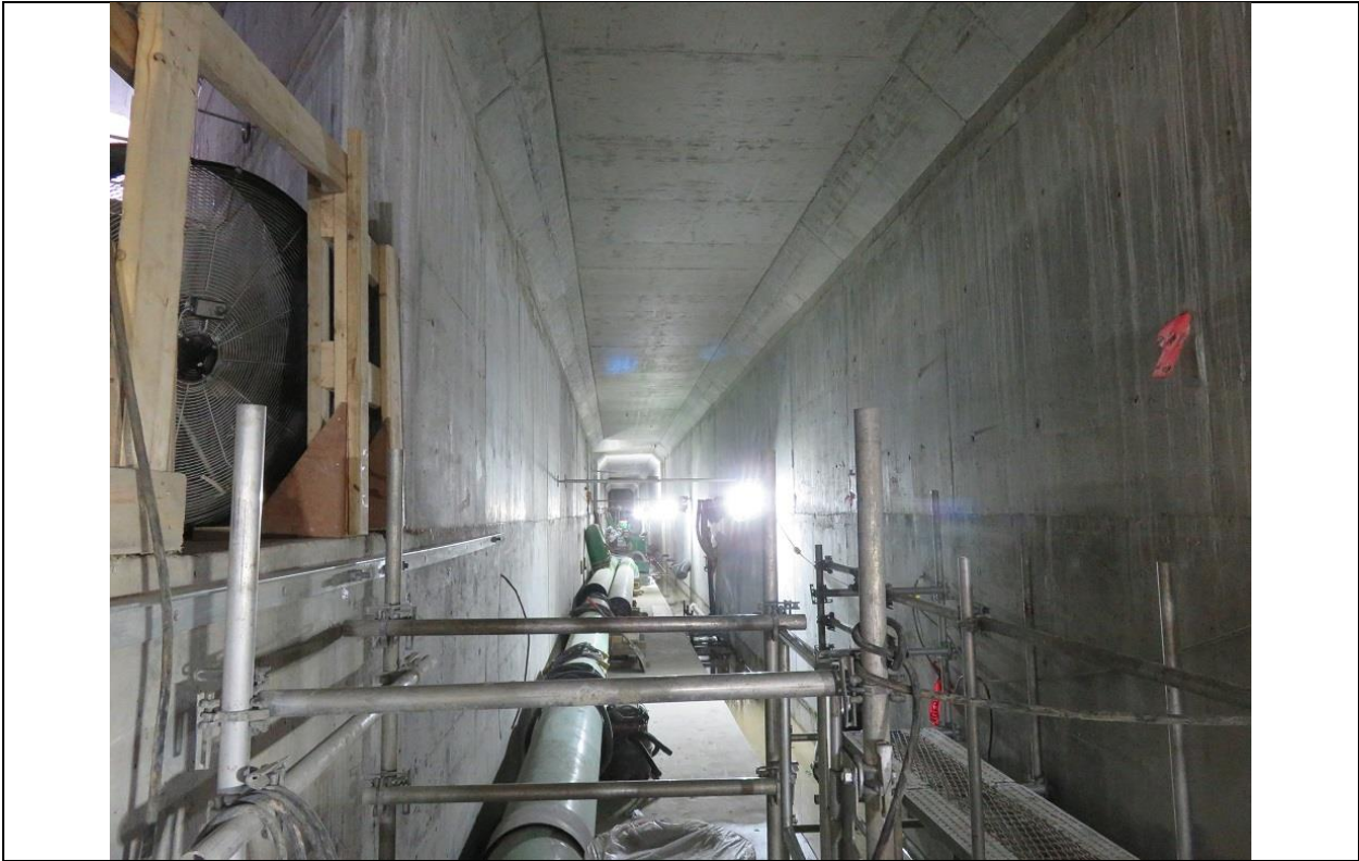
Photo A.10: Powerhouse drainage gallery.
