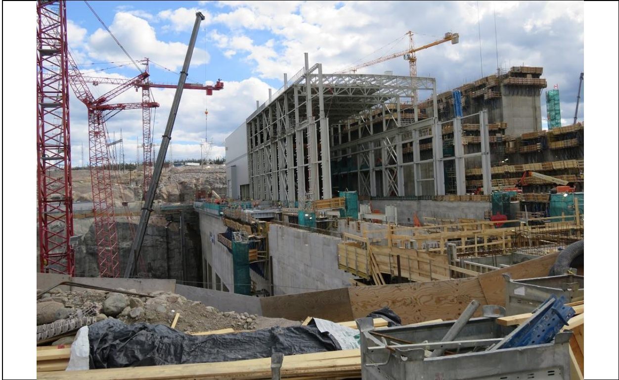
Photo A.3: Southerly view of powerhouse steel superstructure from downstream side.
