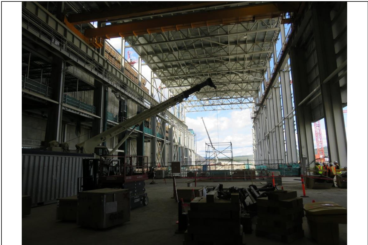
Photo A.4: Inside of powerhouse superstructure, viewed from south service bay.
