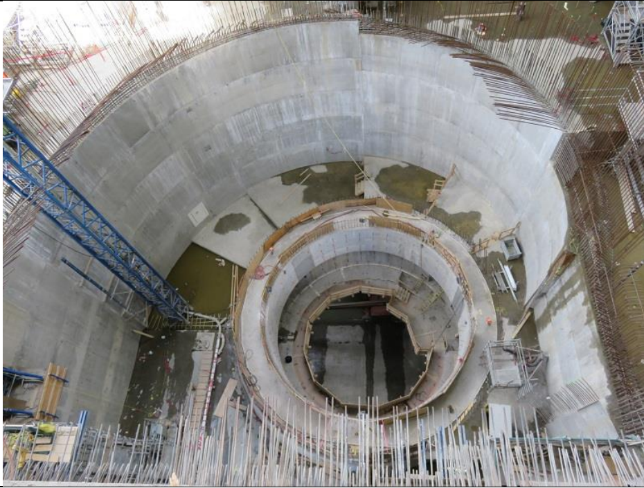
Photo A.7: Completed first stage concrete in Unit 1.
