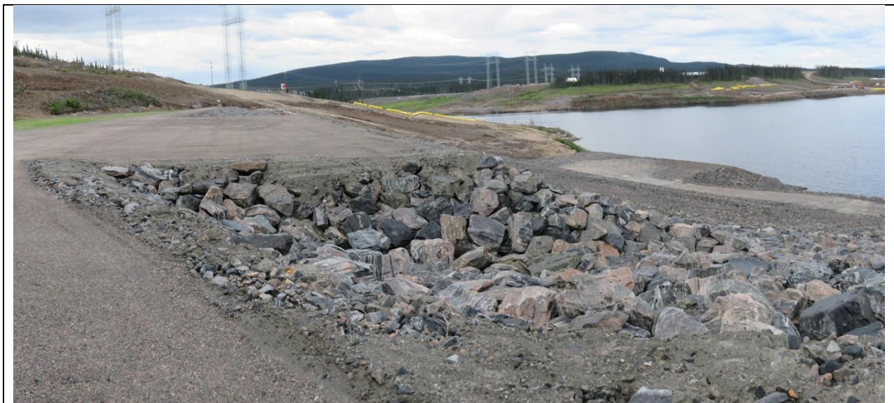
Photo E.4: Southerly view showing log boom platforms at El. 43 m and E. 27 m. Reservoir level is El. 20.33 m. Yellow log boom sections are visible on shore in upper centre and upper right of photo.
