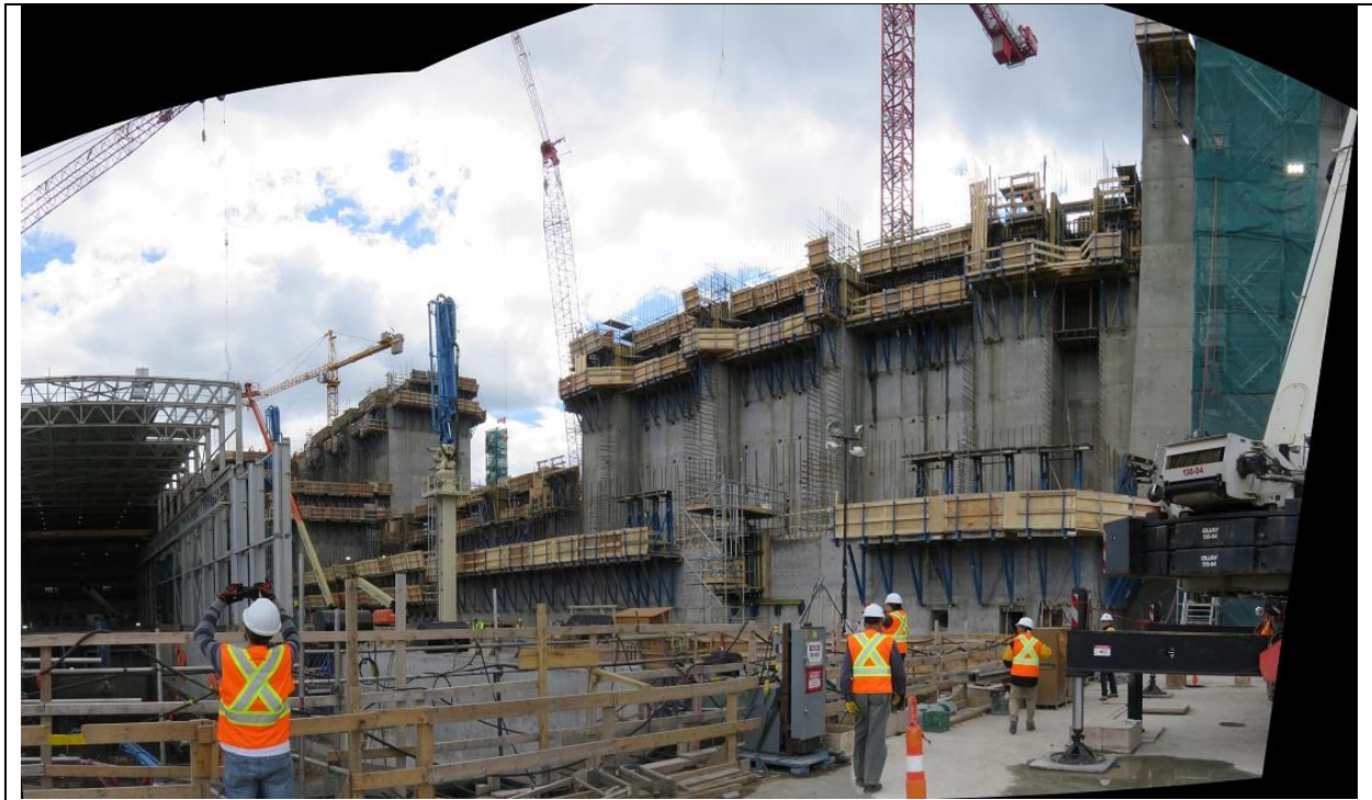
Photo A.2: Panoramic view of downstream side of power intake structure.
