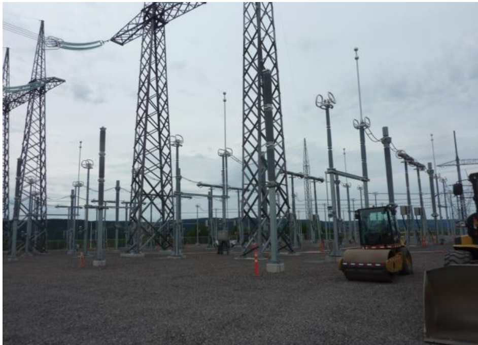
Photo G.2: CF Switchyard - grade completion
