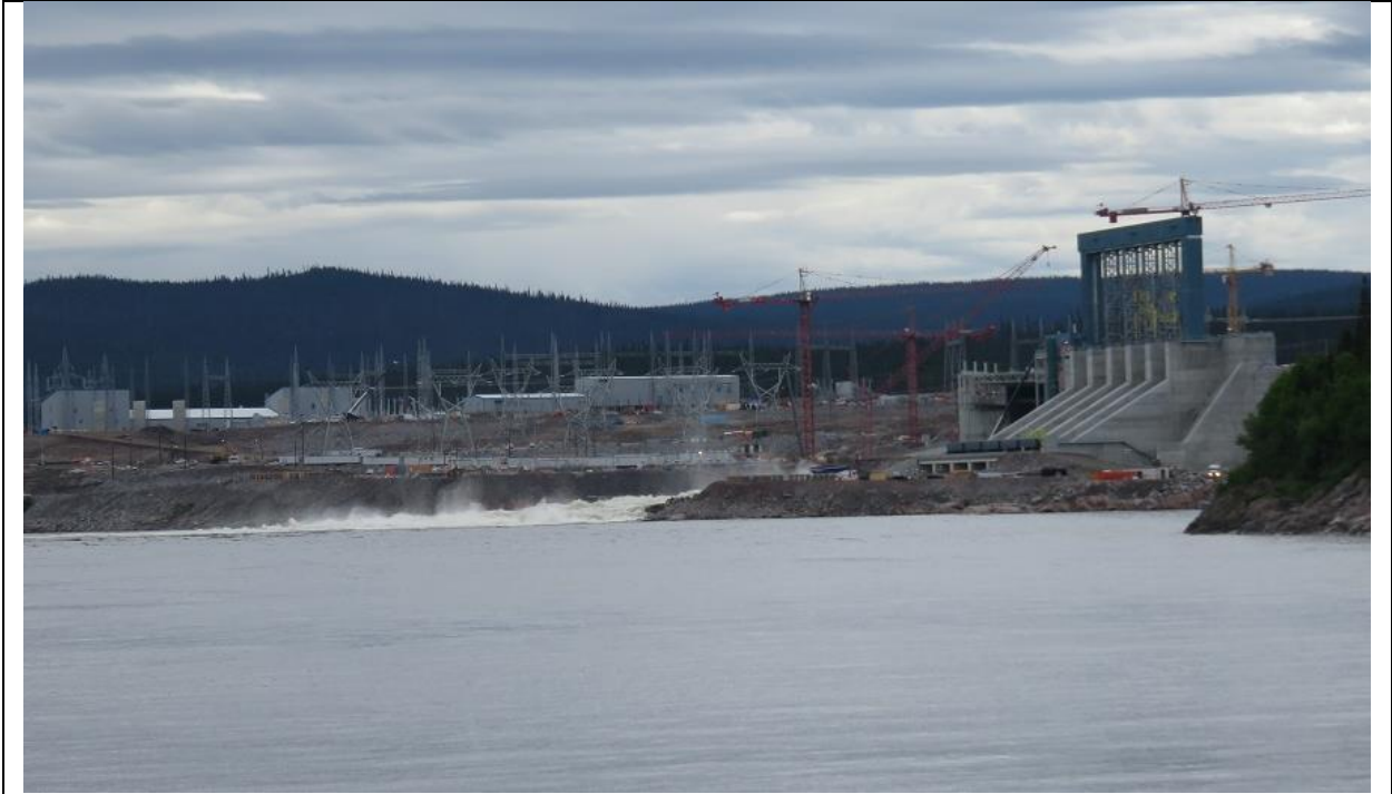
Photo B.3: Spillway release viewed from North Spur.
