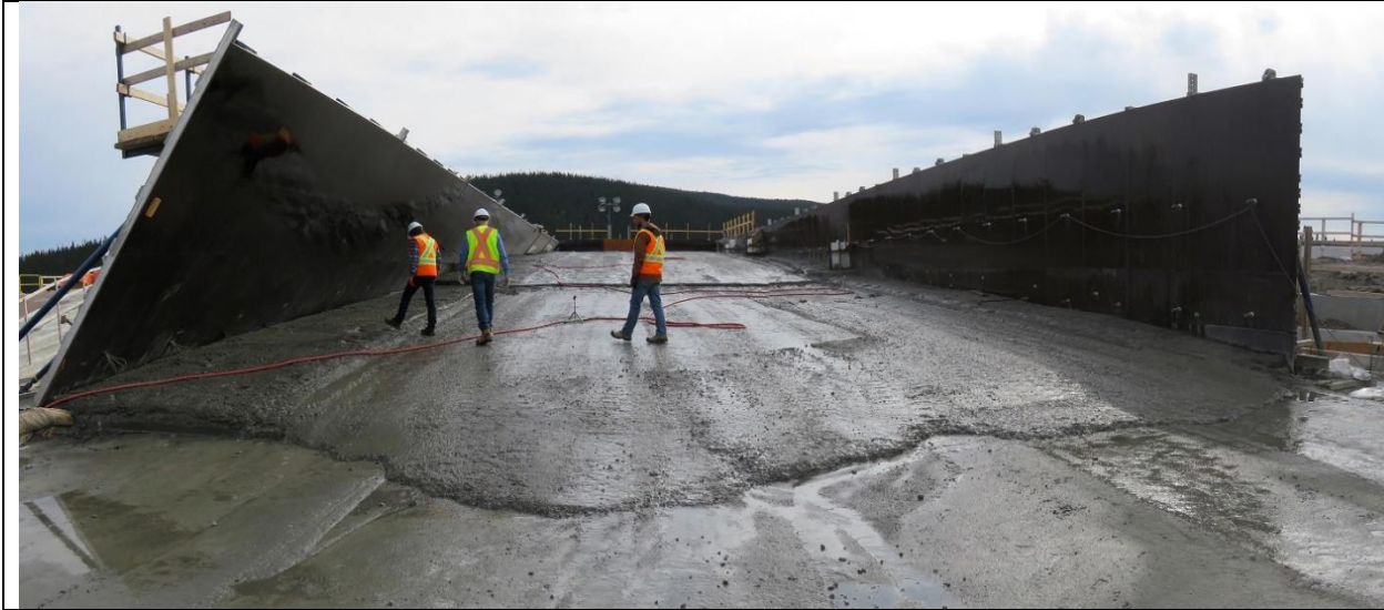
Photo C.11: Recently-placed 2017 RCC trial.
