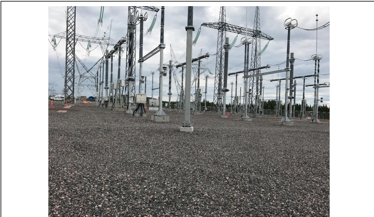
Photo G.4: CF Switchyard Extension essentially completed.
