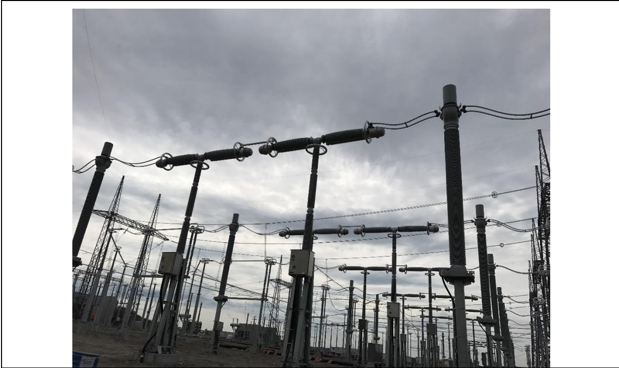
Photo G.3: CF Switchyard equipment installation completed.
