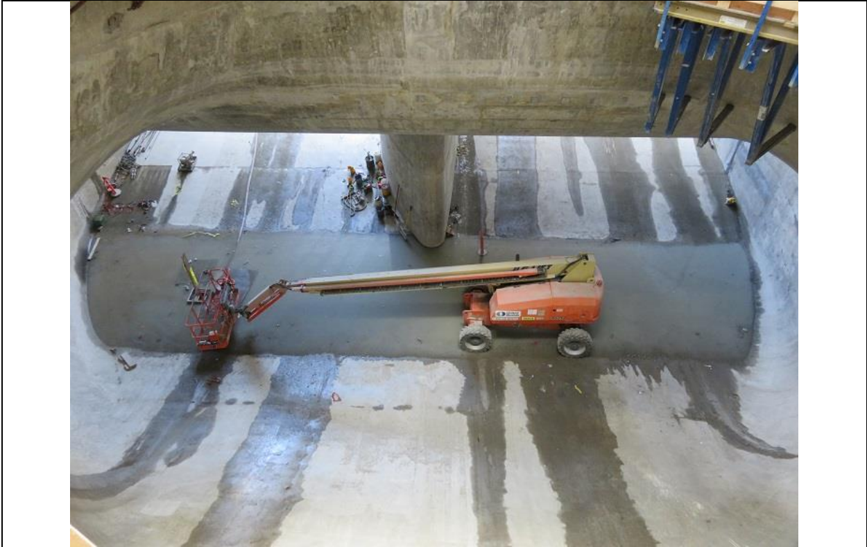
Photo A.9: Looking down into Unit 1 draft tube outlets.
