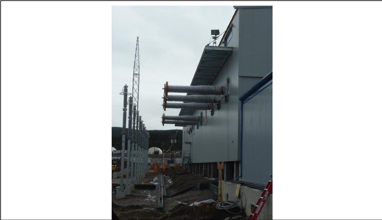
Photo F.6: GIS Building - Wall bushings
