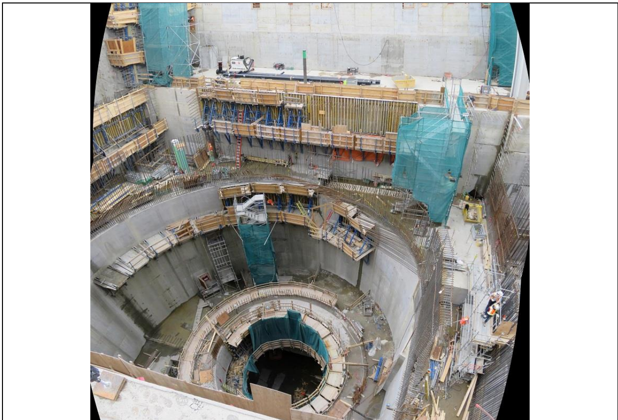
Photo A.6: First stage concrete works nearing completion in Unit 4.
