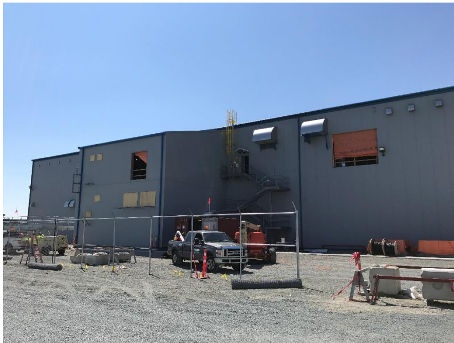
Photo H.14: Synchronous Condensers Power and Exciter Transformers.
