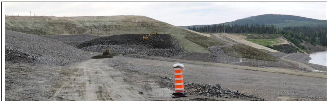
Photo E.6: Northerly panorama view along downstream side of North Spur slope stabilization works. Kettle Lakes discharge channel is at far right. Note local surface erosion (rolling) of upper slope.
