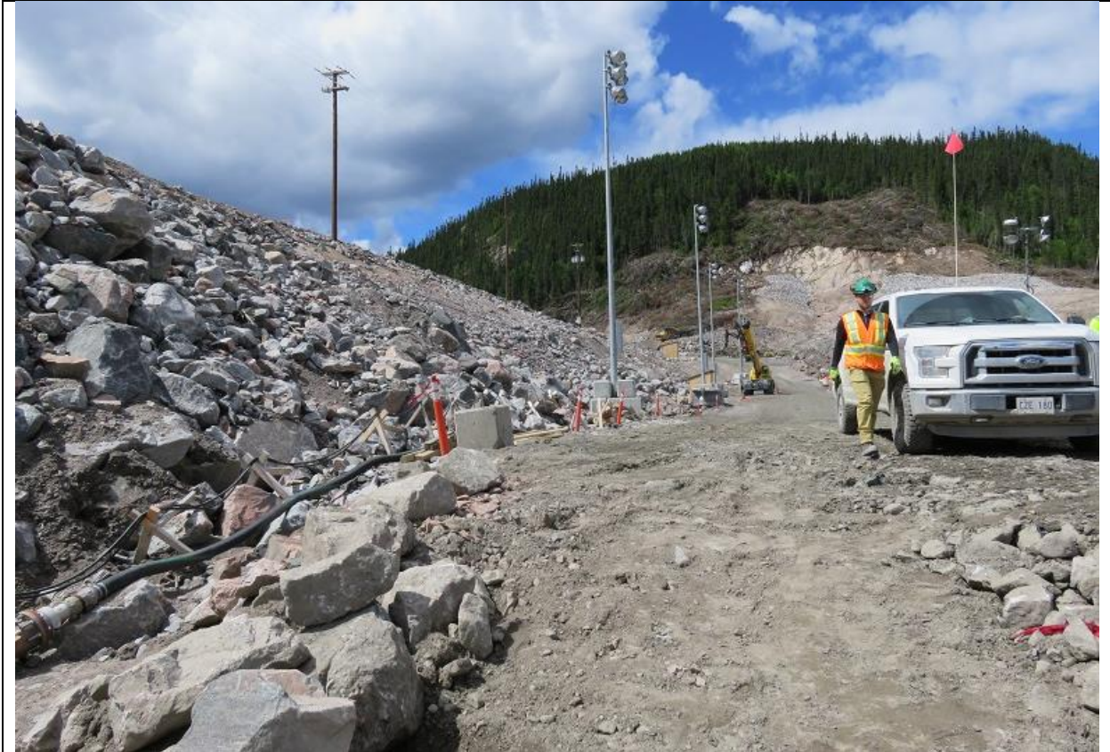
Photo C.1: Northerly view along toe of upstream cofferdam.
