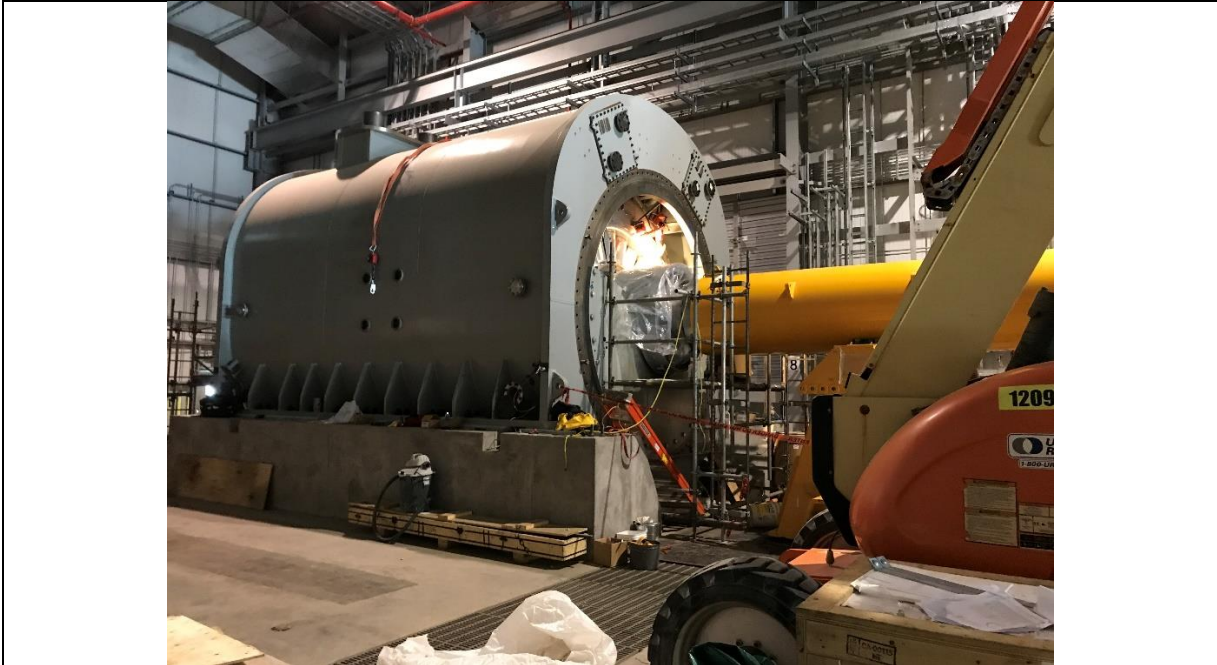
Photo H.15: Synchronous Condenser Unit 1 fully installed on concrete pedestals.
