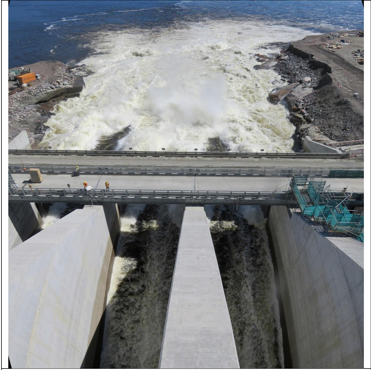
Photo C.3: Spillway outlet channel with central three gates partially open. Bays 1 and 5 are closed for rollway construction.
