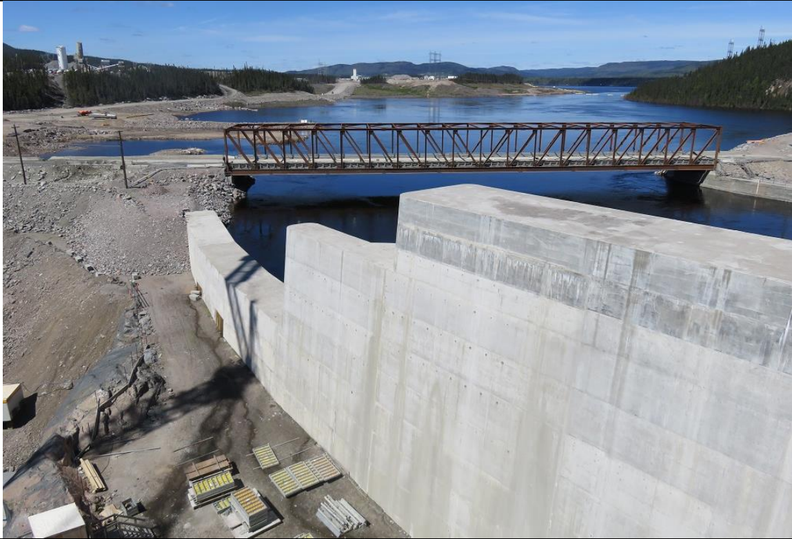
Photo A.1: Upstream view of spillway approach channel and lower reservoir.
