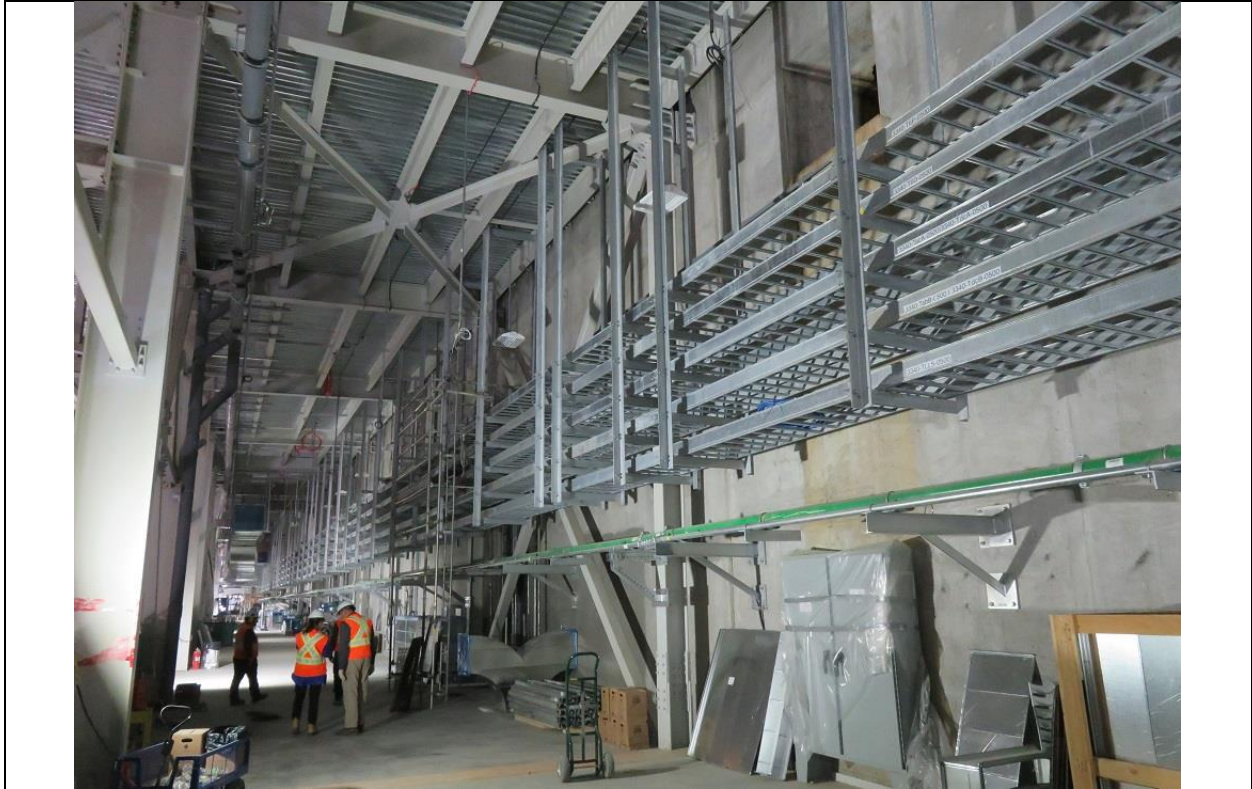
Photo B.6: Mezzanine floor.
