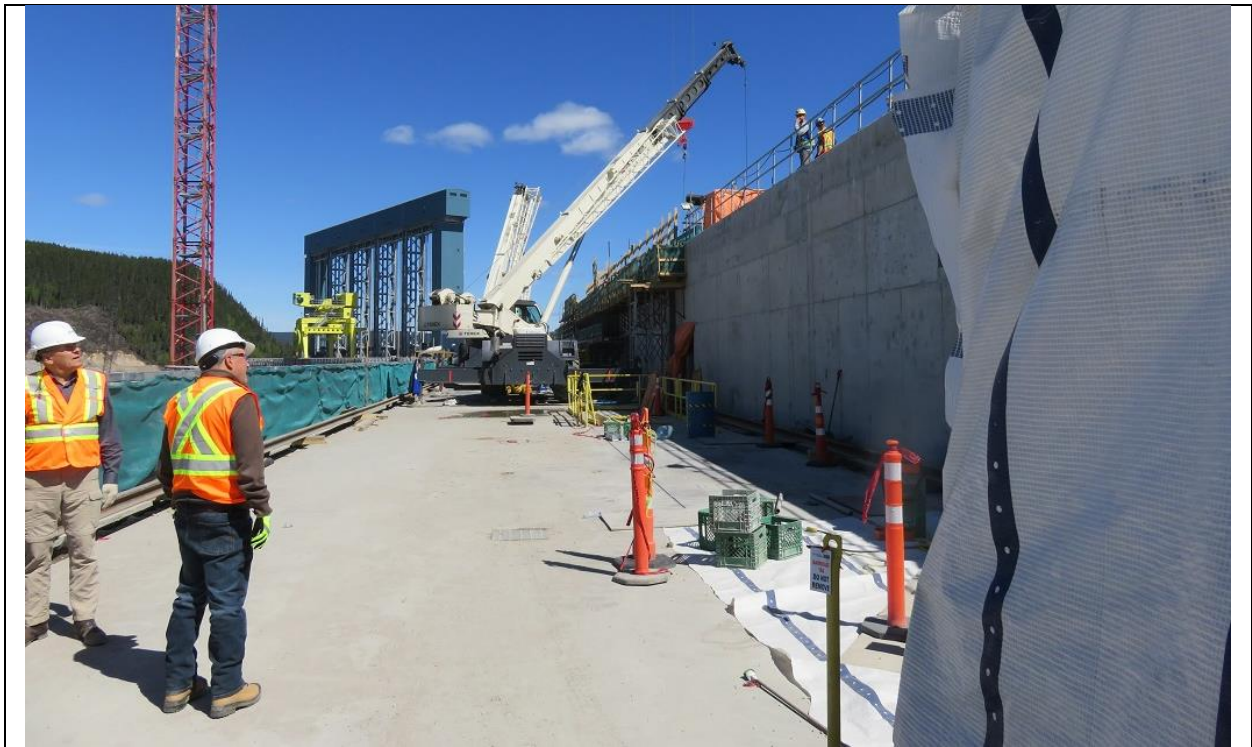
Photo B.2: Power intakes deck.
