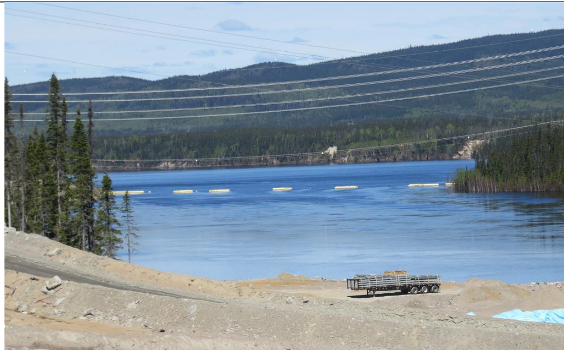
Photo A.2: Upstream view of debris boom, showing irregular spacing of buoys due to slippage of clamps.
