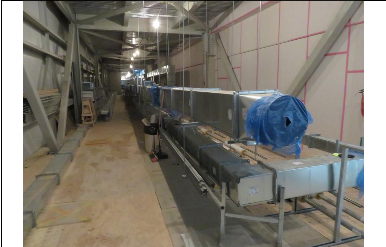
Photo B.7: Powerhouse HVAC works in progress.
