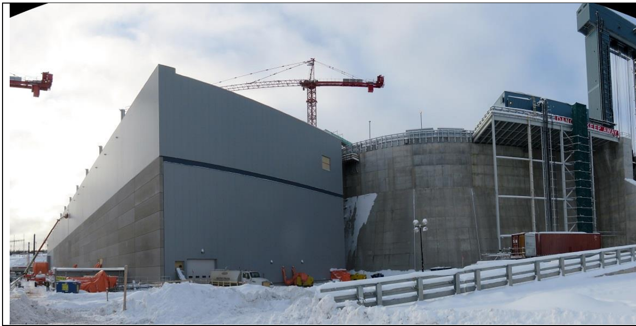
Photo B.2: Panorama view of powerhouse building and centre transition dam.
