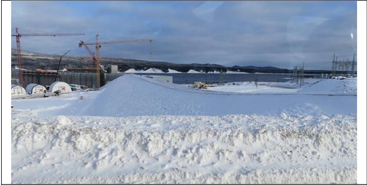
Photo E.1: Upstream side of completed south embankment dam.
