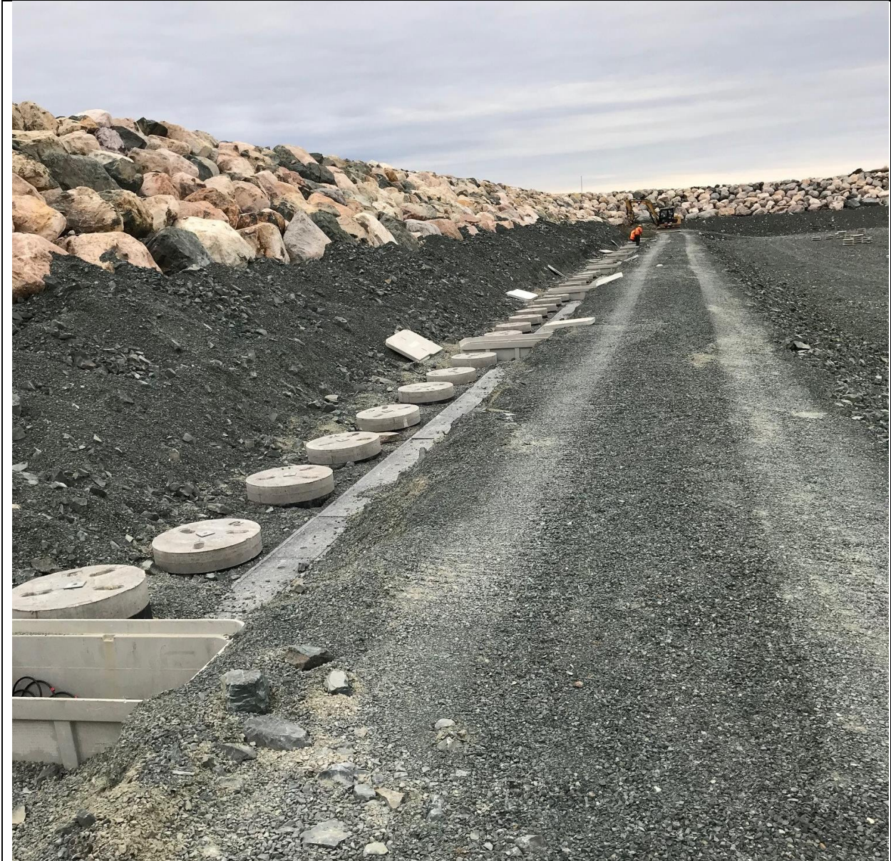
Photo H.3: Dowden's Point electrode wells.
