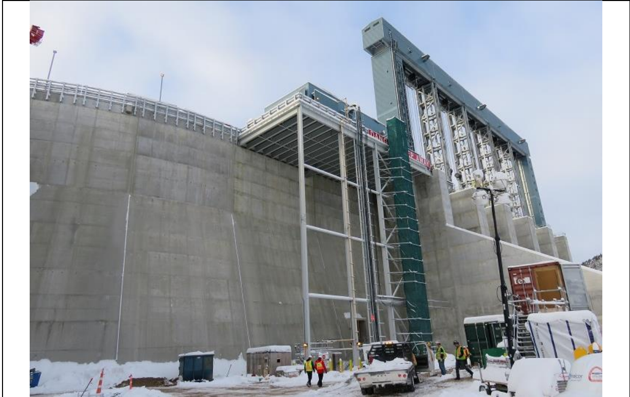
Photo C.1: Centre transition dam and spillway.
