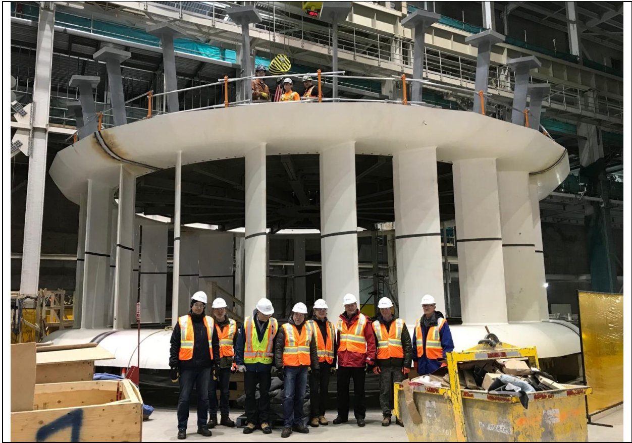
Photo B.5: Unit 1 turbine stay ring.
