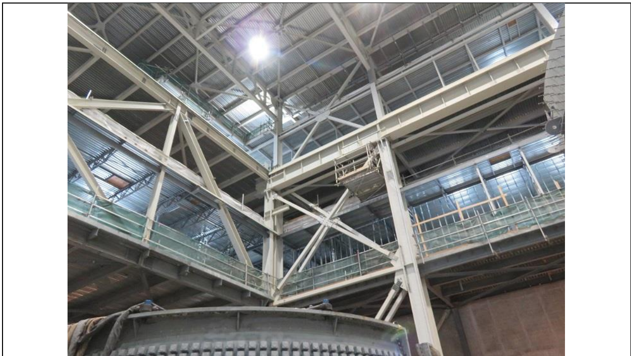
Photo B.4: Mezzanine floors inside powerhouse (above service bay).
