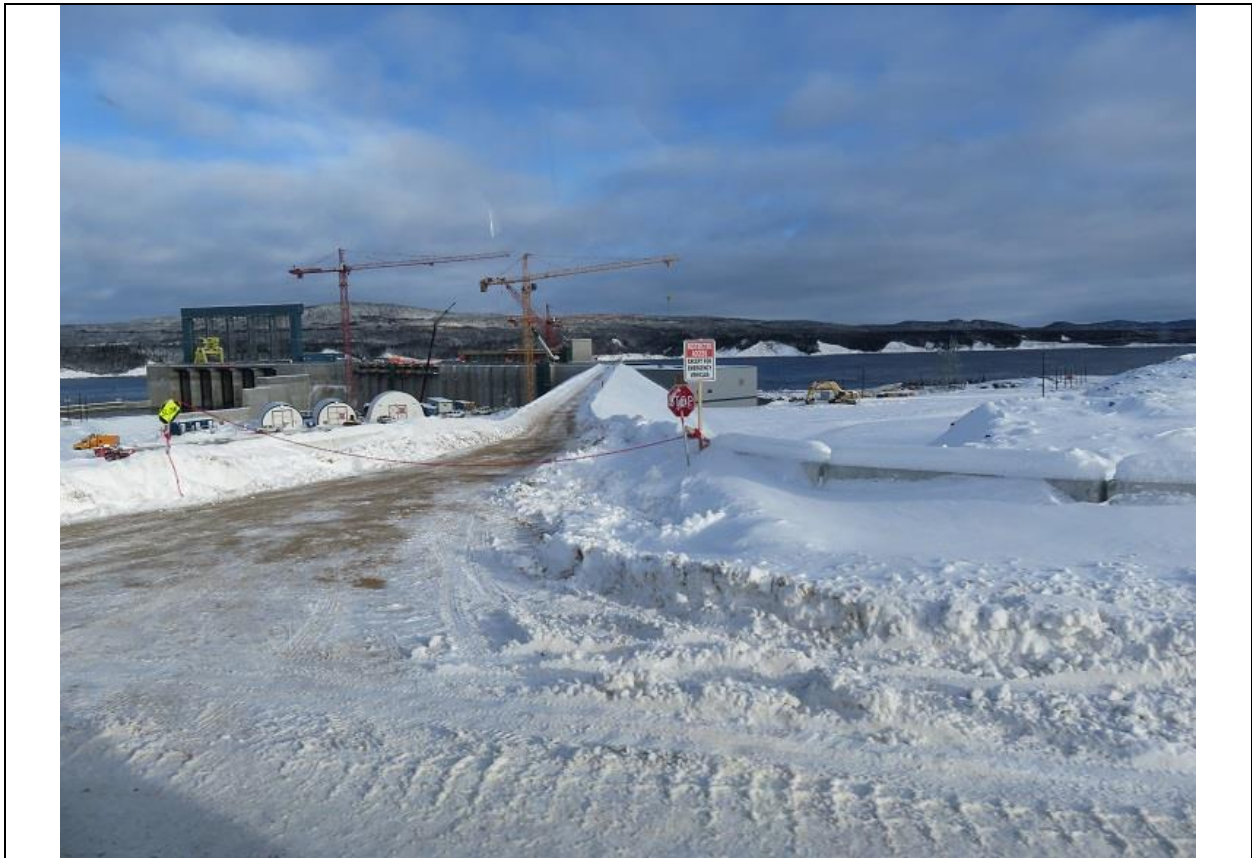
Photo E.2: View along crest of completed south embankment dam.
