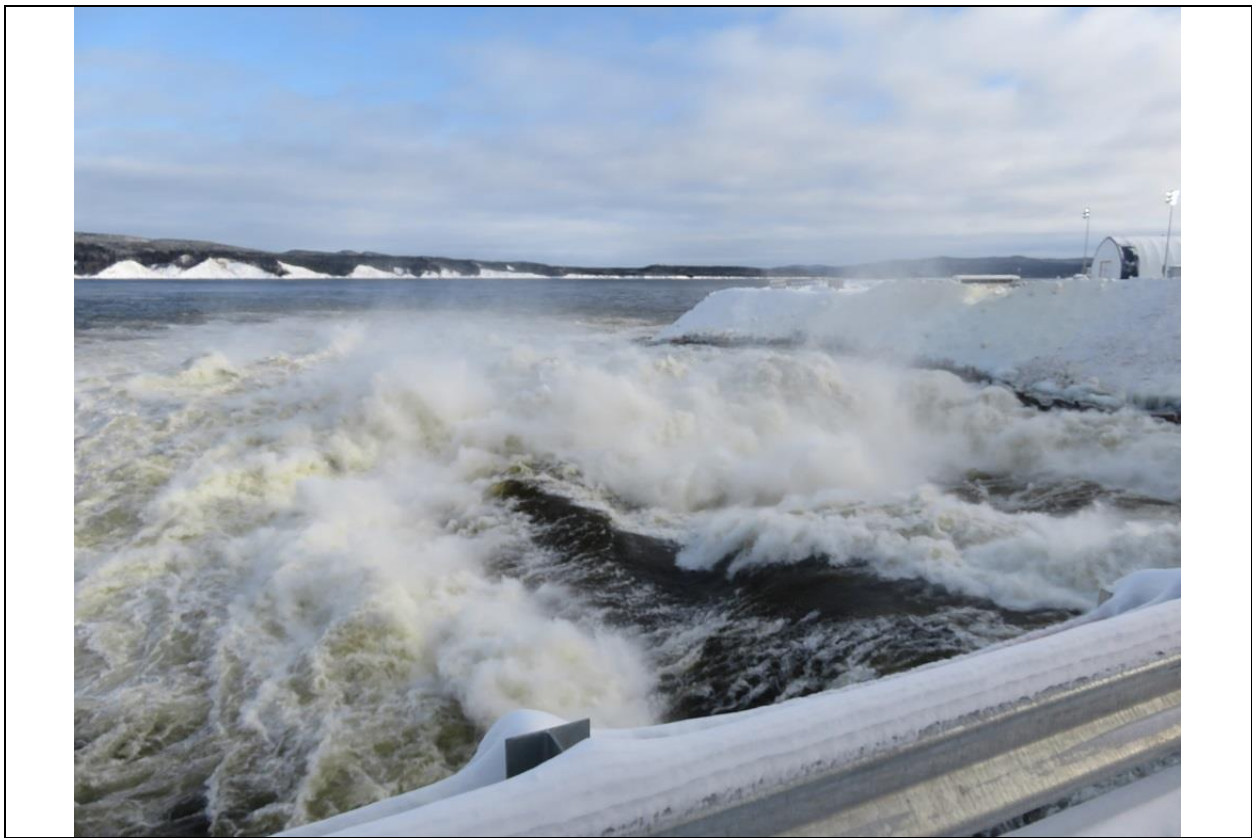
Photo C.4: Spillway discharge entering river.
