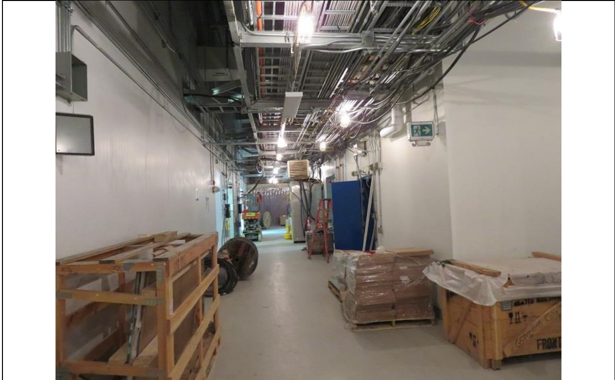
Photo G.1: Soldier's Pond converter building interior works nearing completion.
