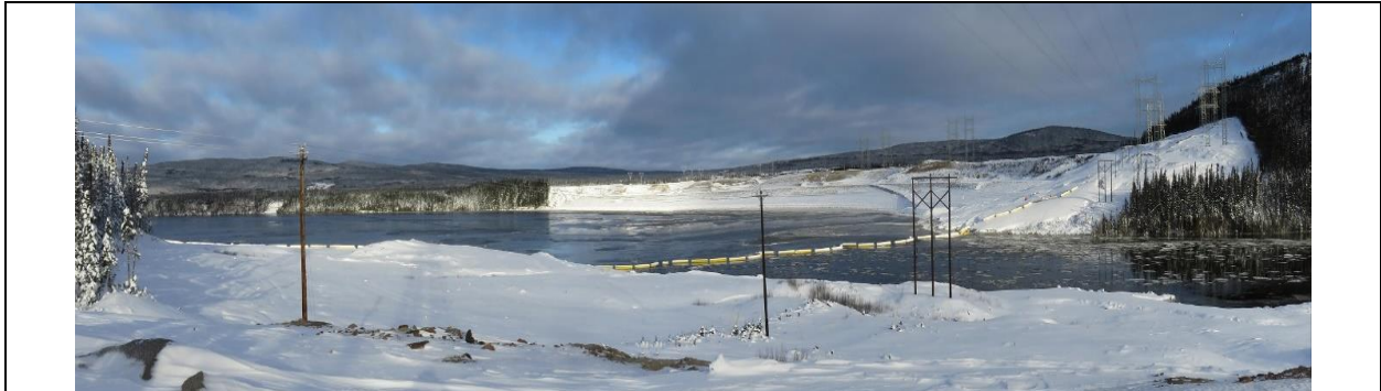
Photo A.1: Upstream view of lower reservoir, with debris/ice/safety boom installed. Reservoir level is about El. 22 m. Snow-covered area in background is upstream side of North Spur.
