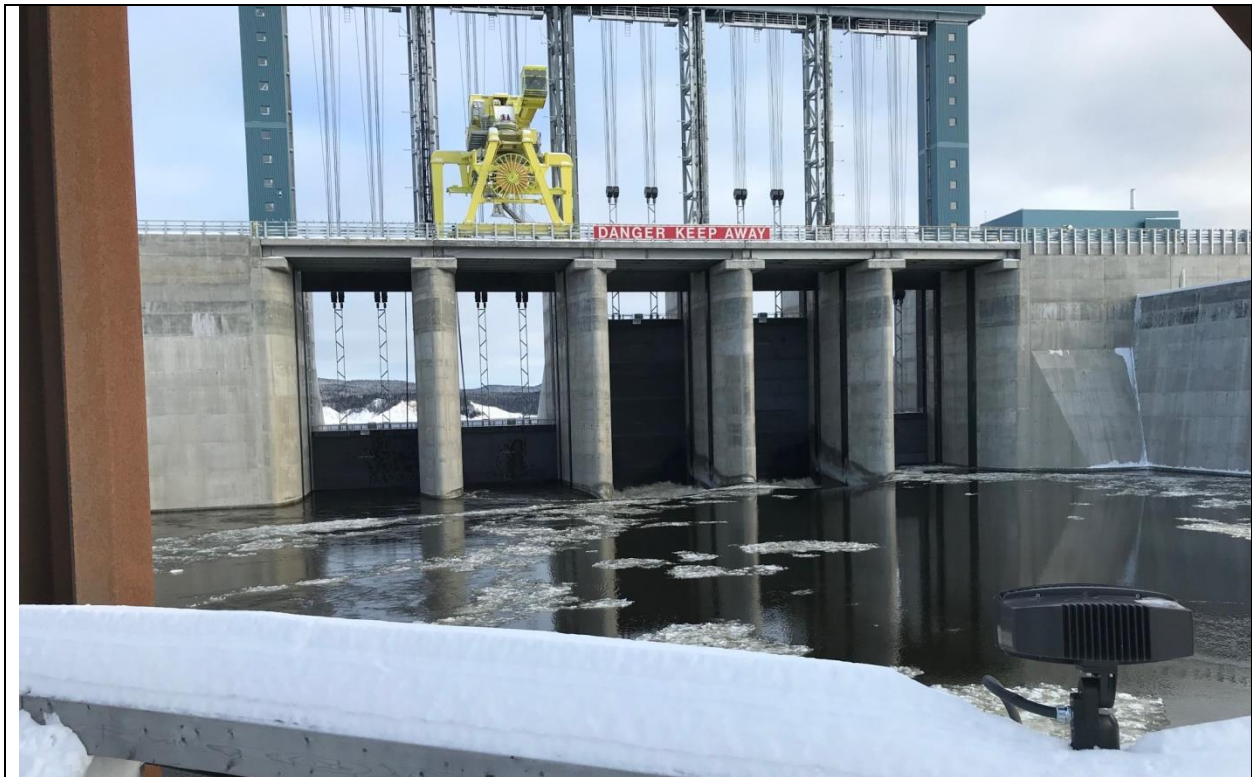
Photo C.2: Upstream side of spillway with two gates open.
