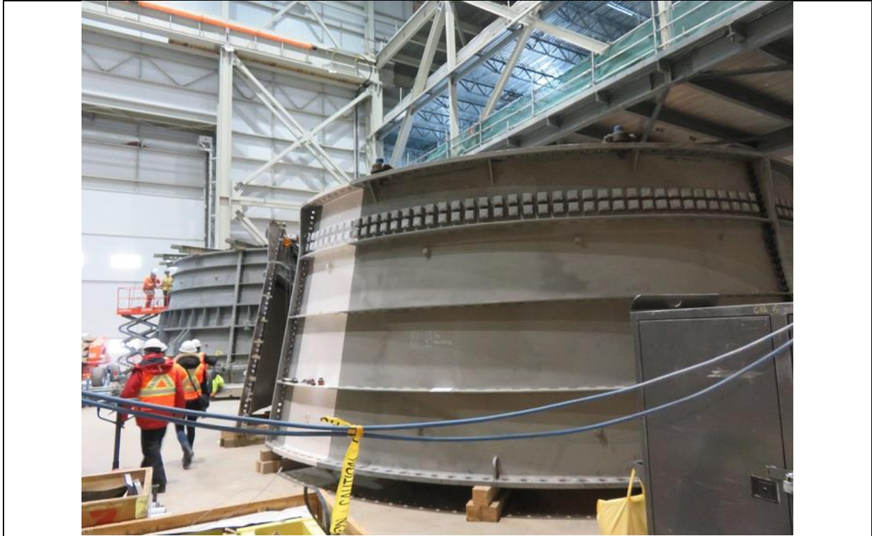
Photo B.7: Draft tube liner.
