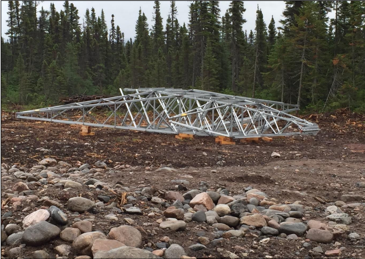
Photo 3.1 HVdc structure assembly (July 8, 2015).
