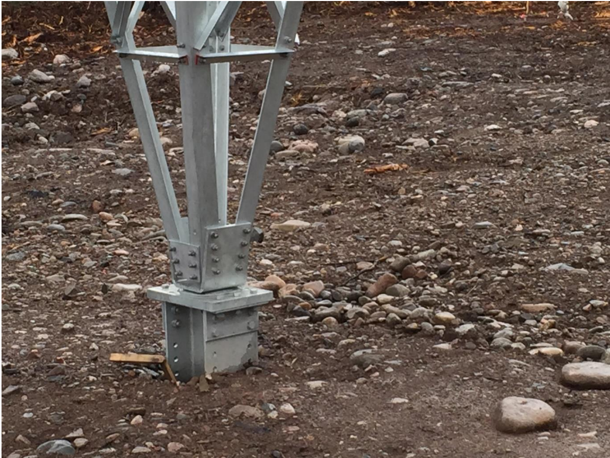
Photo 3.2 HVdc transmission line foundation installation ( July 8, 2015 ).
