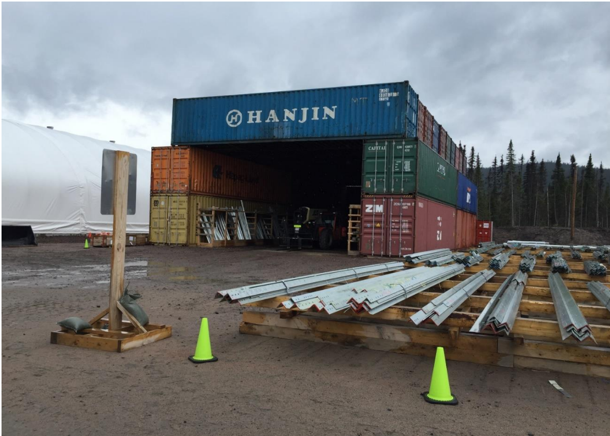
Photo 4.8 Transmission lines Marshaling Yard (July 8, 2015).
