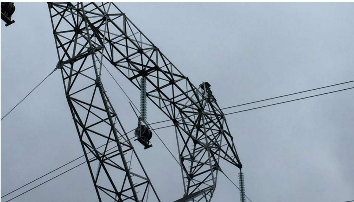
Photo 4.7 HVac transmission line – Stringing (July 8, 2015).
