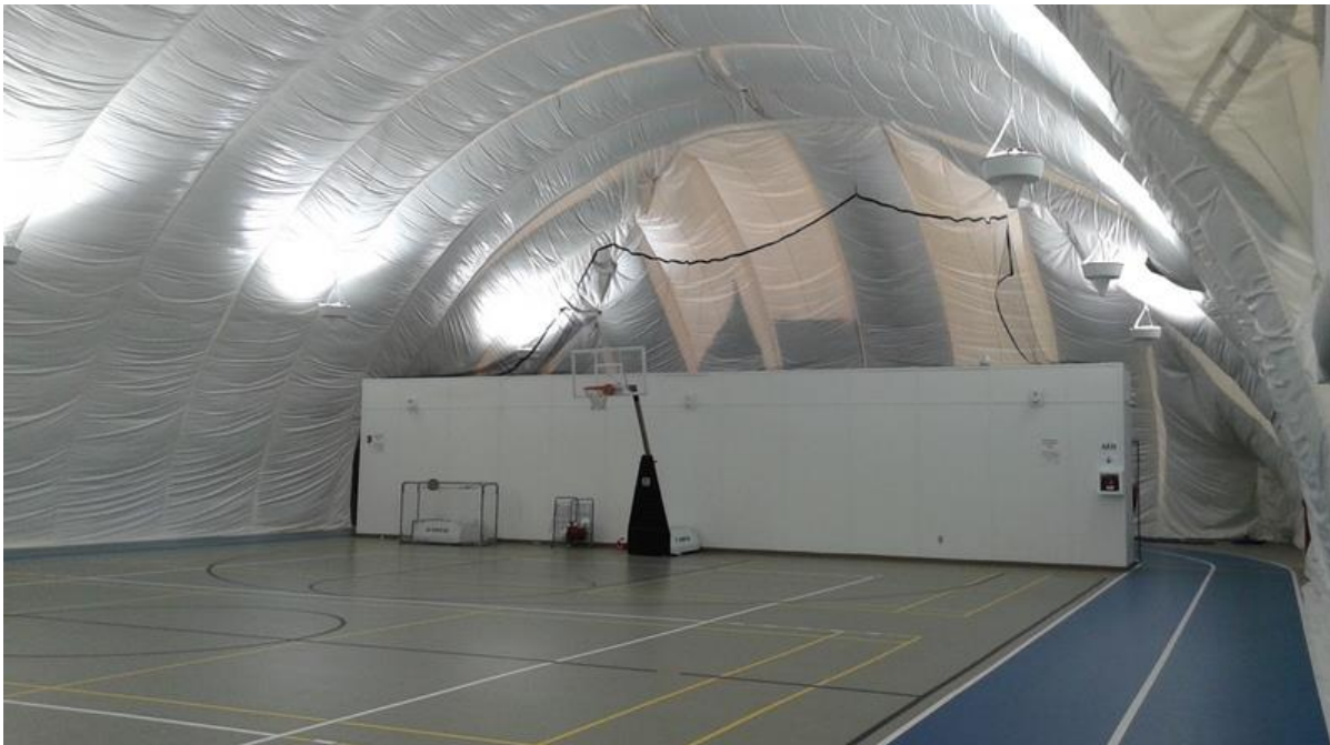
Photo 5 Fully operational gym in the project camp complex (July 7, 2015).
