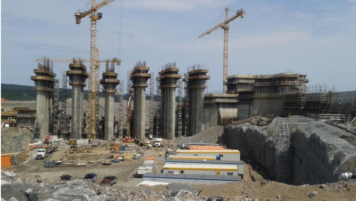
Photo 6.1 Upstream view of Spillway piers, Transition Dams and Separation Wall (July 7, 2015).
