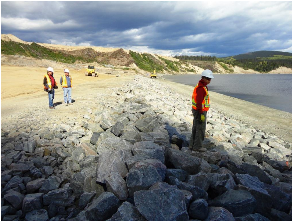
Photo 3.24: Downstream slope, toe rip rap
