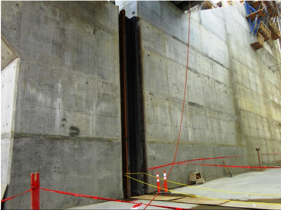
Photo 4.3: Spillway, Bay No. 2. Guide for downstream stop logs.
