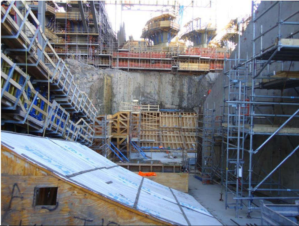
Photo 4.11: Powerhouse, Unit 2. Formworks are visible.
