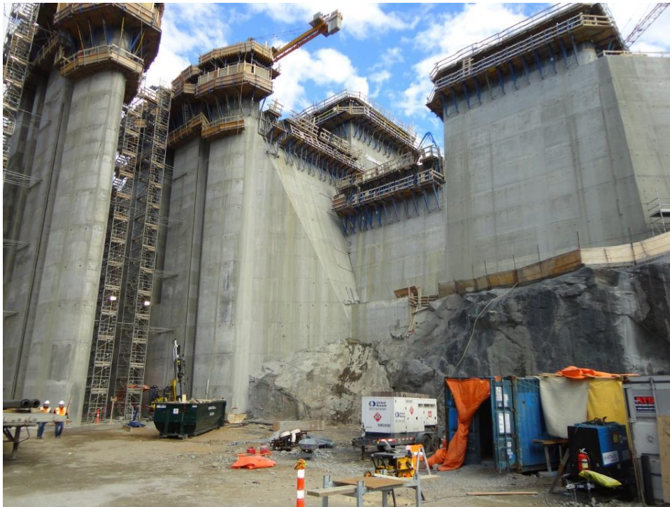
Photo 4.5: Spillway, view of upstream right corner. The left end of the concrete transition dam is visible in the upper central area of the photograph.
