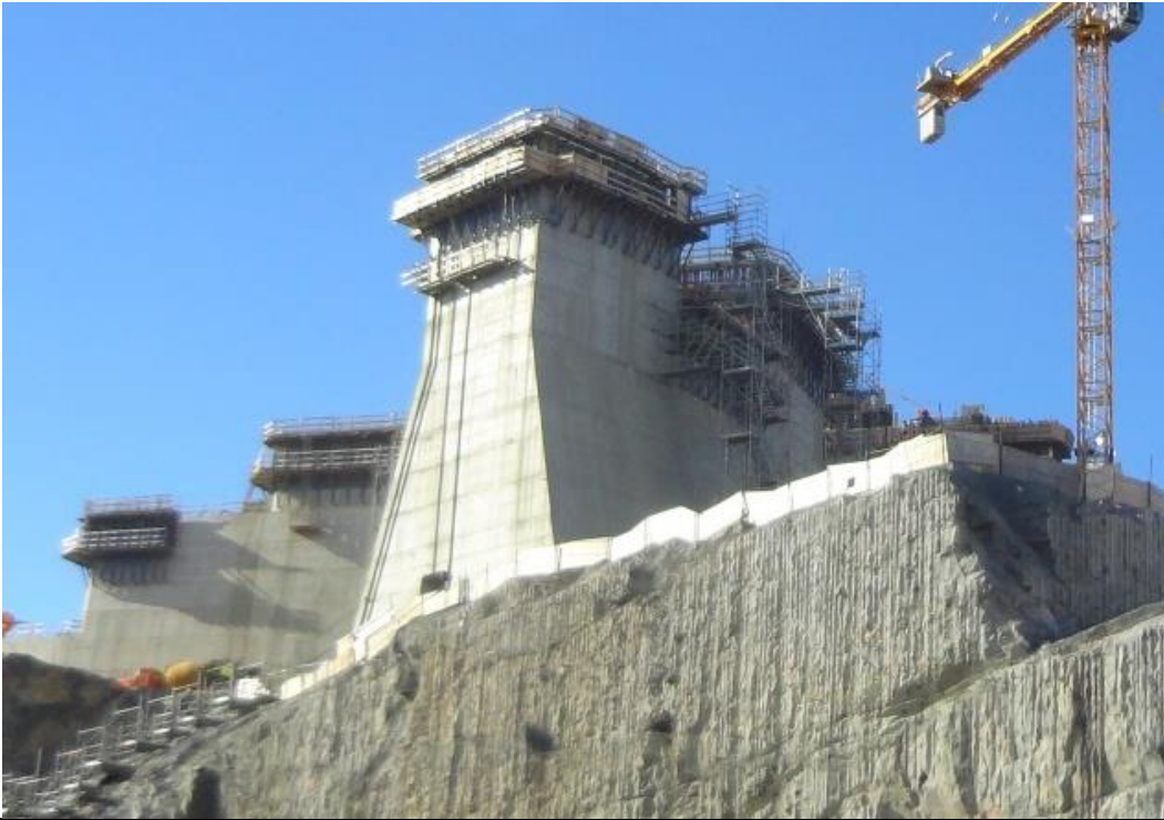
Photo 4.9: Concrete transition dam between the powerhouse and the spillway
