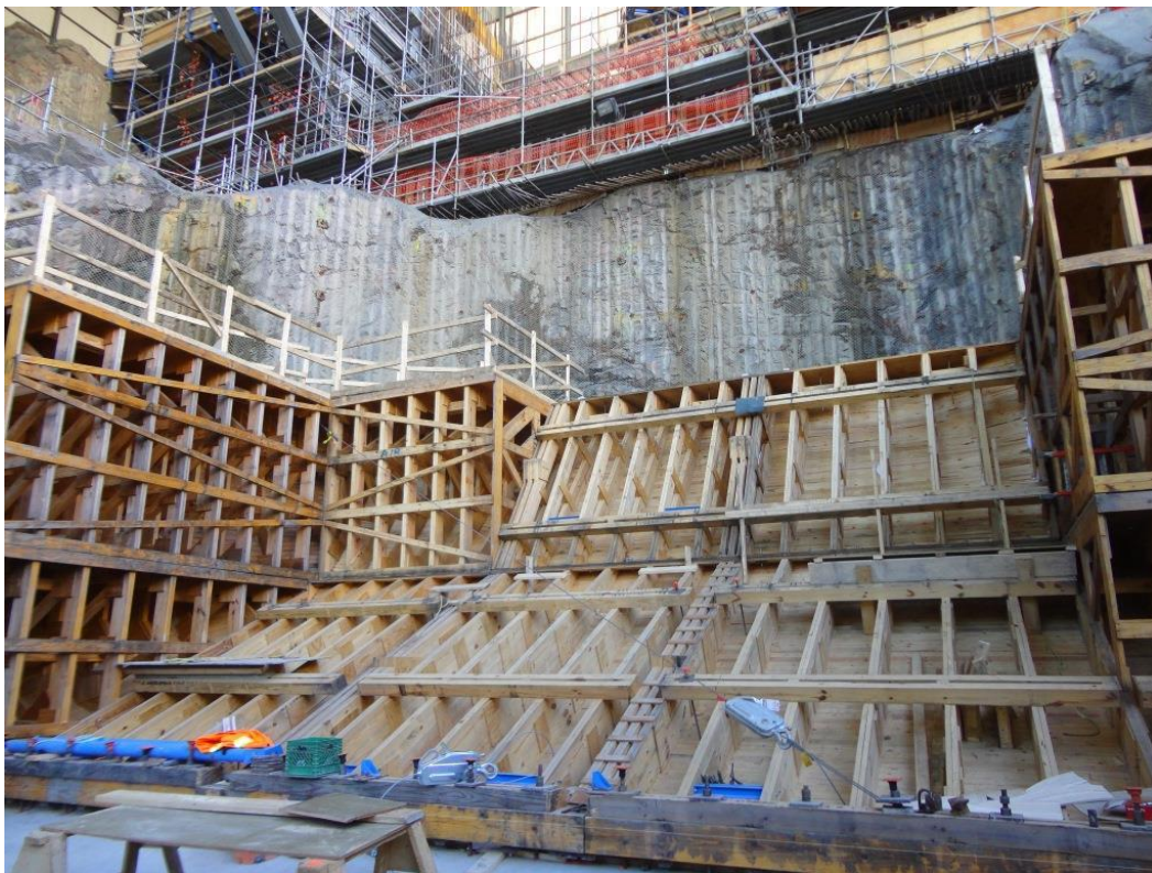
Photo 4.12: Powerhouse. Formwork in Unit 2.
