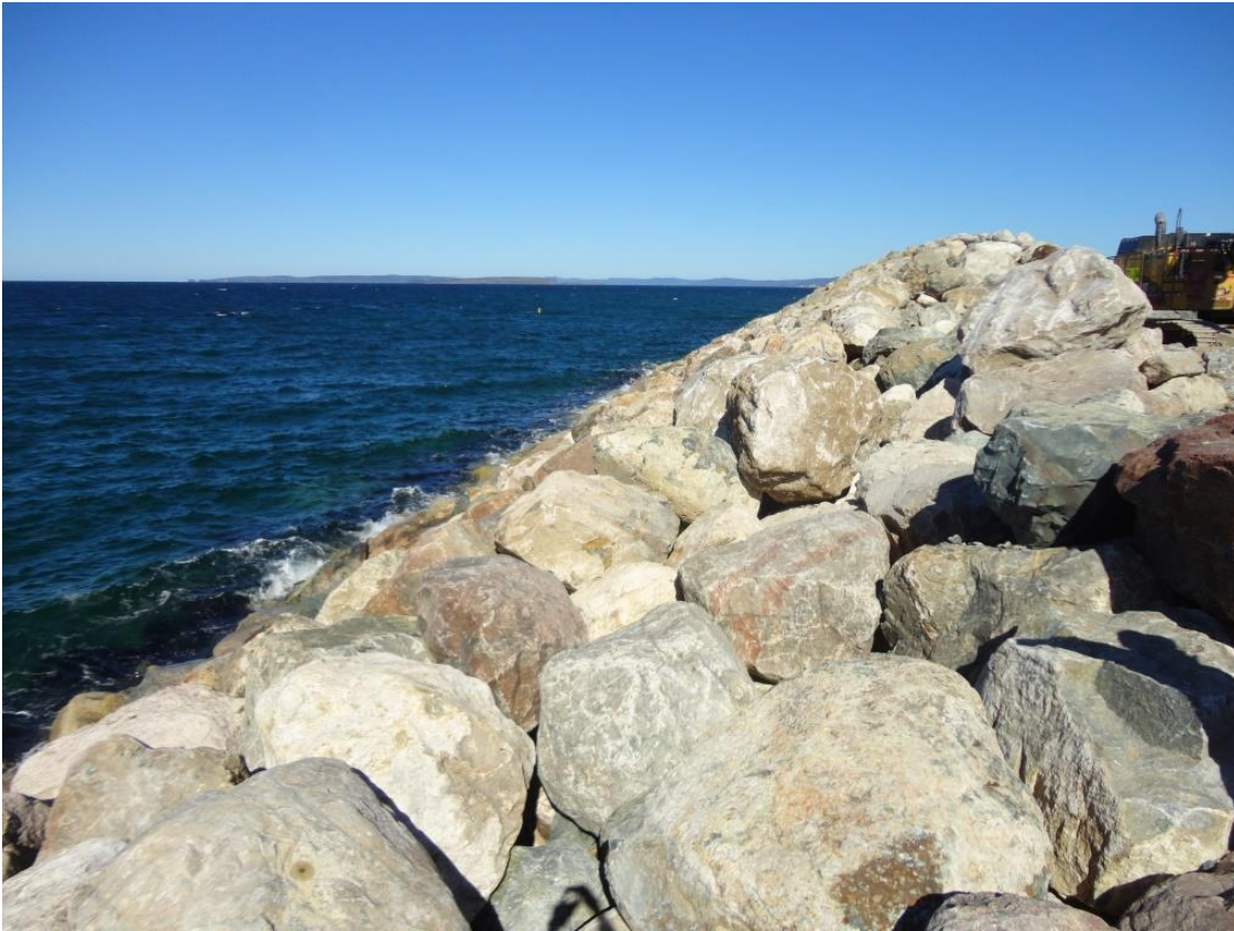
Photo 1.7: Armour stone blanket on the outer slope.
