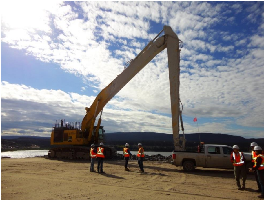
Photo 3.16: Upstream slope- Long stick backhoe excavator used to excavate most of the upstream slope cut-off wall to depths of about 15m
