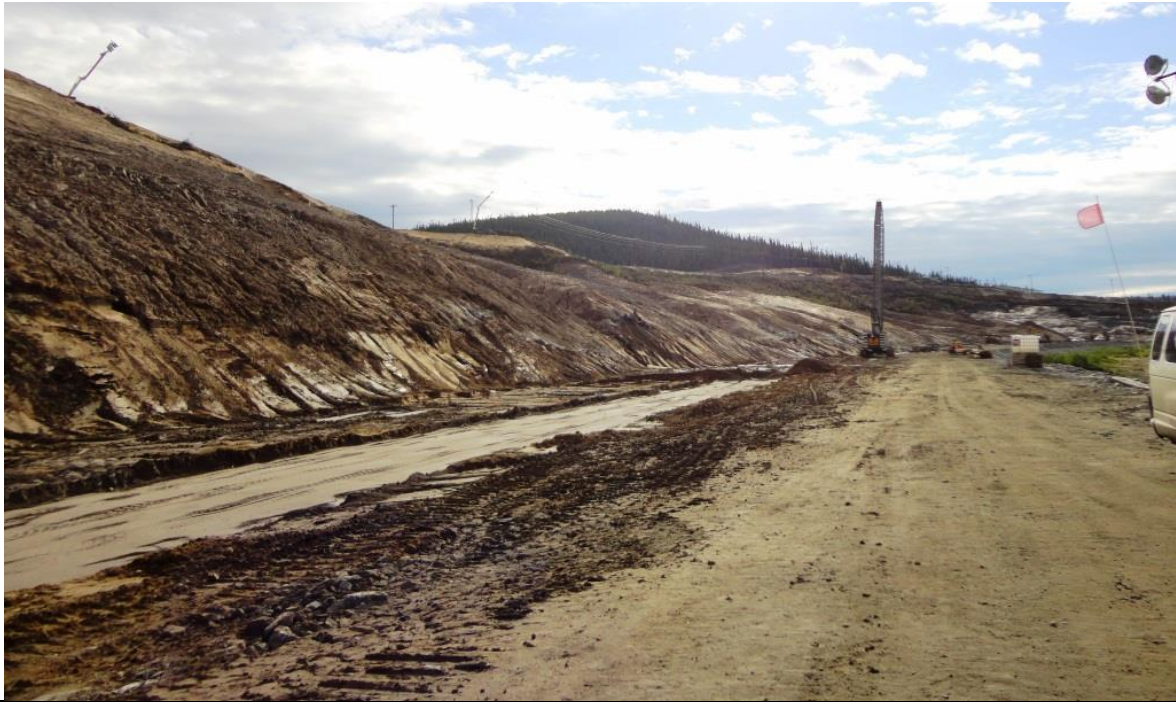
Photo 3.7: Upstream slope - Upstream toe at el 20m; top of cutoff wall, covered by a compacted till is visible running from the lower left corner of the photograph. View is looking south.
