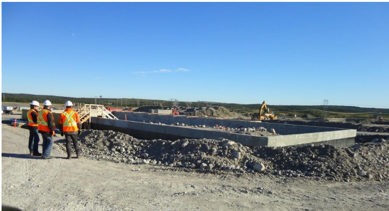
Photo 2.4: AC Substation Control Building foundation
