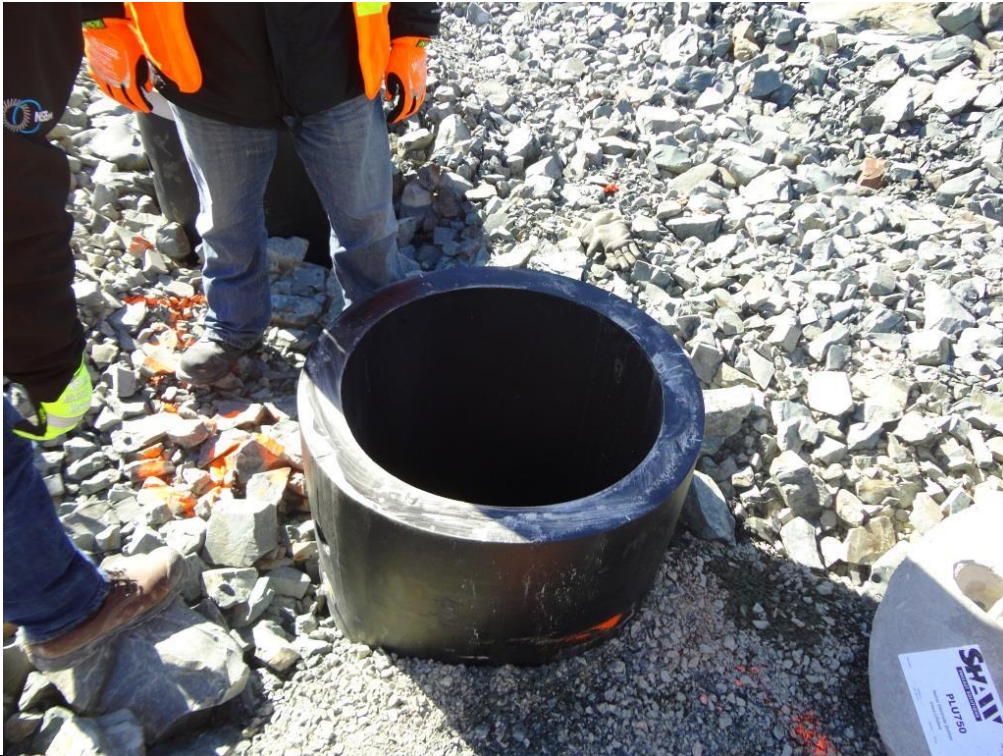
Photo 1.5: Electrode well casing installation
