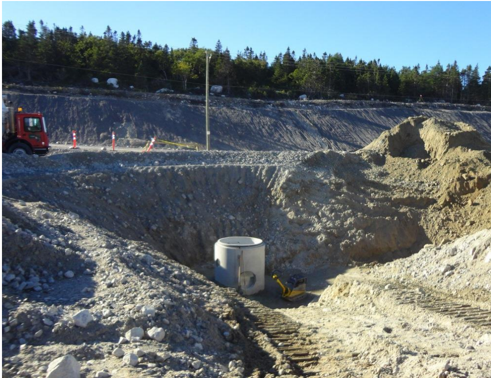
Photo 2.7: Manhole for the oil water separator for the synchronous condenser facility at the west side of the site.
