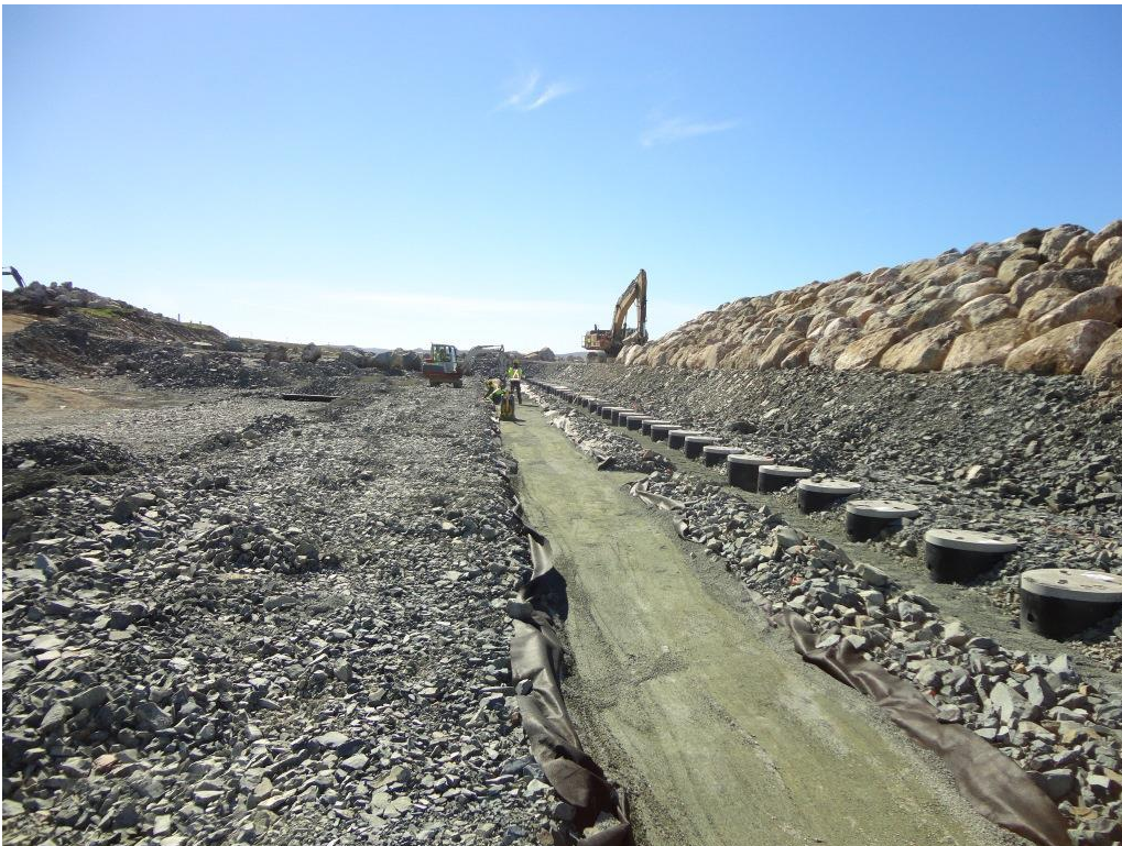
Photo 1.4: Looking west along the line of electrode wells and the conductor bedding trench.
