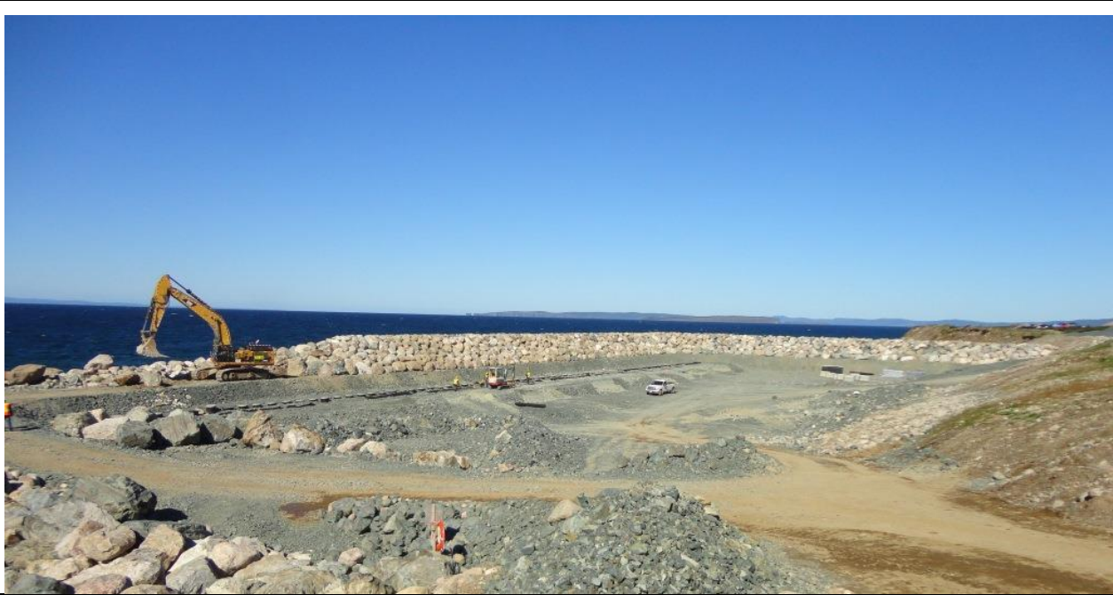
Photo 1.1: Dowden's Point dyke. Note the line of electrode wells at the base of the dyke.
