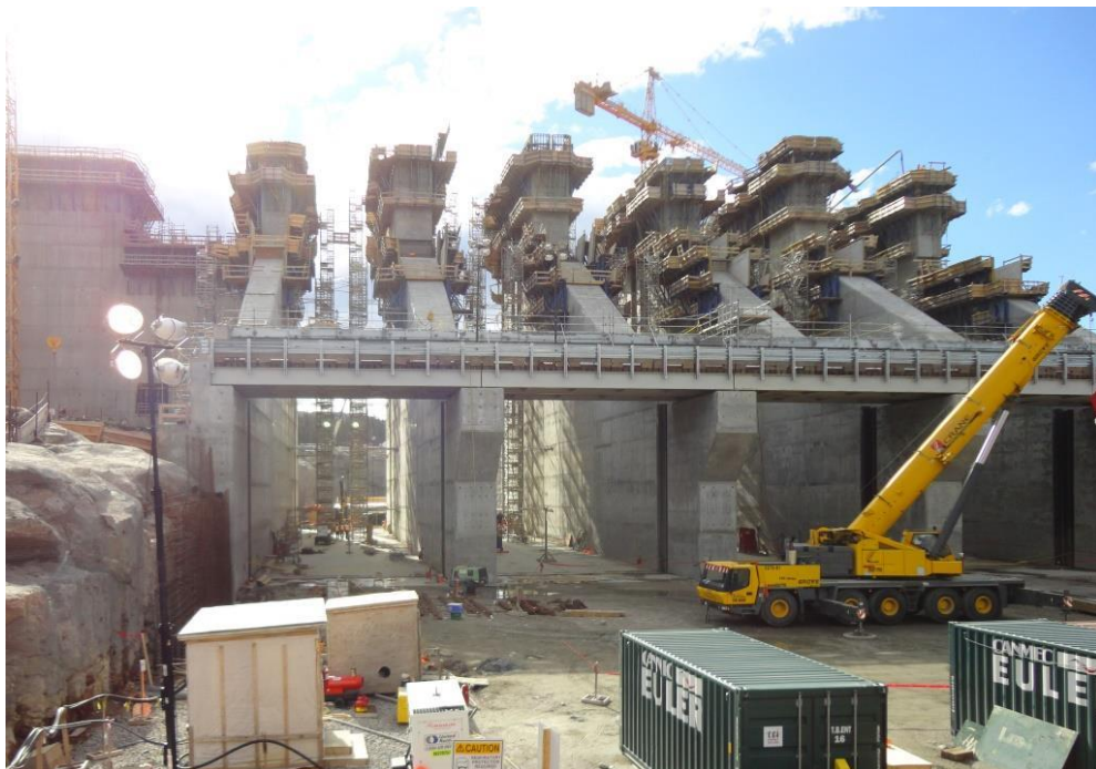
Photo 4.2: Spillway, downstream side as viewed looking upstream.
