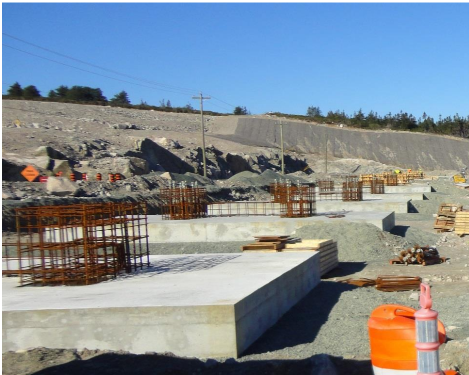
Photo 2.8: Foundation pads of the gantries in the AC substation
