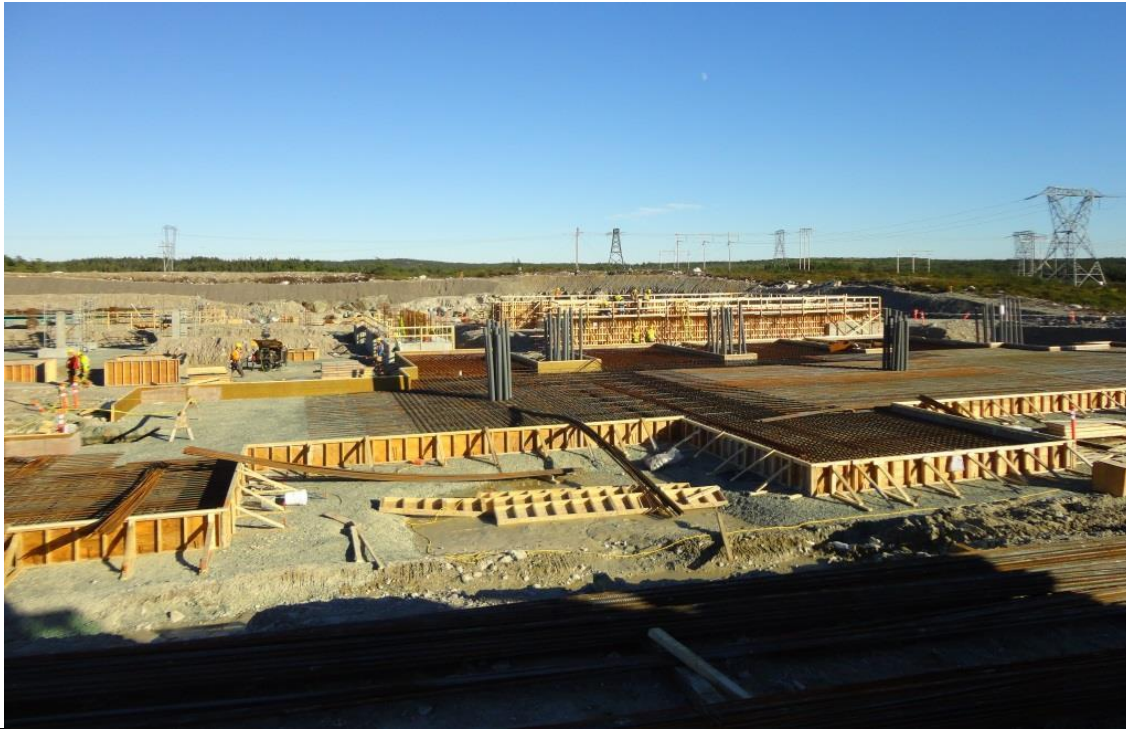
Photo 2.9: DC transformer foundation pads, southern area
