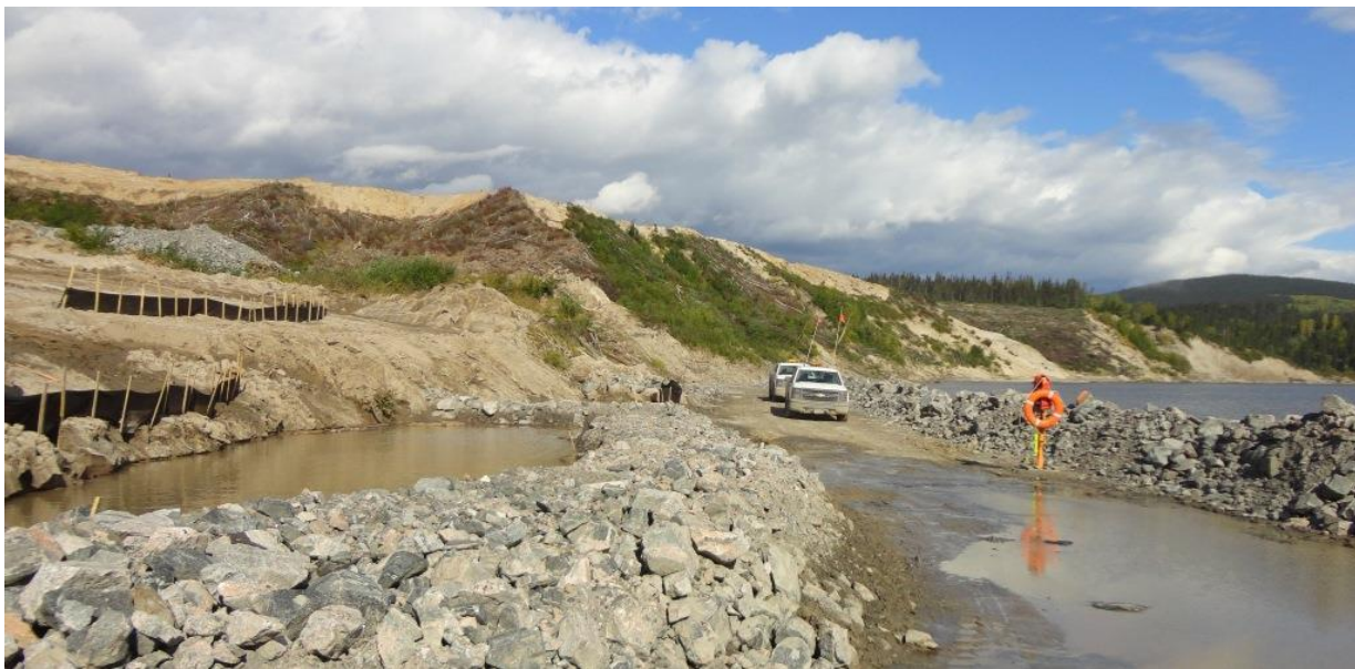
Photo 3.20: Downstream slope; water collection and silt fences at toe of slope. Some slope trimming has been done in the lower slope. Some debris from the 1978 slide are visible in the background (upslope from the white pick-up trucks).
