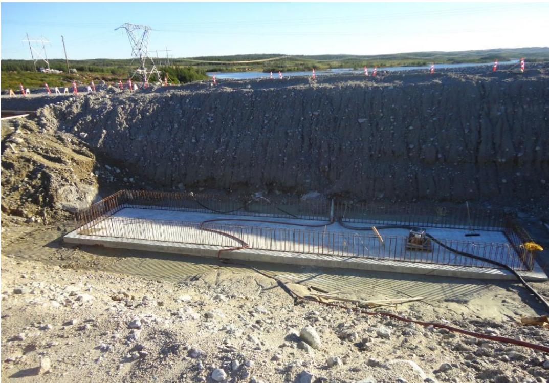
Photo 2.6: Base slab for oil/water separator
