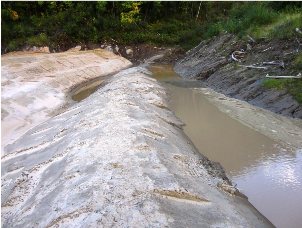
Photo 3.21: Downstream slope. Water collection ditch at the toe of the slope.
