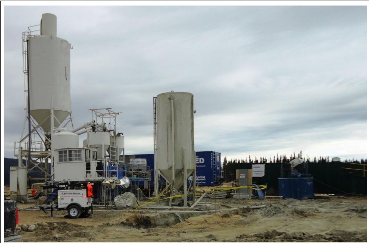
Photo 3.18: Plant for mixing the cement bentonite slurry of the cut-off wall.
