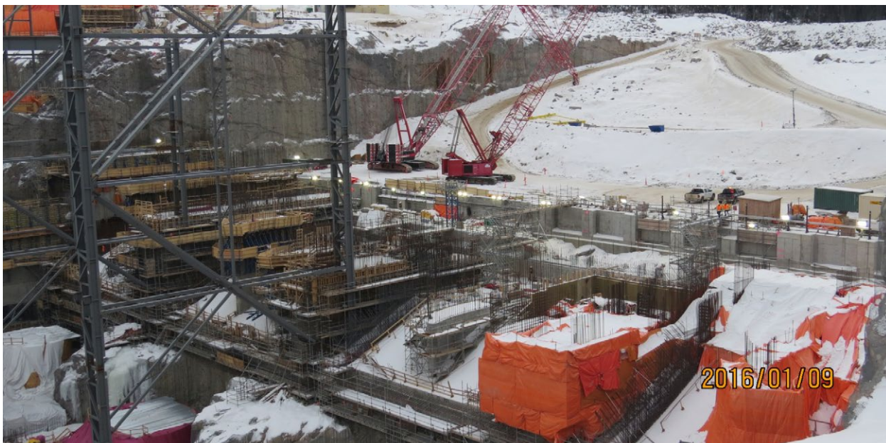
Progress on the Powerhouse at the Muskrat Falls Site – January 2016
