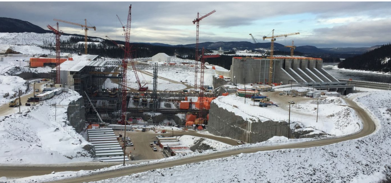
Muskrat Falls Site – Progress on Spillway and Powerhouse – December 2015
