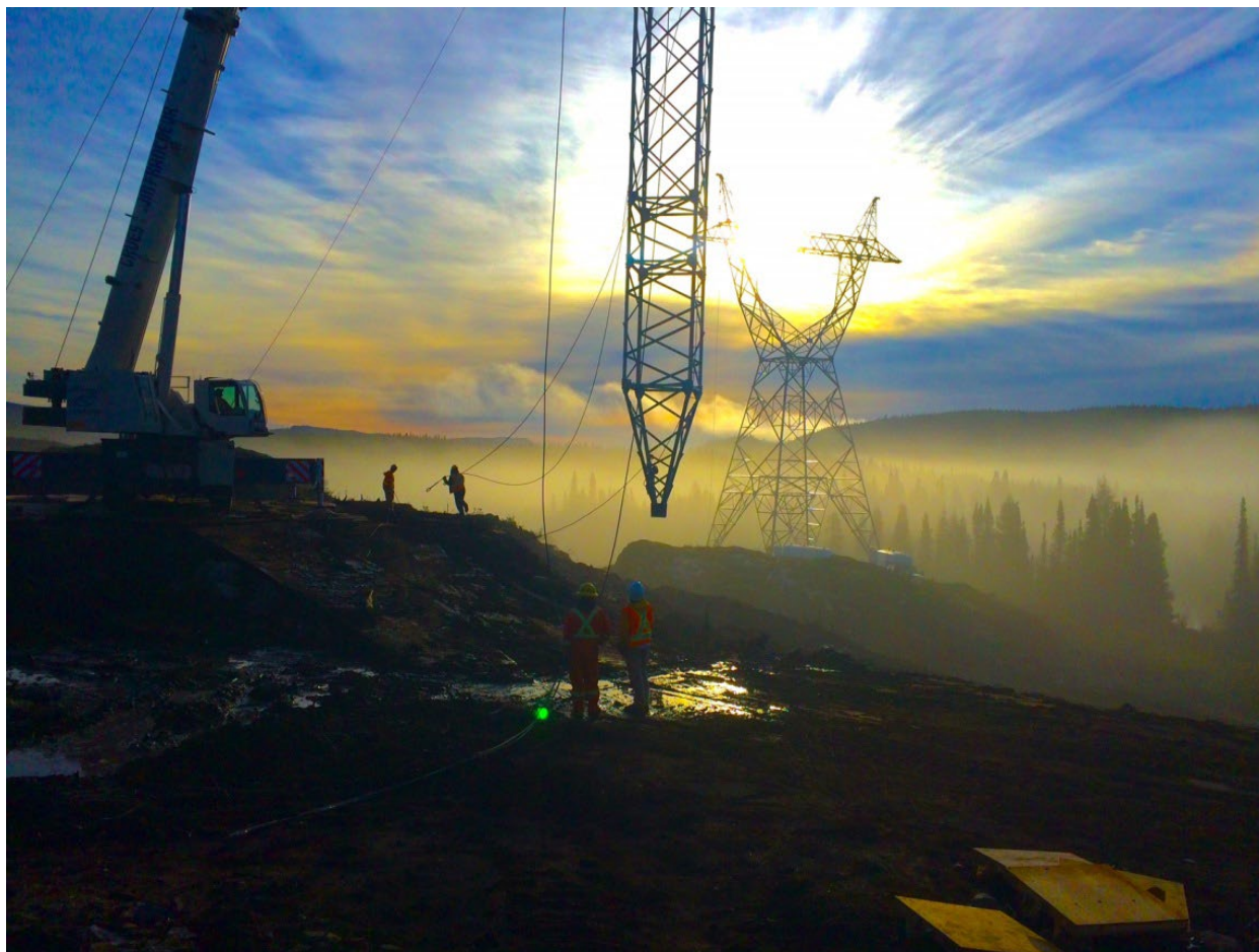
Progress on the HVdc Transmission Line (Labrador-Island Transmission Link) – December 2015
