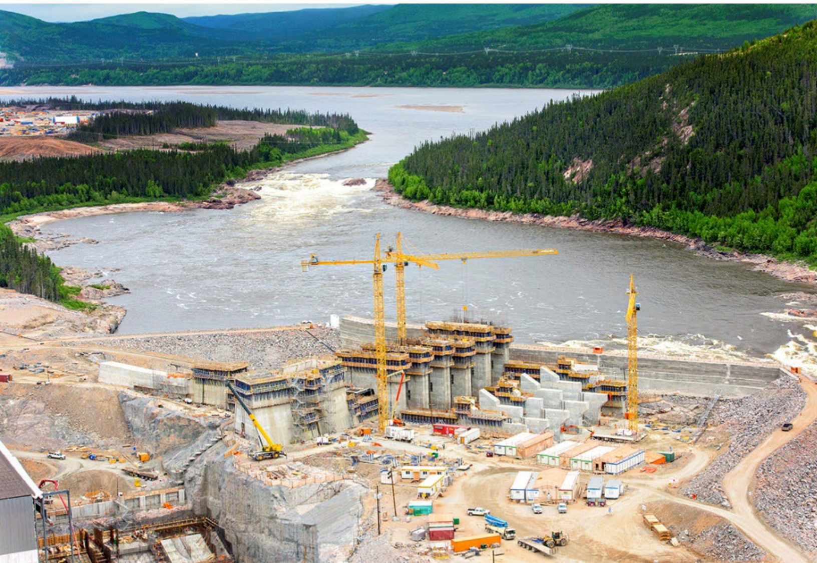
Muskrat Falls Site – Progress on Spillway and Powerhouse – August 2015
